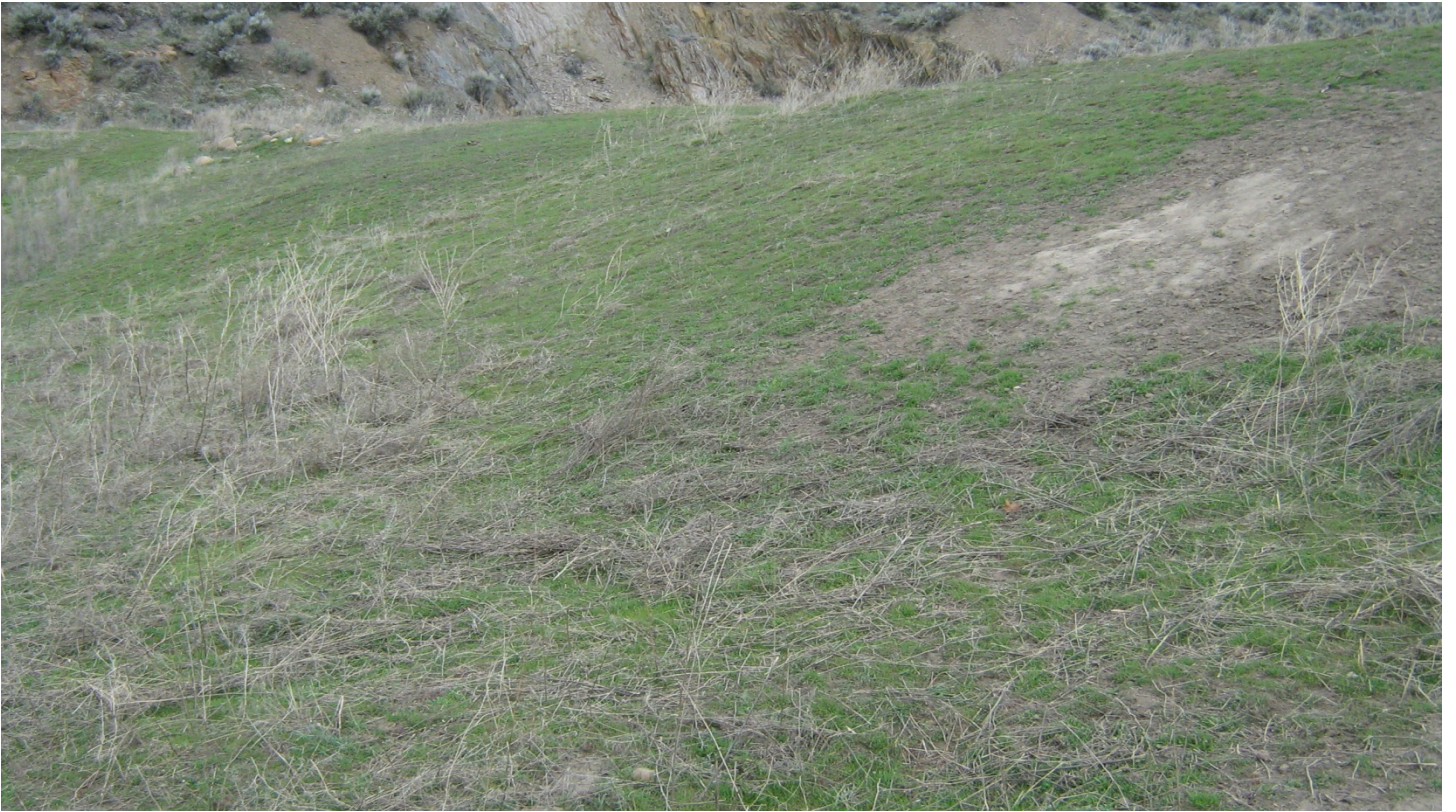
SMM Tailings Cap with Exposed Soil from the Southeast
