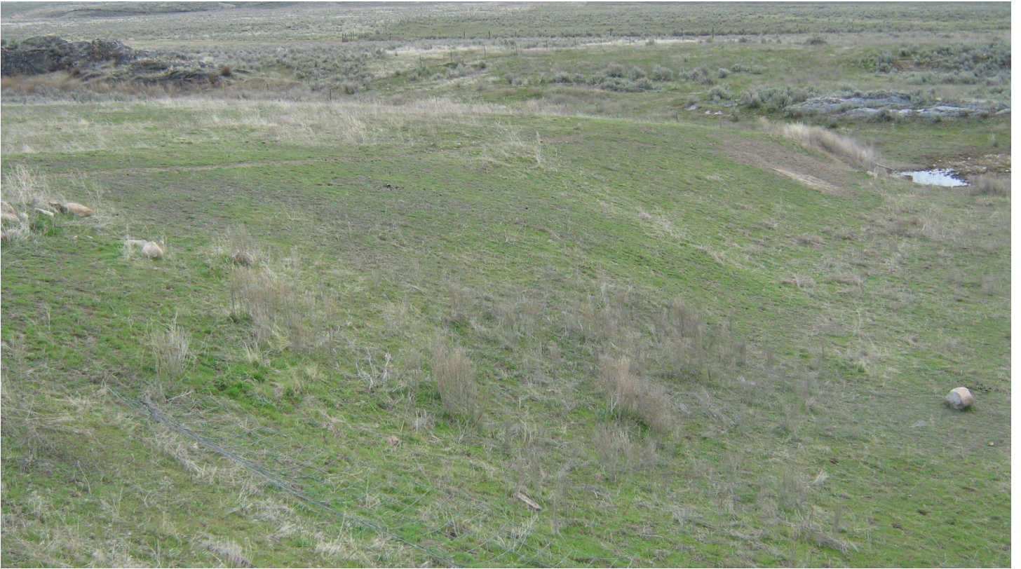
SMM Tailings Cap from the Southwest
