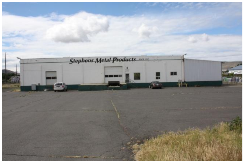
Figure 3: FMC's former warehouse, occupied until recently by Stephens Metal Products
