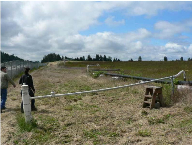
Landfill cover with gas extraction system.
