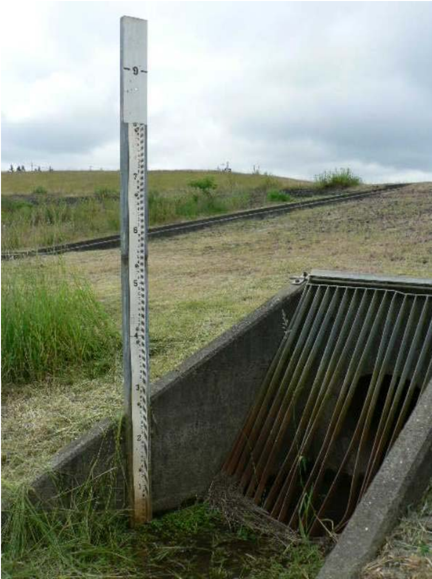
Retention pond drainage.
