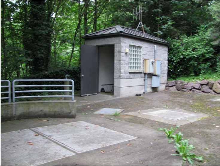
Linda Heights Park storm water diversion mechanical room.
