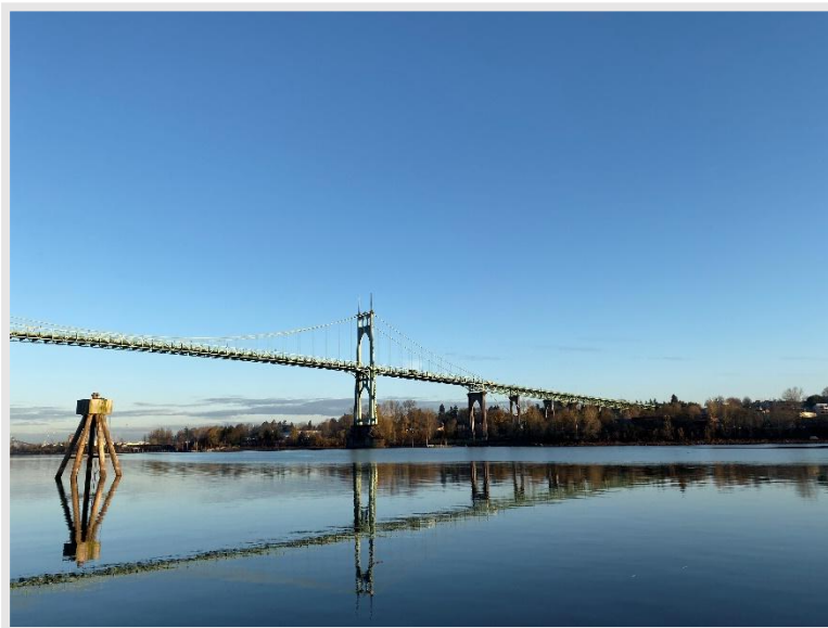
St. Johns Bridge
