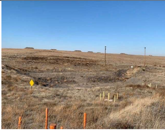
Lagoon area with Lagoon Infiltration Field in the background
