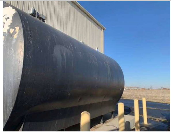
Exterior tank (View 3)
