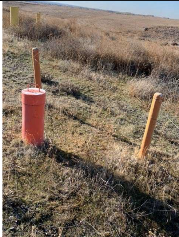
Well near washout lagoons with only two bollards
