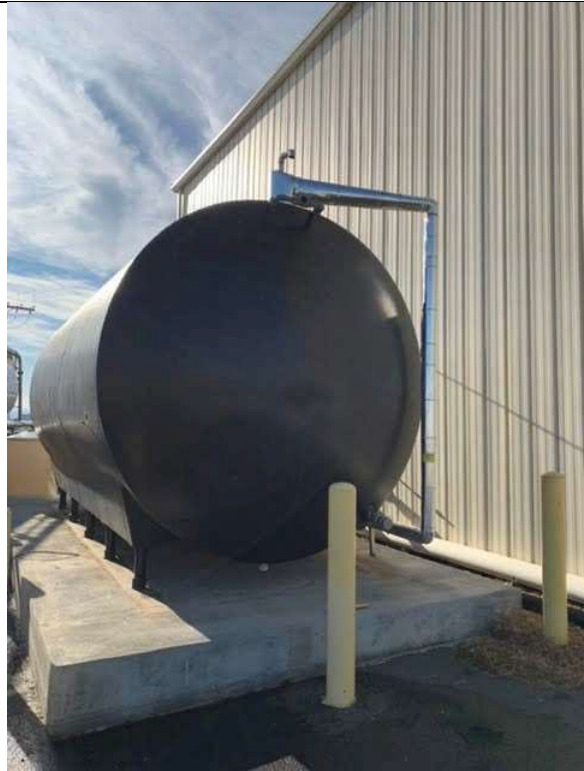
Exterior tank (View 1)
