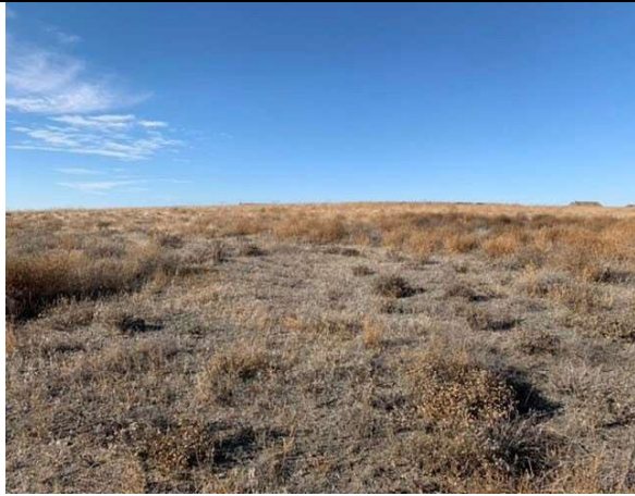
Landfill Cap (Southern side)
