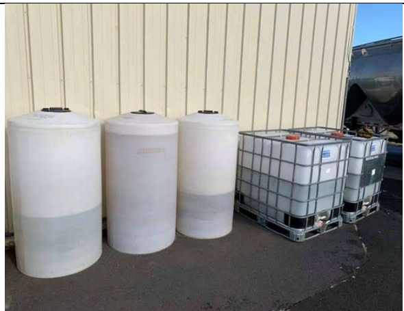
Storage tanks in front of the GETS building
