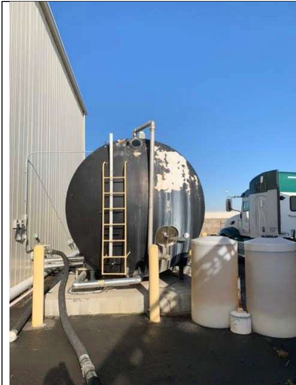
Exterior tank (View 2)
