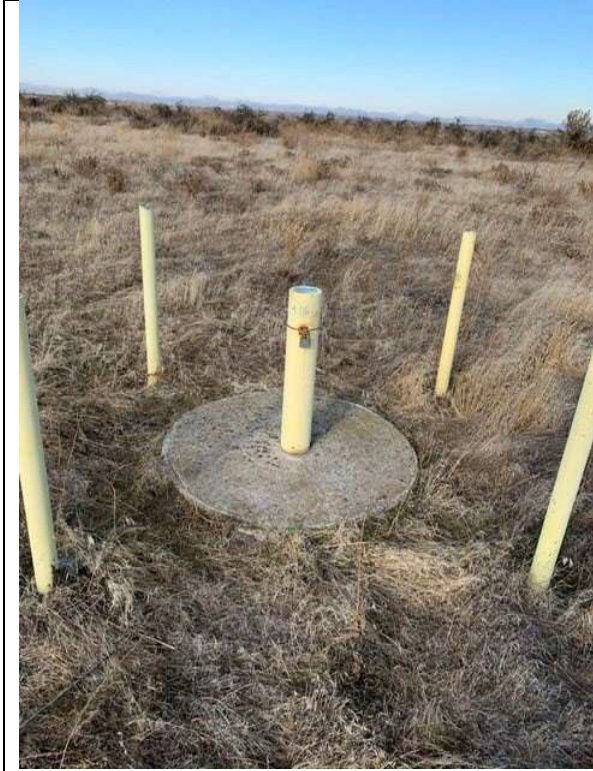
Typical well condition on site (pictured: 4-116)
