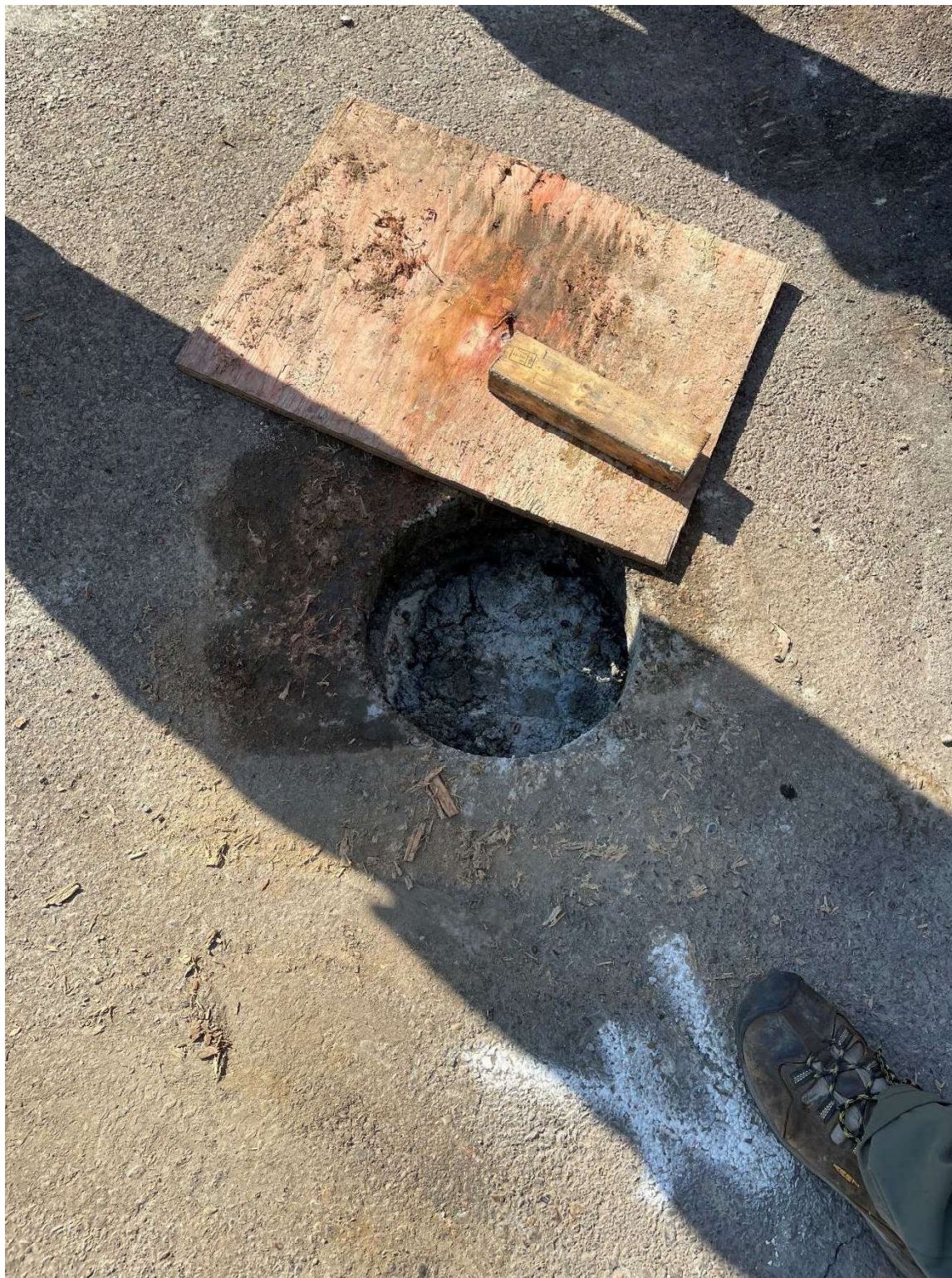
Photo 4 – Example of Abandoned Temporary Emulsified Oil/ZVI Substrate and Microbe Injection Point filled with Grout in the Acid Sump Area
