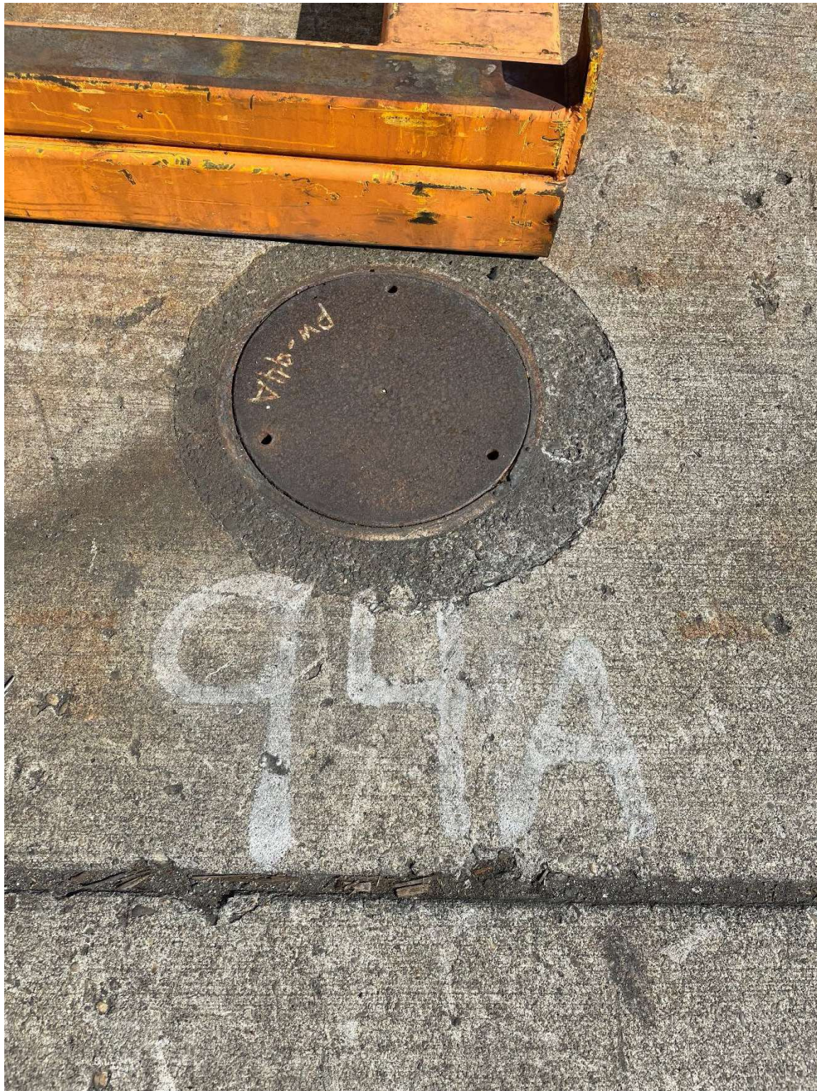
Photo 2 – Example of custom flush steel well cover on Well PW-94A in the Former Crucible Cleaning Area
