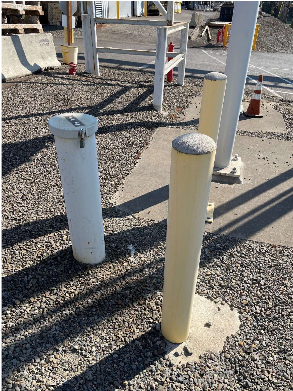
Photo 6 –Above Ground Monitoring Well PW-01A in Ammonia Sulfite Storage Area
