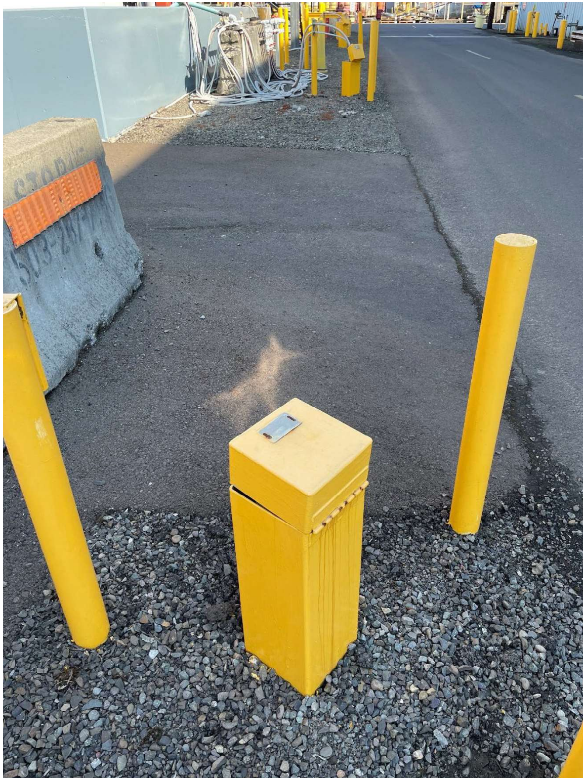
Photo 7 – Example of Ammonia Sulfite Storage Area Temporary Extraction Well
