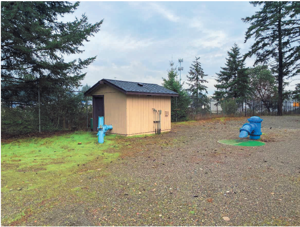
H1 supply well pump house
