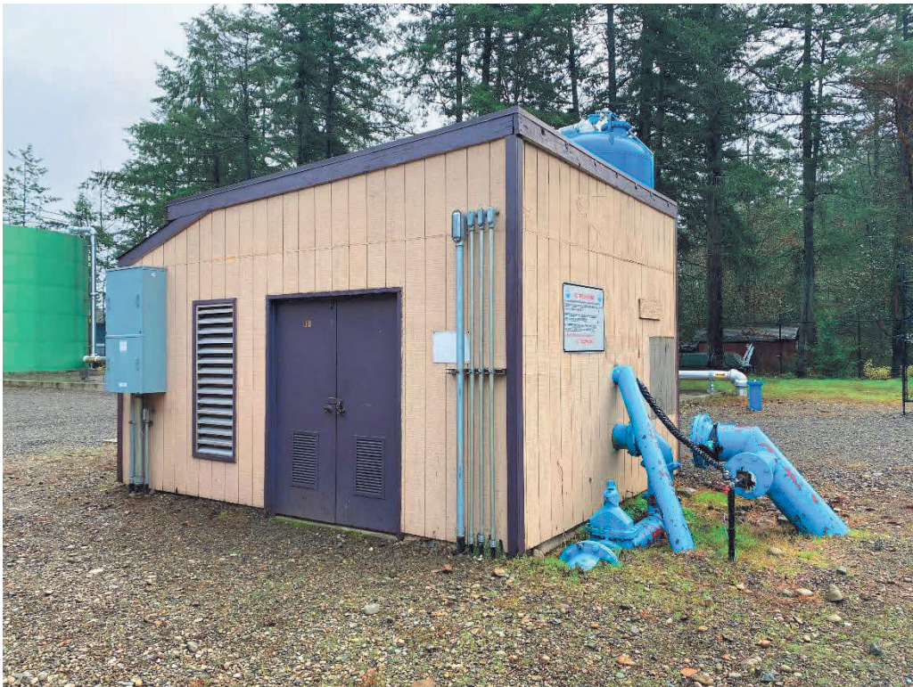
H2 supply well pump house
