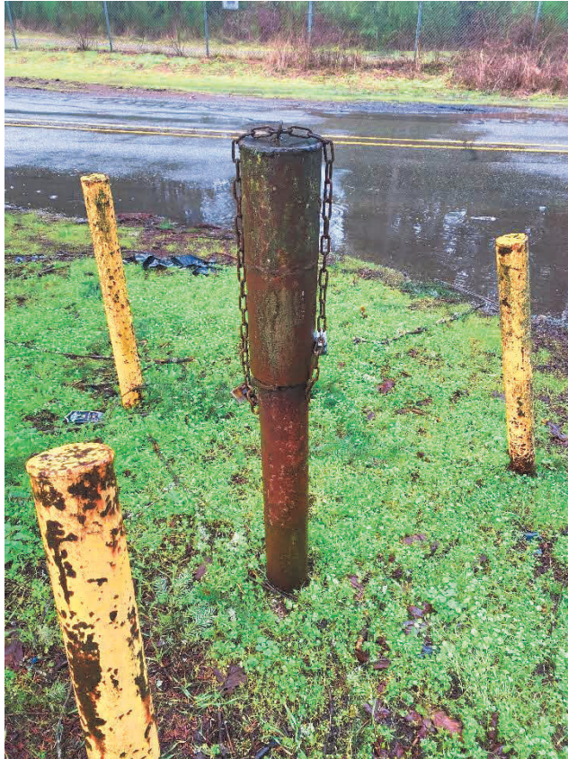
MW-33 along McChord Drive
