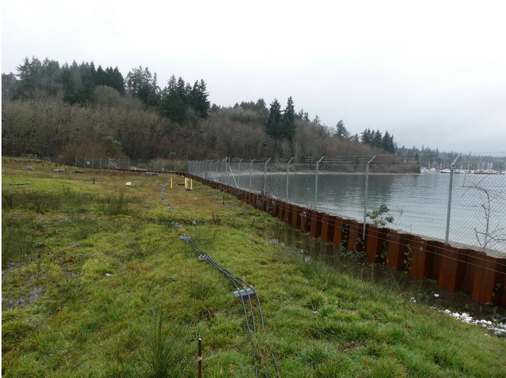
Interior sheet pile wall with West Beach visible in background
