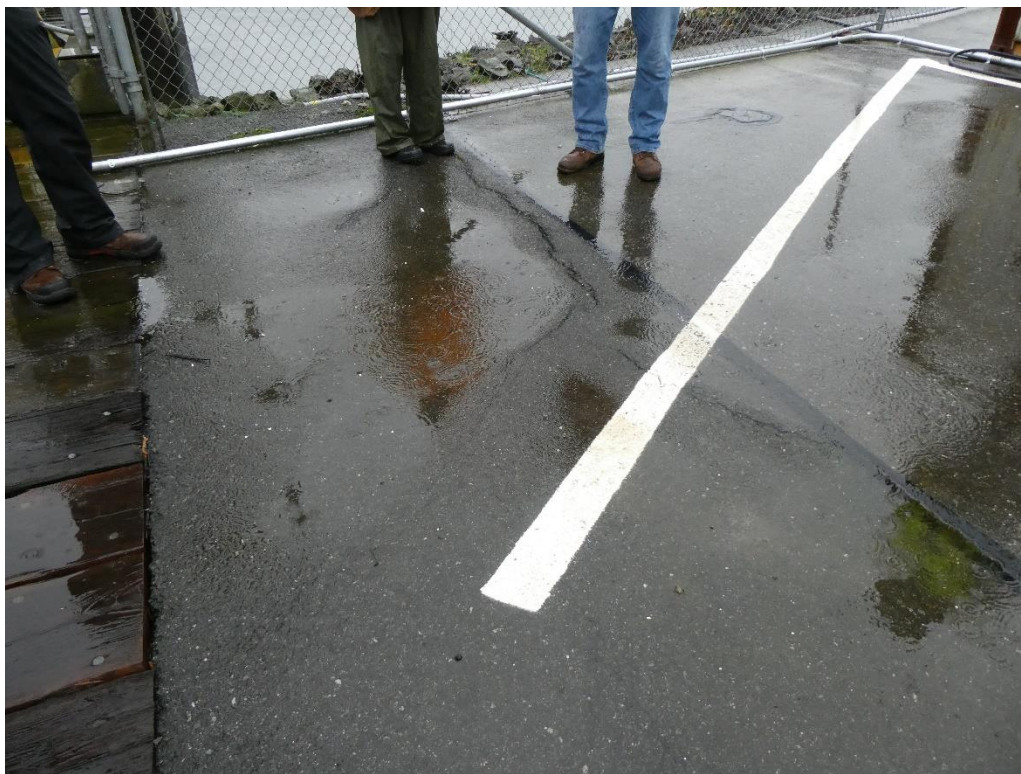
Asphalt crack repair
