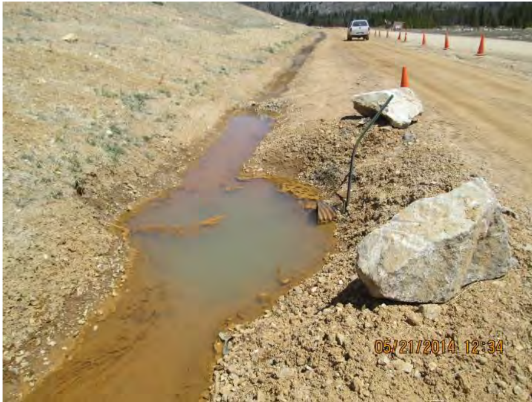
Figure 9E. Photo of the Heap leach seep (YP-T-23A) from the Surface Water Quality Baseline Study, Appendix G, May 2014 Site Photos, page 29. Photo caption reads, “YP-T-23A, Heap leach seep. Looking east and downstream. A portion of the flow is entering a rehabilitated culvert, which daylight on the other side of airstrip. May 2014.”
