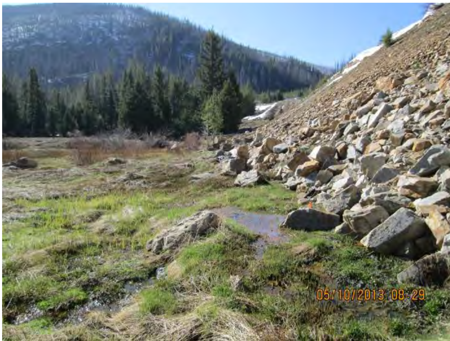
Figure 4D. Photo of the Middle Keyway Dam seep (YP-S-7) from the Surface Water Quality Baseline Study, Appendix G, May 2013 Site Photos, page 15. Photo caption reads, "YP-S-7, Middle Keyway Dam seep. Looking south and across seep source emerging from base of dam, flows downstream to left. May 2013."
