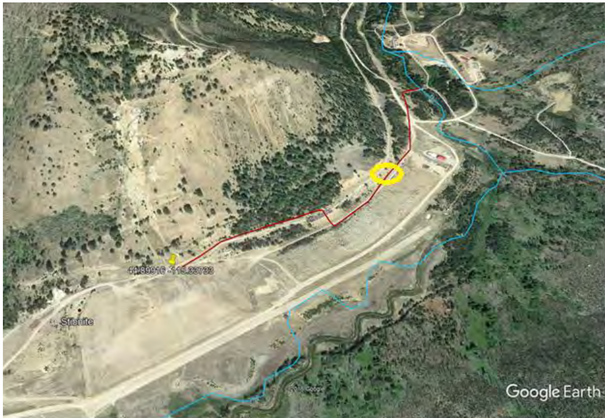
Figure 20A. Aerial view of the flow path that a NPT staff member witnessed during May of 2018. The yellow circle denotes where adit flows went subsurface three weeks later (June, 2018) during a follow-up site visit.
