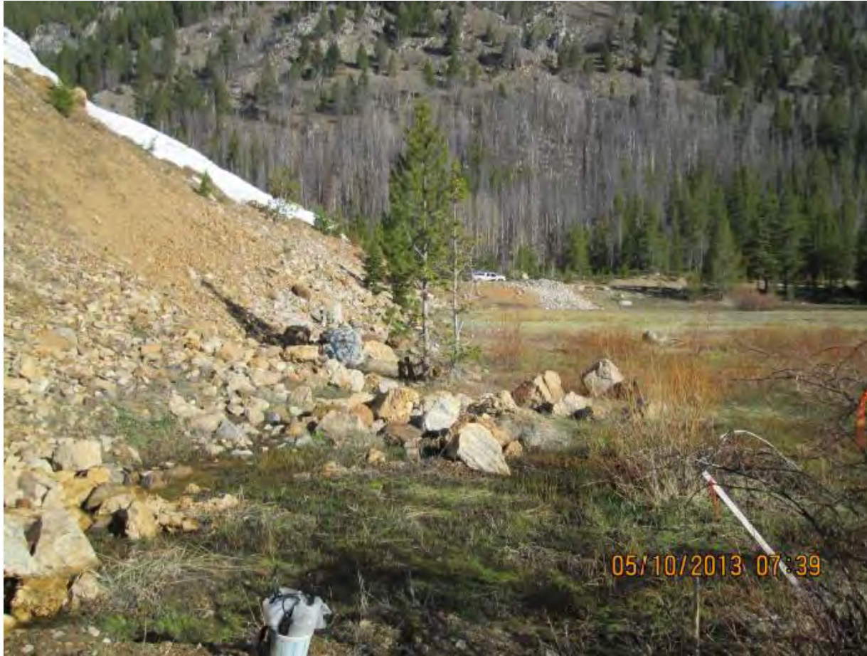
Figure 4A. Photo of the South Keyway Dam seep (YP-S-6) from the Surface Water Quality Baseline Study, Appendix G, May 2013 Site Photos, page 14. Photo caption reads, “YP-S-6, South Keyway Dam seep. Looking north and across seep emerging from base of dam, flows downstream to right. May 2013.”
