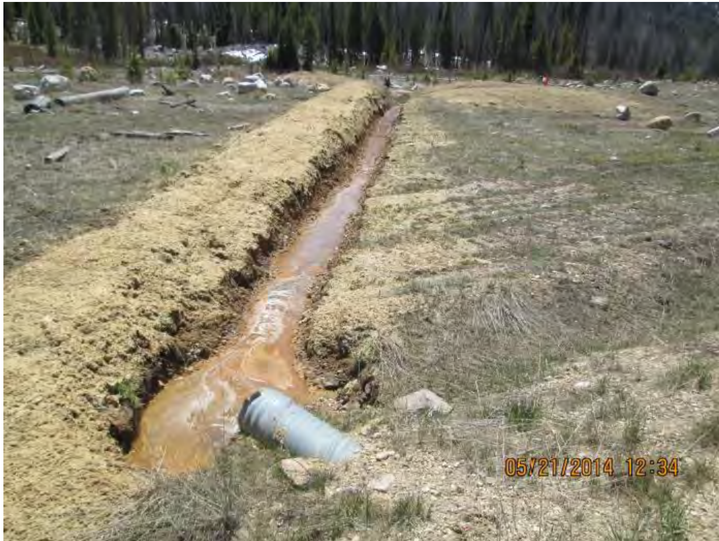
Figure 9F. Photo of the Heap leach seep (YP-T-23A) from the Surface Water Quality Baseline Study, Appendix G, May 2014 Site Photos, page 29. Photo caption reads, "YP-T-23A, Heap leach seep. Looking south and downstream at flow from culvert in previous photo, with trench to convey flow toward sediment basin. May 2014."
