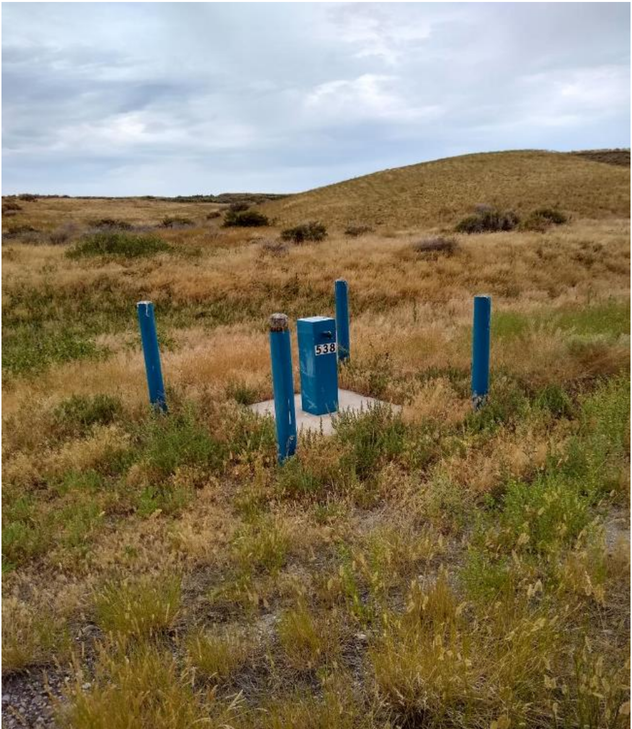
Photograph 32 - IMG_20200722_114247955_HDR: Compliance Area; well 538, locked with bollard protection
