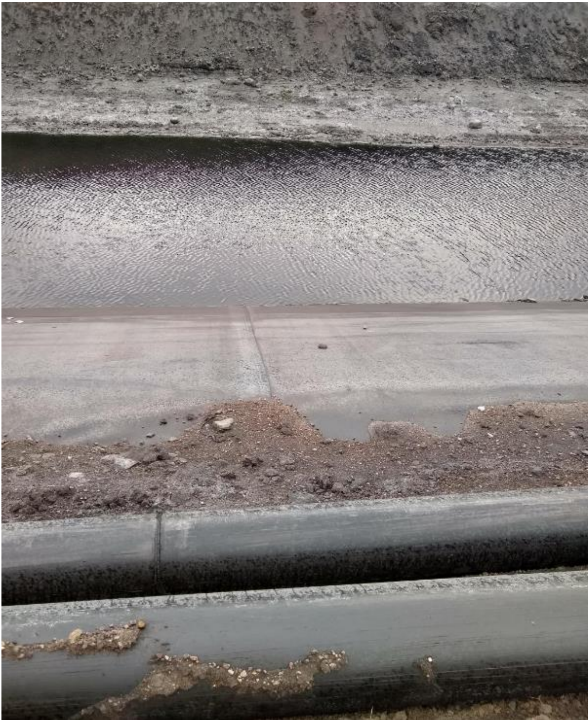
Photograph 24 - IMG_20200722_103706566_HDR: Gypsum Stack; exposed liner in seepage collection ditch [Note: Exposed liner in decant ditches is not in operation.]
