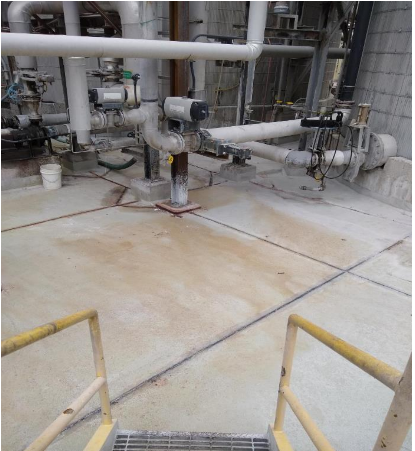
Photograph 2 - IMG_20200722_091551584: Phosphoric acid Plant; phosphoric acid tank sump pad repair, acid brick and mortar replaced by cement and impervious acid/heat resistance coating
