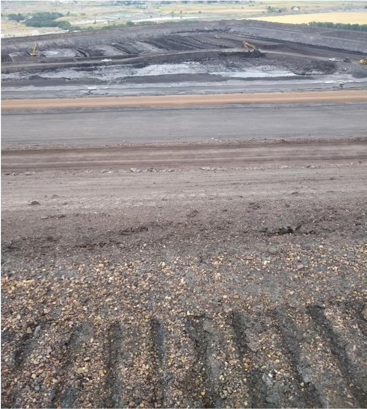
Photograph 23 - IMG_20200722_103352893: Gypsum Stack; middle of picture, road 50' above phase I, phase I will grow to connect with Phase 4
