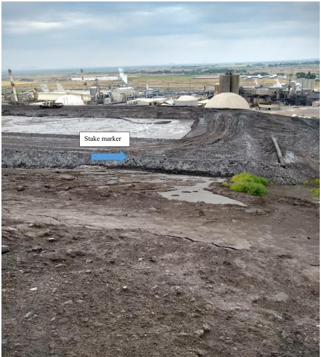
Photograph 31 - IMG_20200722_111719935_HDR: Gypsum Stack; stake with orange tape, such as in foreground indicate no dig area as liner is less than 1 foot below
