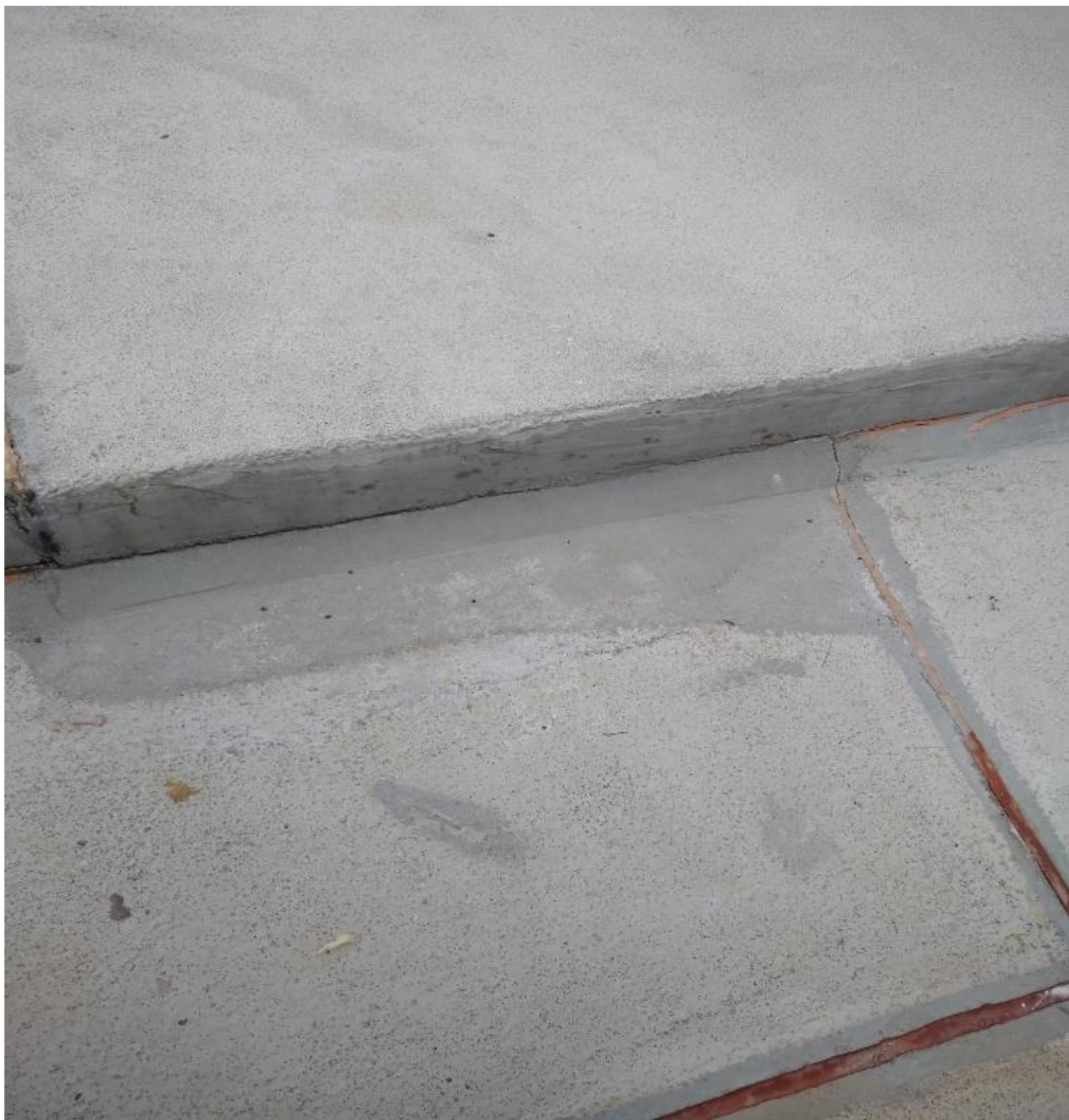
Photograph 3 - IMG_20200722_091607849: Phosphoric acid Plant; acid tank sump pad repair, expansion joints and floor and wall abutments
