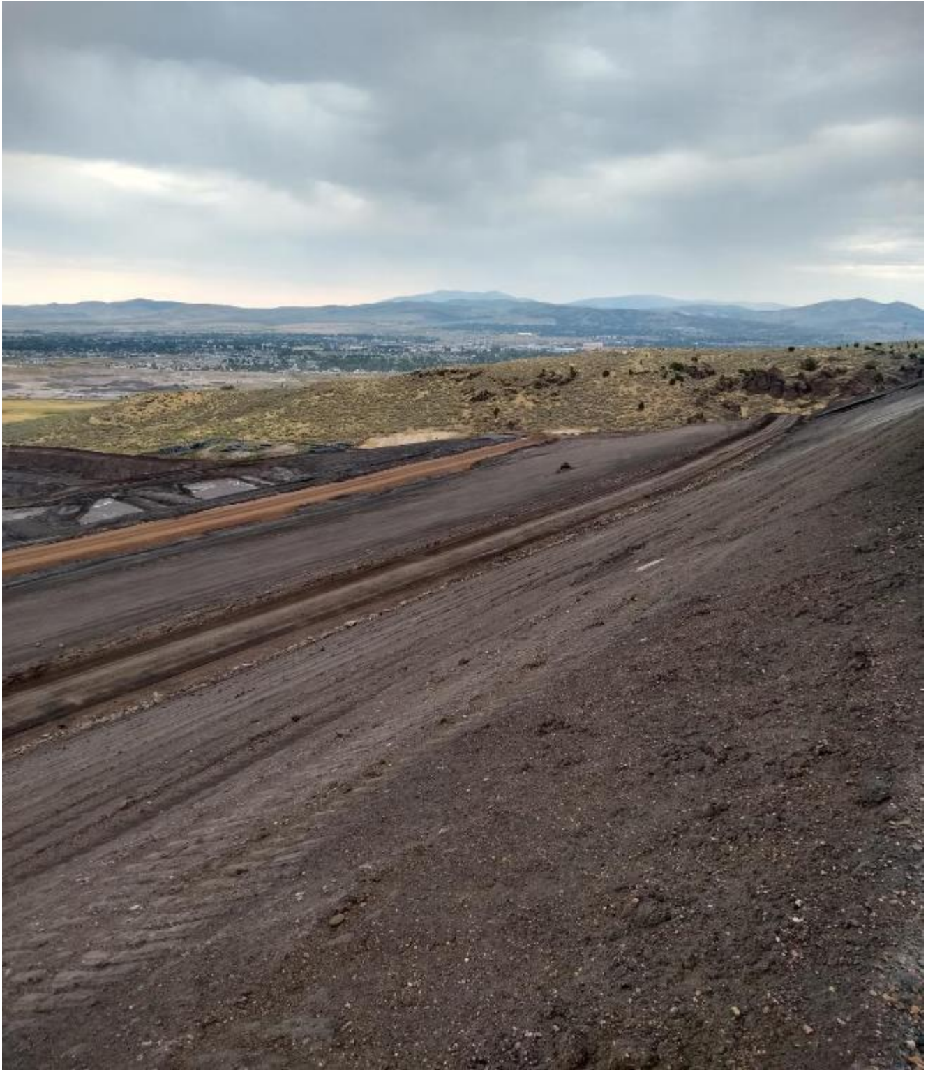
Photograph 21 - IMG_20200722_103247945_HDR: Gypsum Stack; phase 7C, looking straight down slope, ballast rock at 50' bench for extension liner, Phase I compartment
