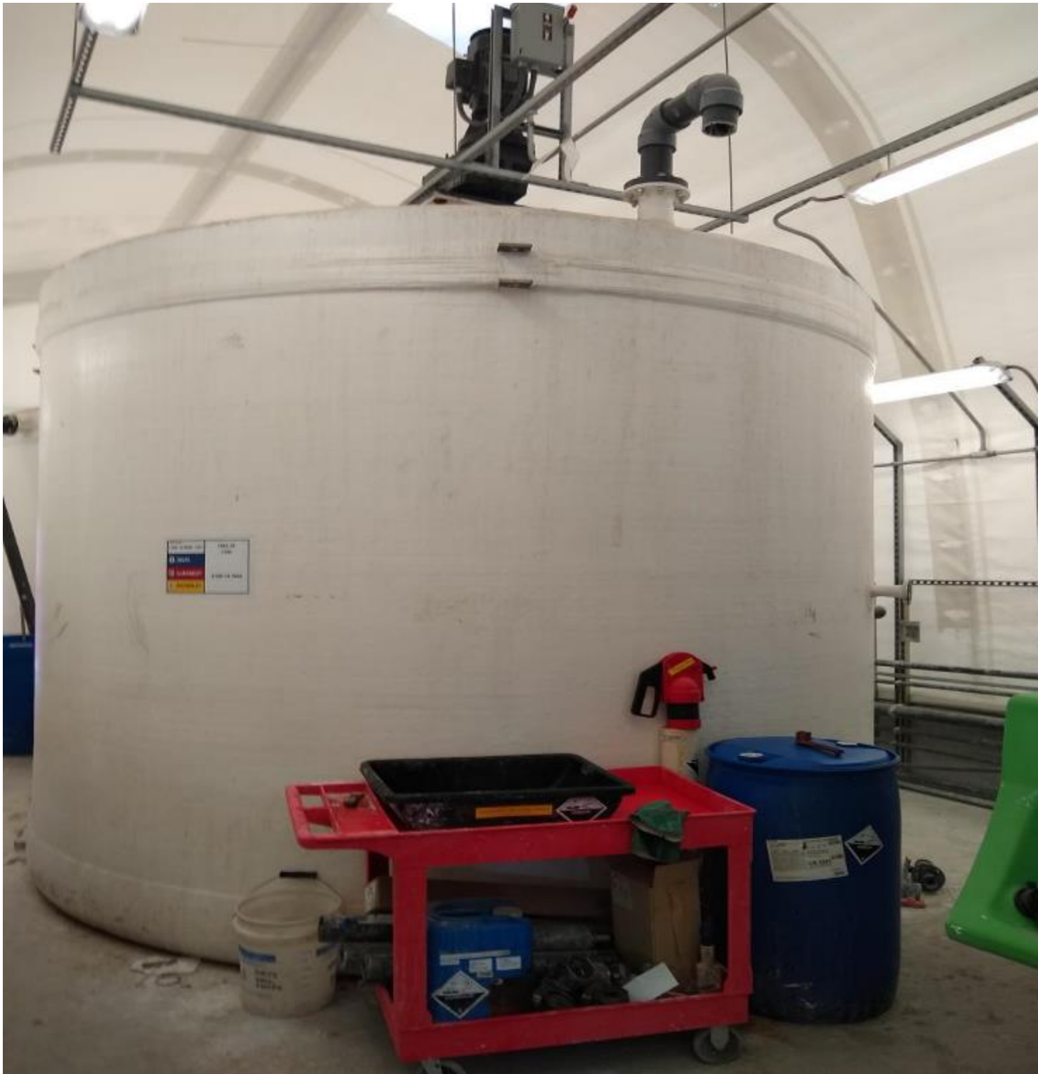
Photograph 12 - IMG_20200722_093654388: Inside former Well #419/423 Treatability Study Pilot tent; former milk of lime storage tank
