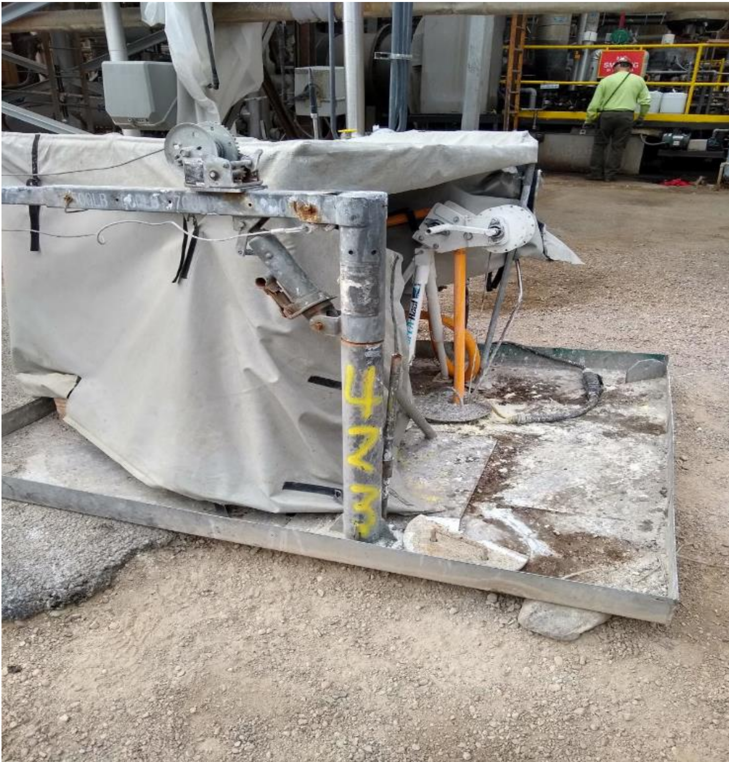
Photograph 13 - IMG_20200722_094015451_HDR: Phosphoric Acid Plant; well #423; protective covering; winch used to set well pump; yellow hose connected to pump at proper depth
