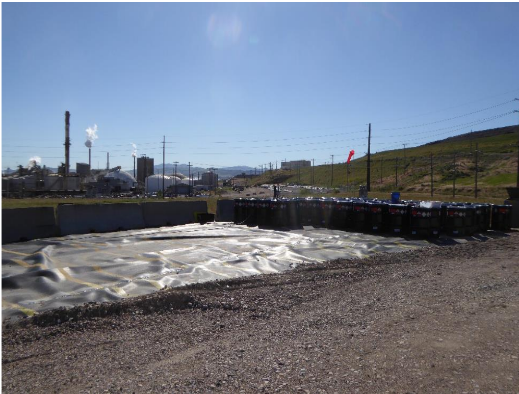
Temporary storage area for drums containing segregated material from remaining soil remedy area on FMC OU
