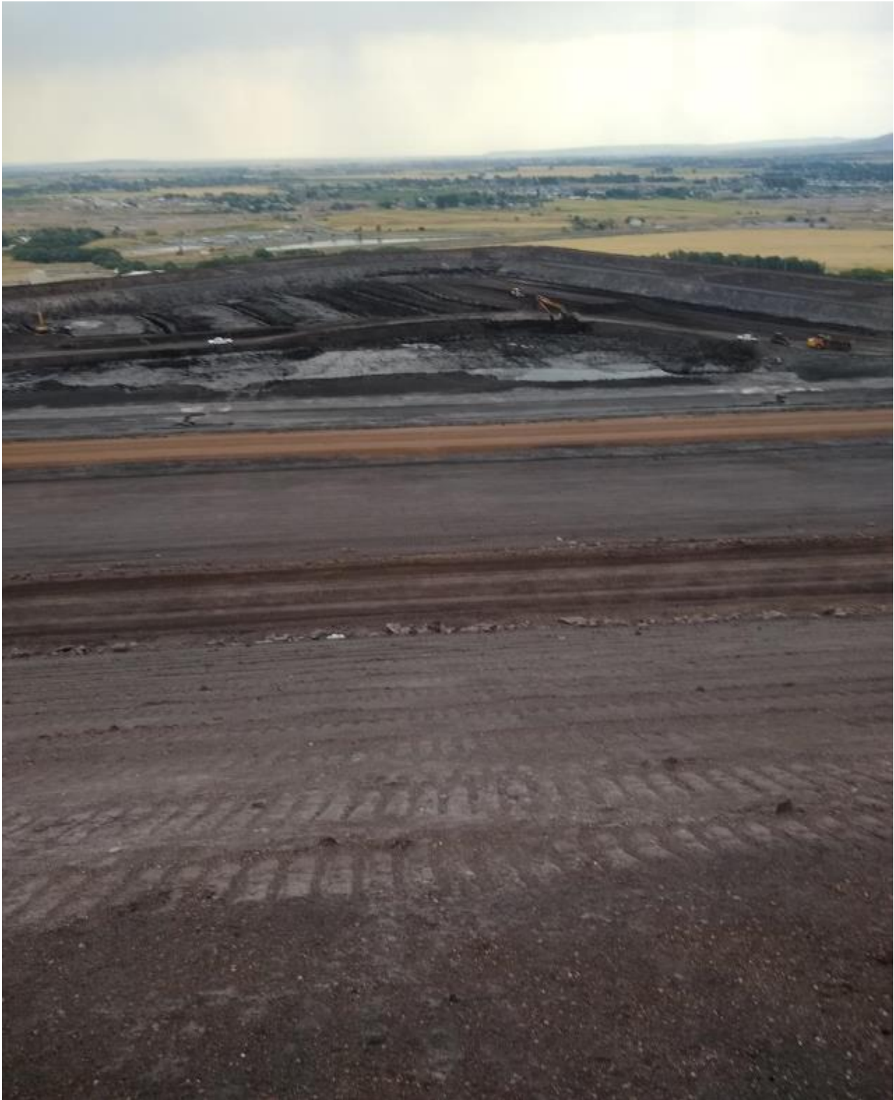
Photograph 20 - IMG_20200722_103243135: Gypsum Stack; phase 7C, looking straight down slope, ballast rock at 50' bench for extension liner from P compartment
