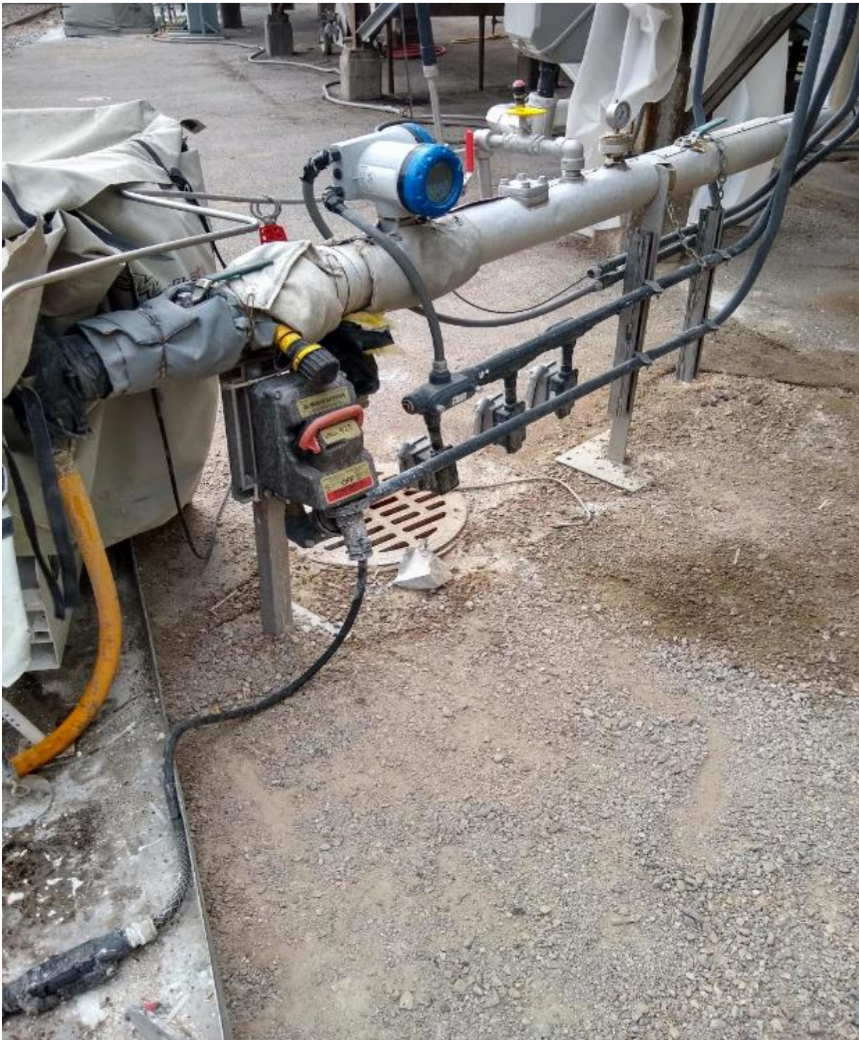
Photograph 15 - IMG_20200722_094154799_HDR: Well #419; piping and instrumentation used to route pumped water to the plant process
