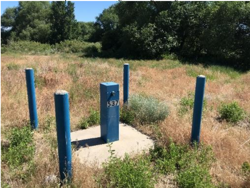
FMC OU locked monitoring well at Batiste Spring
