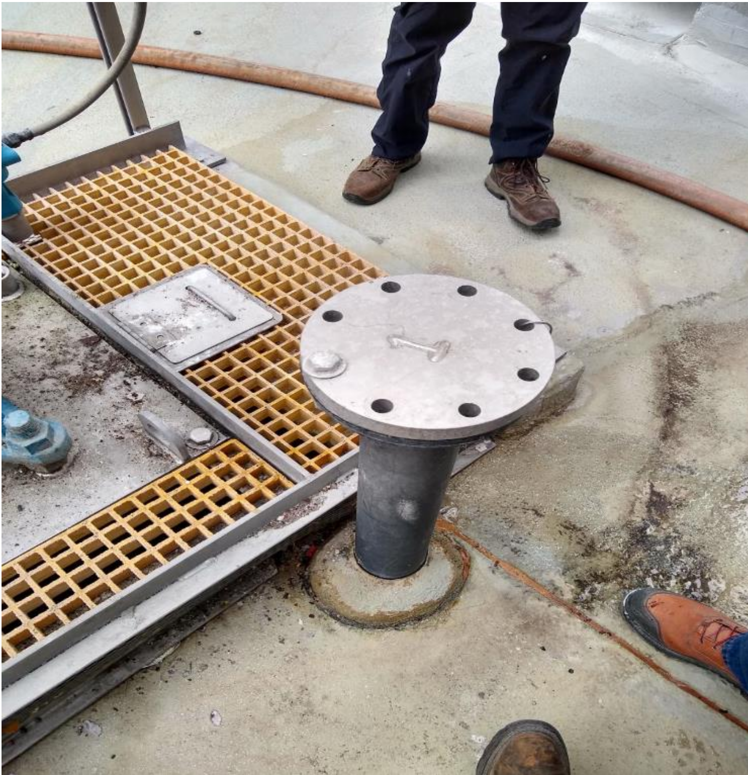
Photograph 7 - IMG_20200722_091848626_HDR: Sump #7; #1 secondary sump monitoring port, monitors between sump pad and within the interstitial
