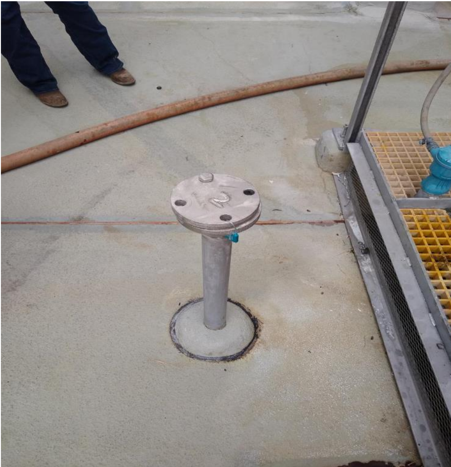
Photograph 8 - IMG_20200722_092110928: Sump #7; #2 secondary sump monitoring port, monitors below the interstitial containment and sump the sum
