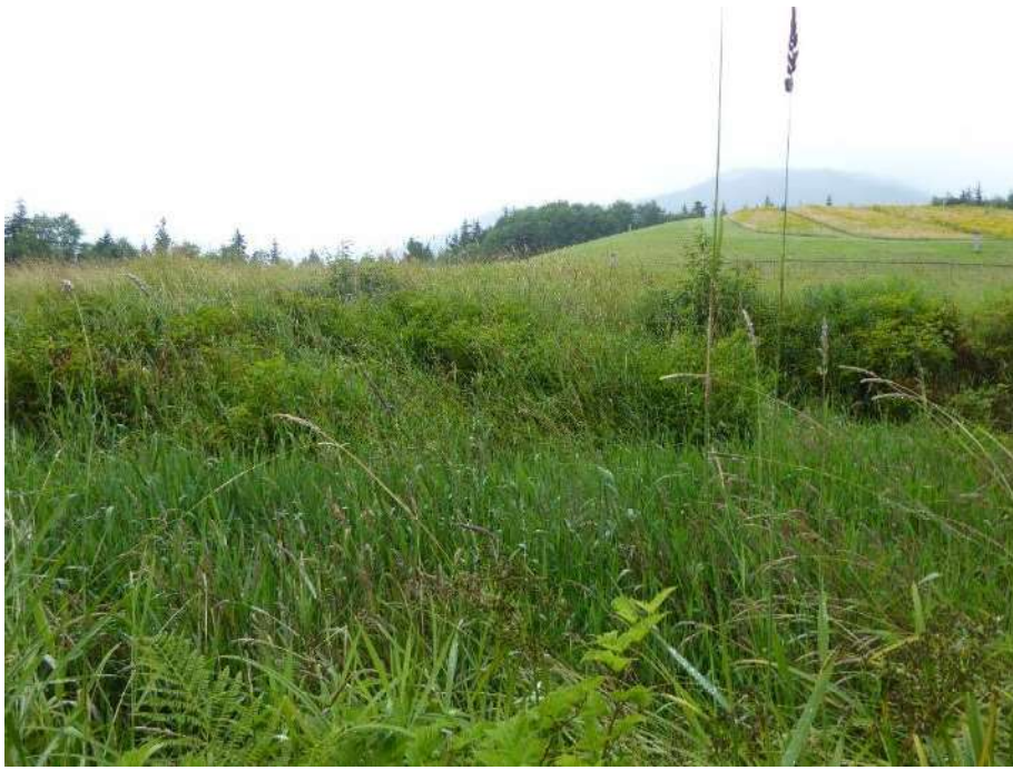
Leachate passive treatment system
