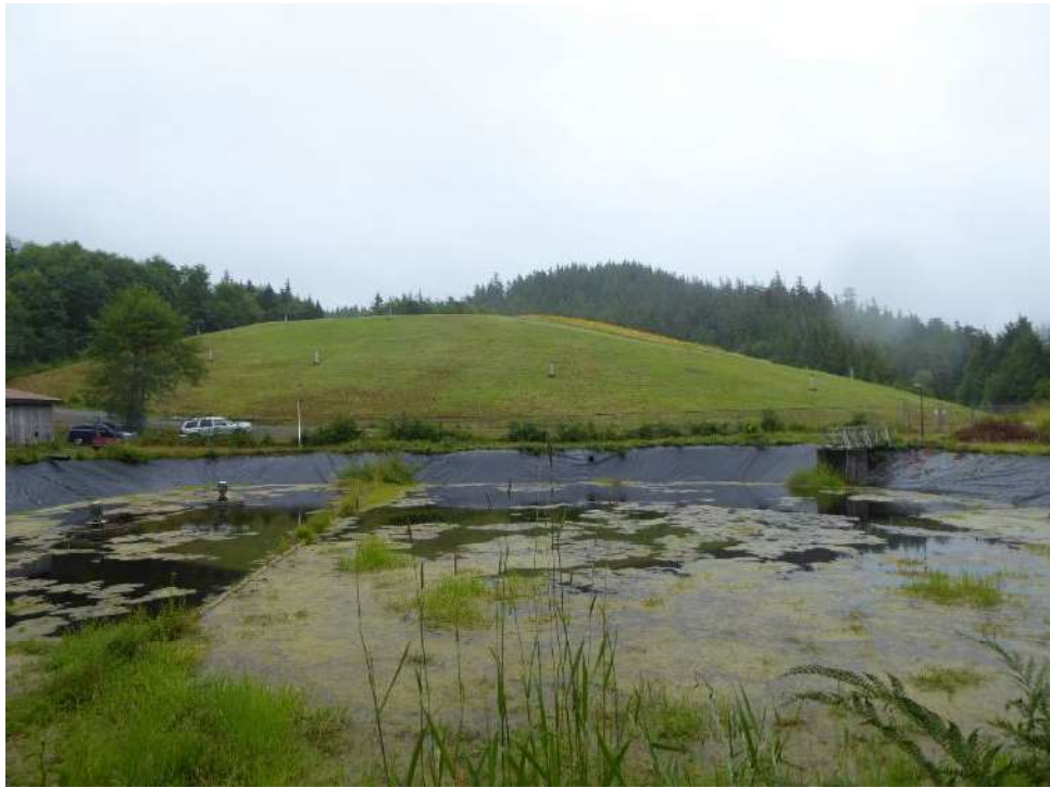
Leachate lagoon with landfill in background
