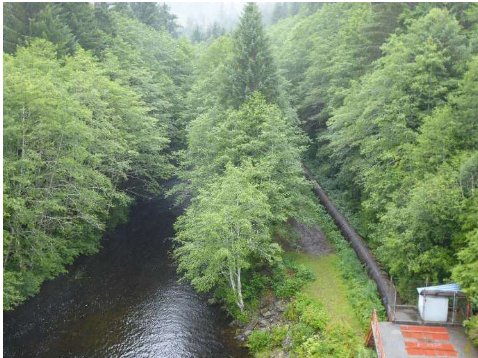
Pipeline and trail near dam at Connell Lake
