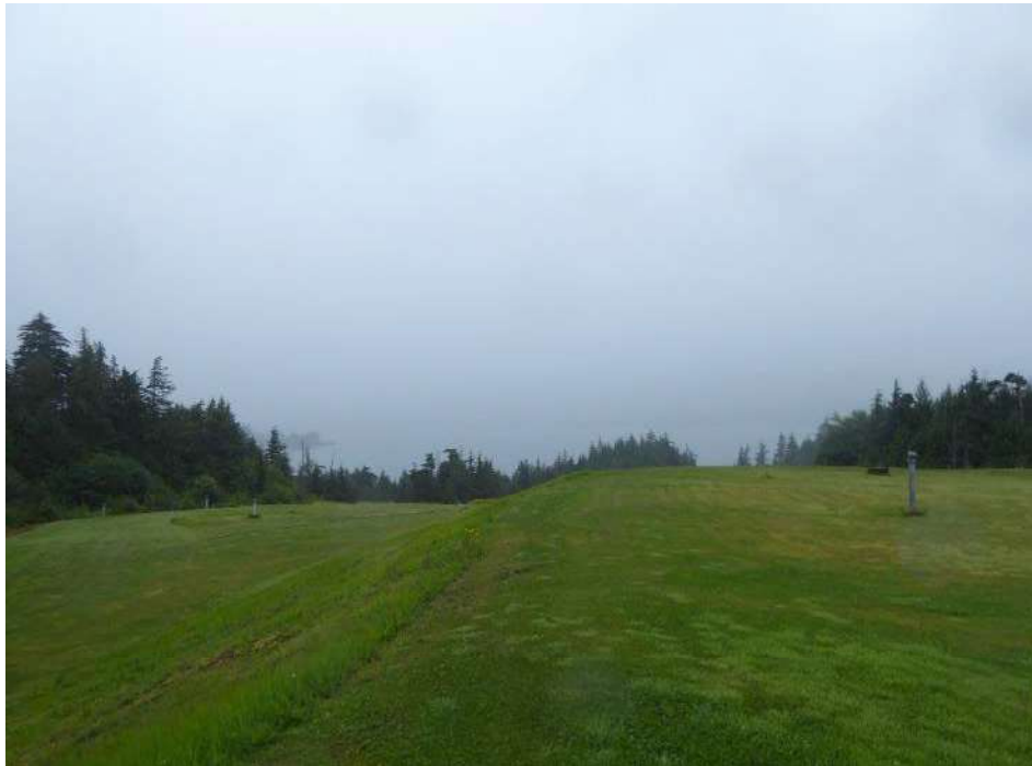
Wood waste and ash landfill
