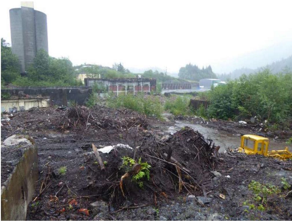
Former mill property foundations and debris
