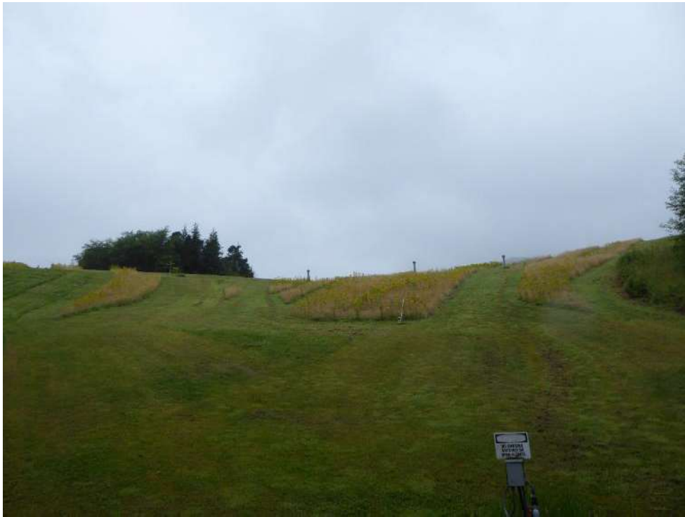
Wood waste and ash landfill
