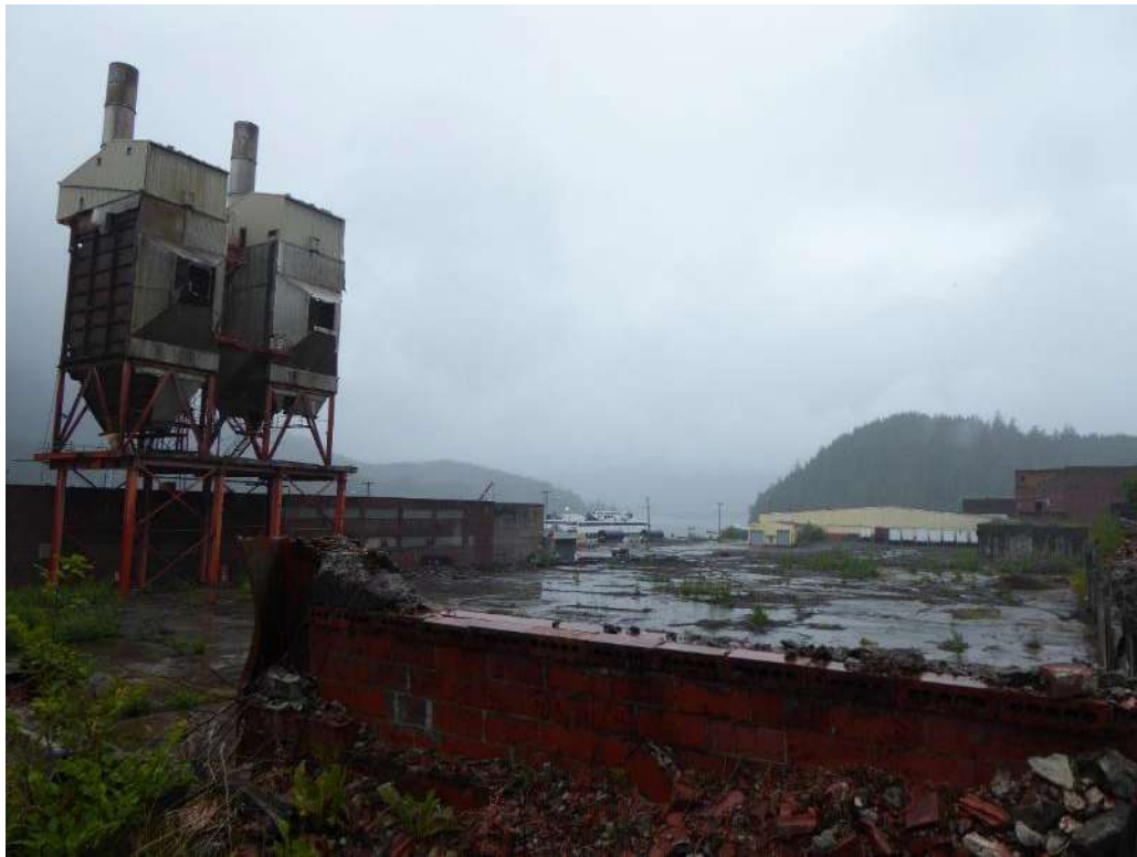
Former mill property foundations and debris
