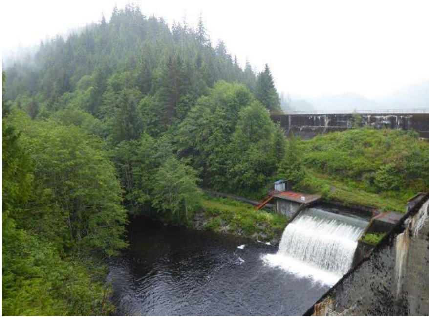
Dam at Connell Lake
