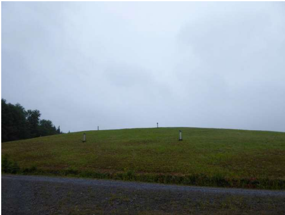
Gas vents on wood waste and ash landfill
