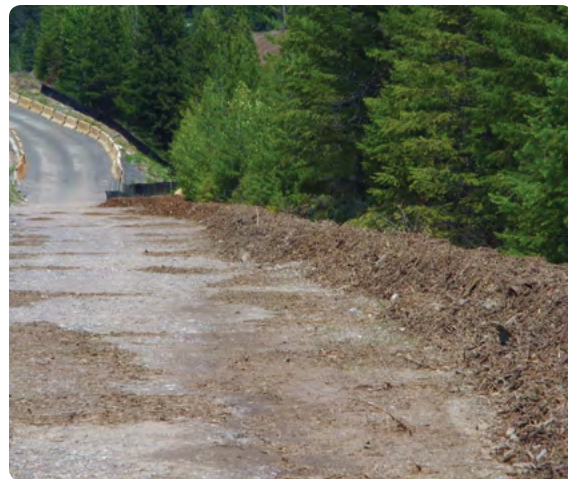
Placing shredded wood around waste repositories keeps soil and sediment out of local waterways.
