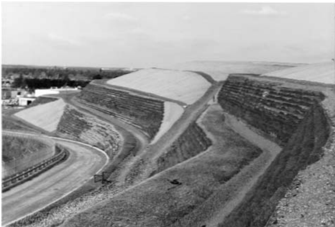
Figure 6-27. Constructed Reinforced Soil Slope Cover System for a Hazardous Waste Landfill.
