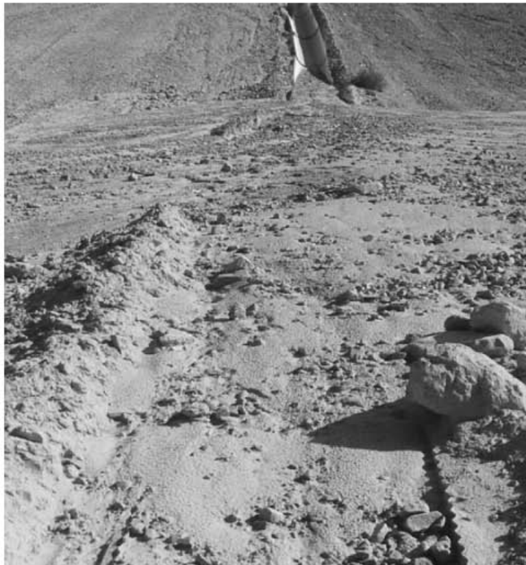
Figure 7-19. Failed Surface-Water Runoff Control System for Another Portion of the Closed MSW Landfill Located at an Arid Climate Site and Shown in Figure 7-18.
