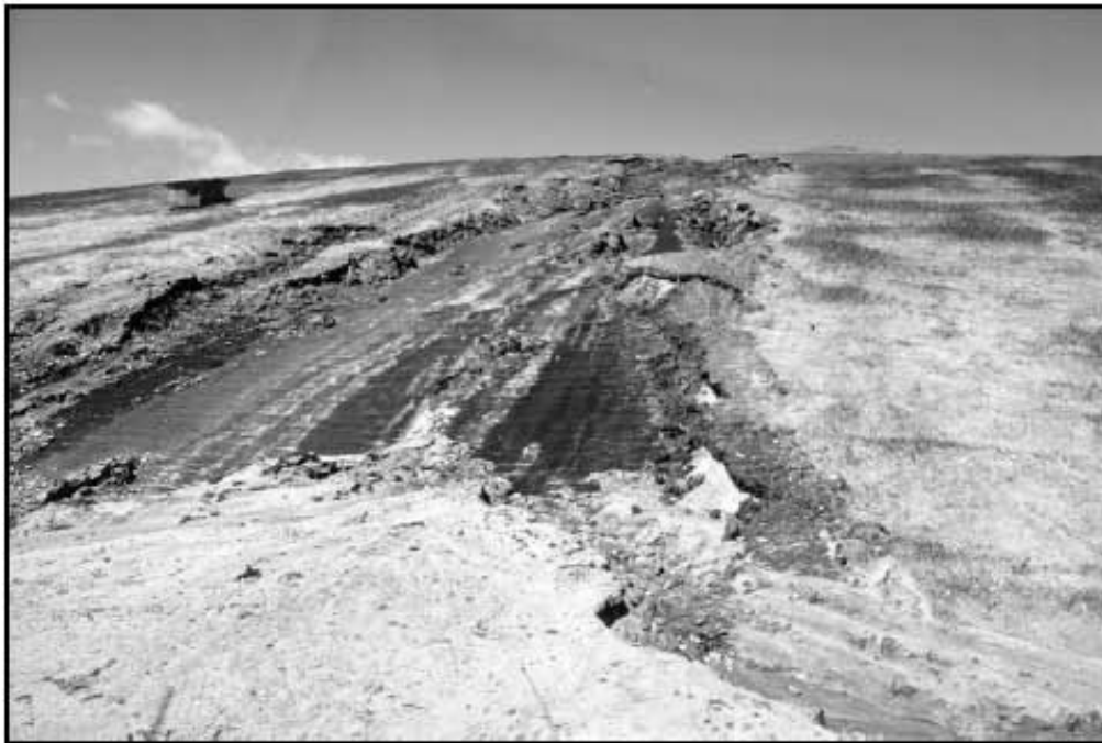
Figure 7-17. Deep Gullies Through the Topsoil and Sand Drainage Layers Exposed the GM Barrier on 60-m Long, 3H:1V Landfill Sideslopes.
