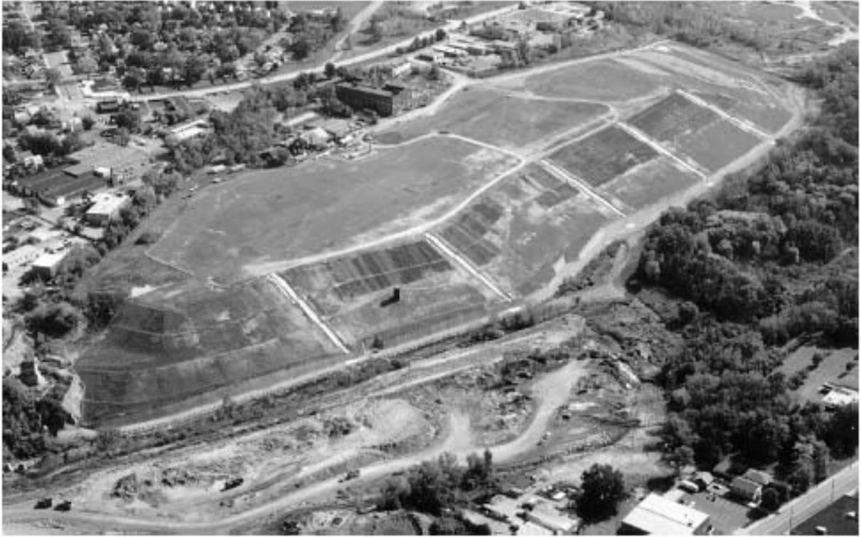
Figure 6-32. Aerial View of Constructed Cover System with a Pre-cast Concrete Crib Wall Waste Buttress at a Sanitary Landfill.
