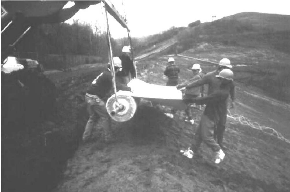
Figure 7-12. GCL Panels Deployed on Slopes of Cincinnati, Ohio Test Plots by Pulling Them Downslope from a Spreader Bar at the Slope Crest.
