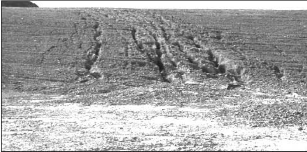
Figure 7-18. Gullies on a RCRA Subtitle D Cover System without Surface-Water Runoff Control System and Located in an Arid Setting.
