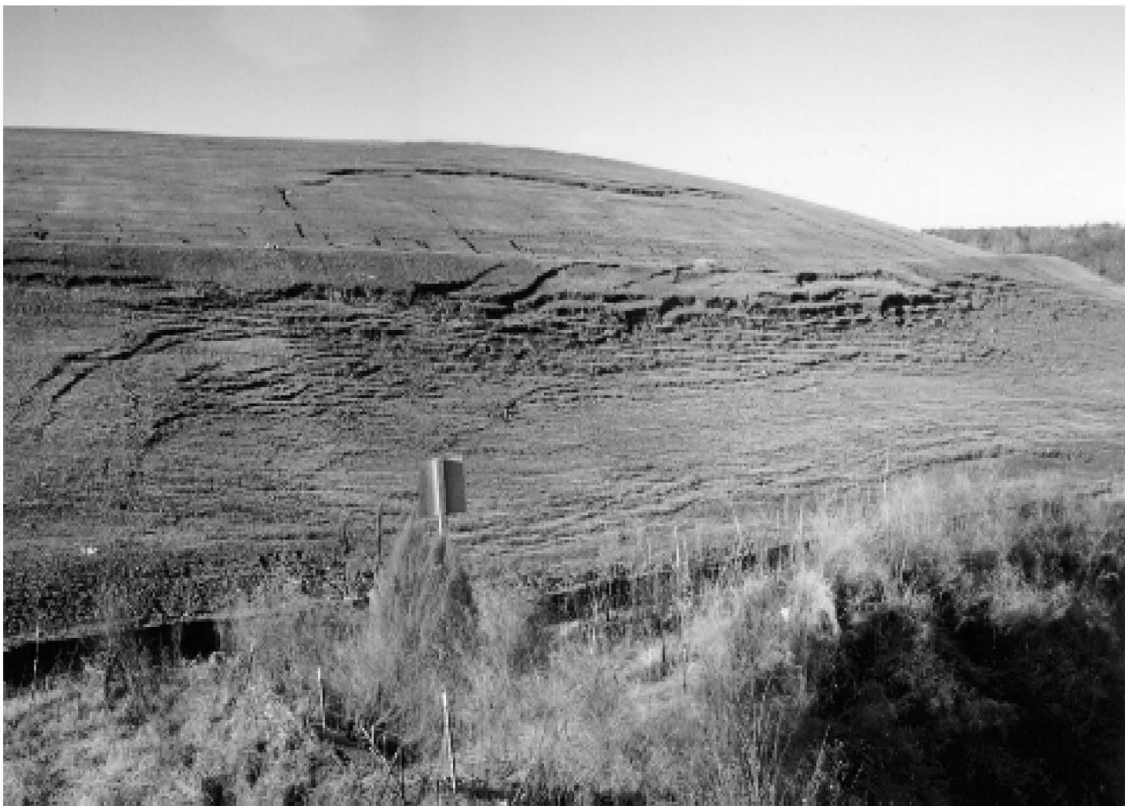
Figure 6-1. Example of Cover System Slope Stability Problem. The Topsoil Surface/Protection Layer Slid Downslope Over the Reinforced GCL Barrier.
