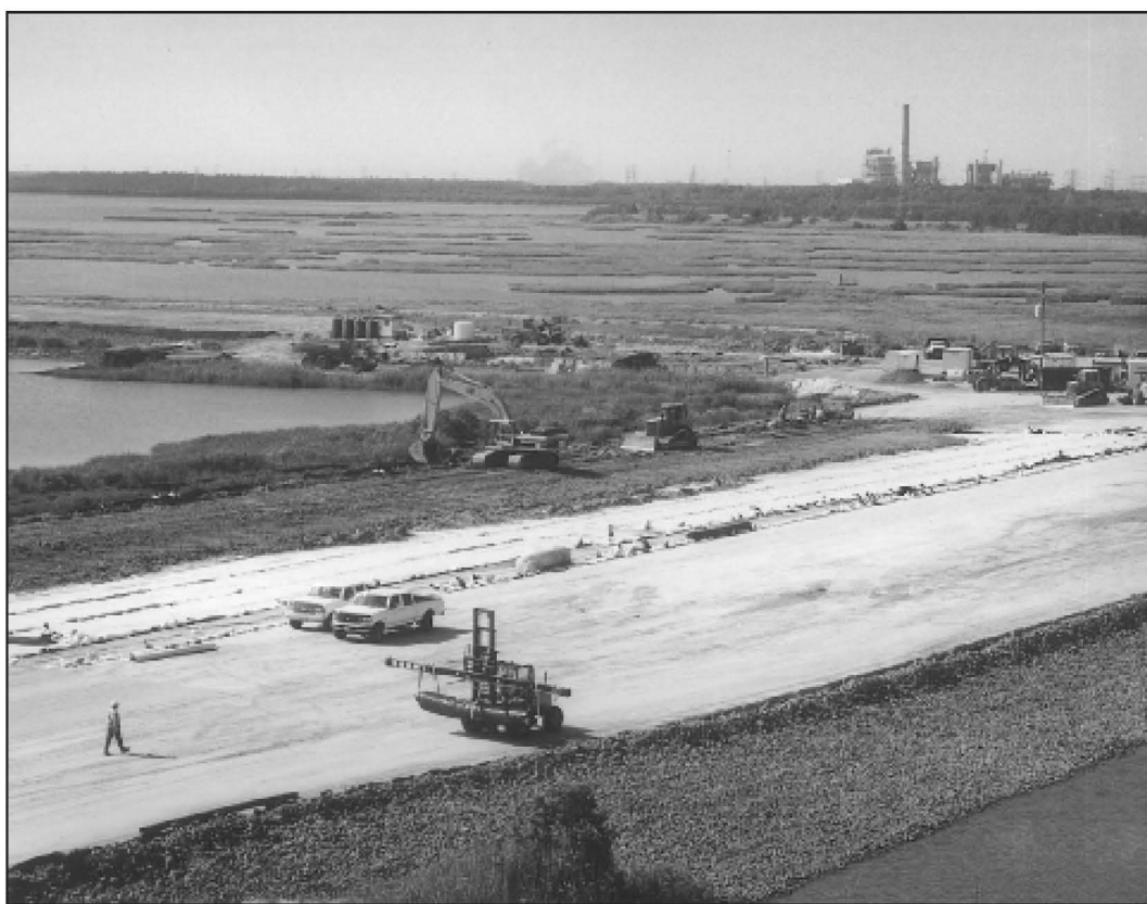
Figure 6-35. Example of a Lightweight Cover System Constructed Over Soft Waste and Soil at CERCLA site near Beaumont, Texas.
