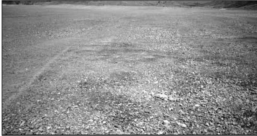
Figure 7-25. Surface Stains on Landfill Cover System Caused by Landfill Gas.
