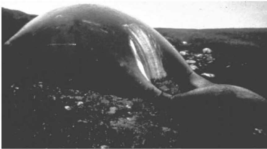
Figure 7-23. GM “Whale” Caused by Gas Pressures Beneath the GM.
