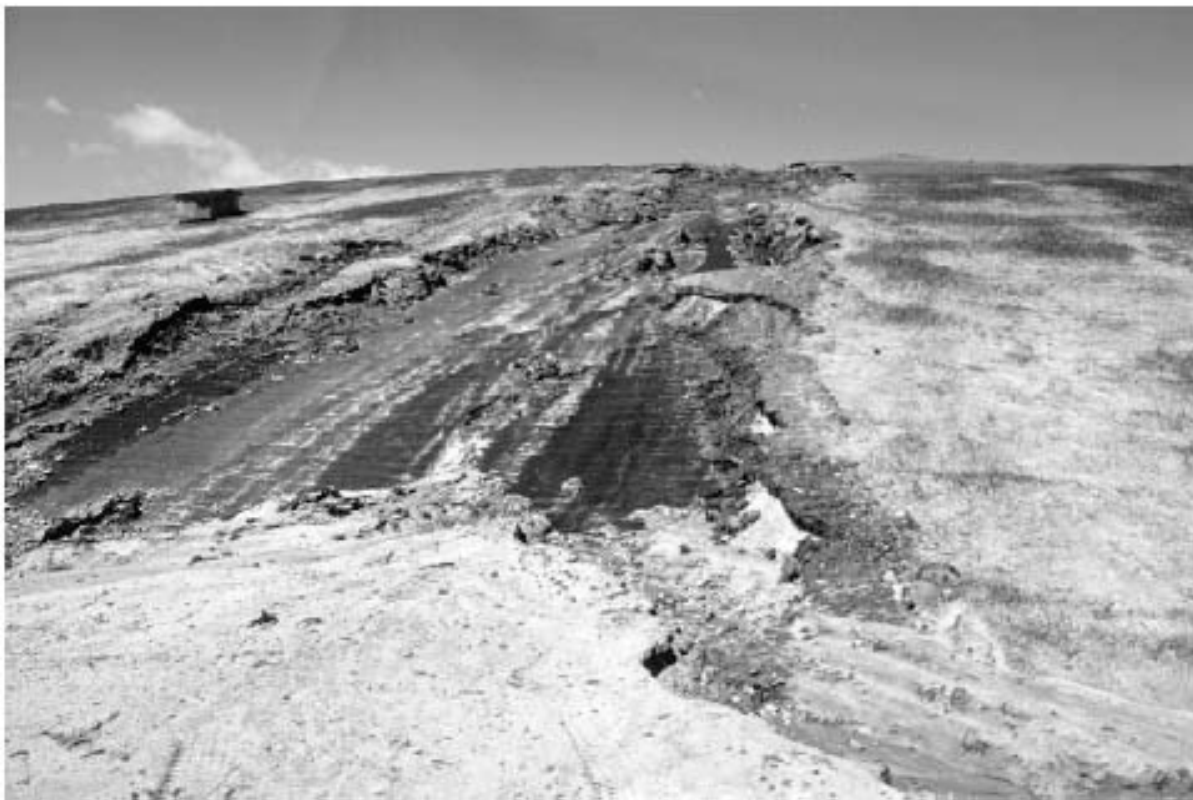
Figure 2-6. Deep Gullies Through the Topsoil and Sand Drainage Layers Exposed the GM Barrier on 60-m Long, 3H:1V Landfill Sideslopes.
