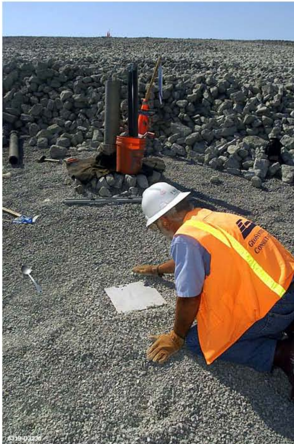
Figure 8-11. Placement of GPR Target on Top of Drainage Layer (and at the Bottom of the Protection Layer) During Cover System Construction.
