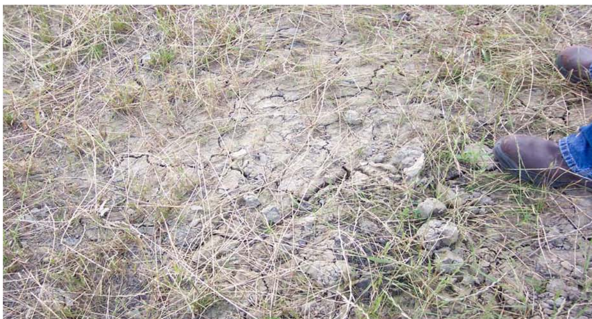
Figure 5-3. Surface Cracks at a Landfill
