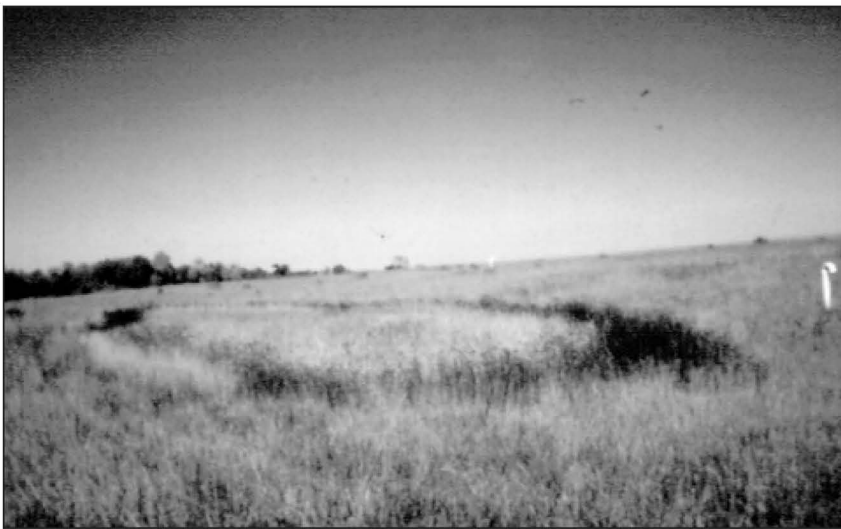
Figure 7-24. Landfill Cover System Vegetation Killed by Landfill Gas.
