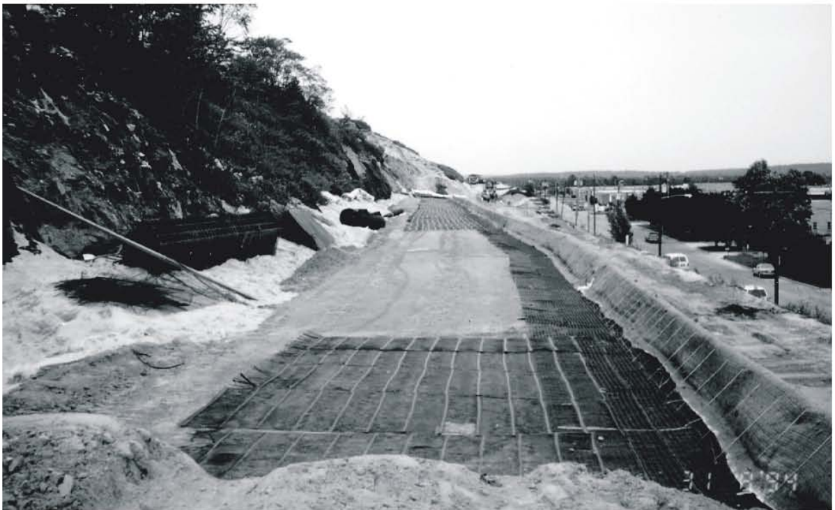
Figure 6-26. Construction of Reinforced Soil Slope Cover System on Steeper Slope Sections of a Hazardous Waste Landfill.
