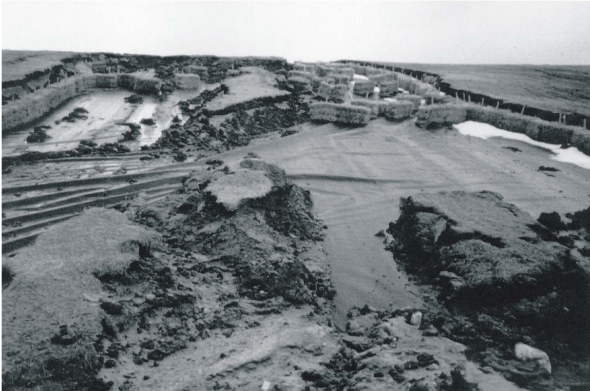
Figure 6-2. Example of Cover System Slope Stability Problem. The Topsoil Surface/ Protection Layer and Underlying Sand Drainage Layer Slid Downslope Over the Textured HDPE GM Barrier.
