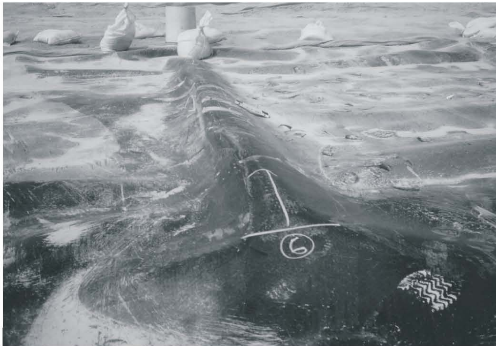
Figure 7-7. Wrinkles Developed in an HDPE GM and Folded Over During Placement of Cover Soil.
