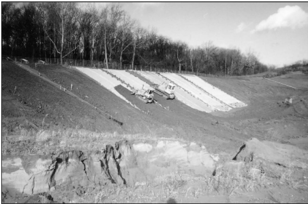
Figure 7-13. Cover Soil on the Cincinnati, Ohio Test Plots Placed over the Geosynthetics from the Slope Toe Upward.
