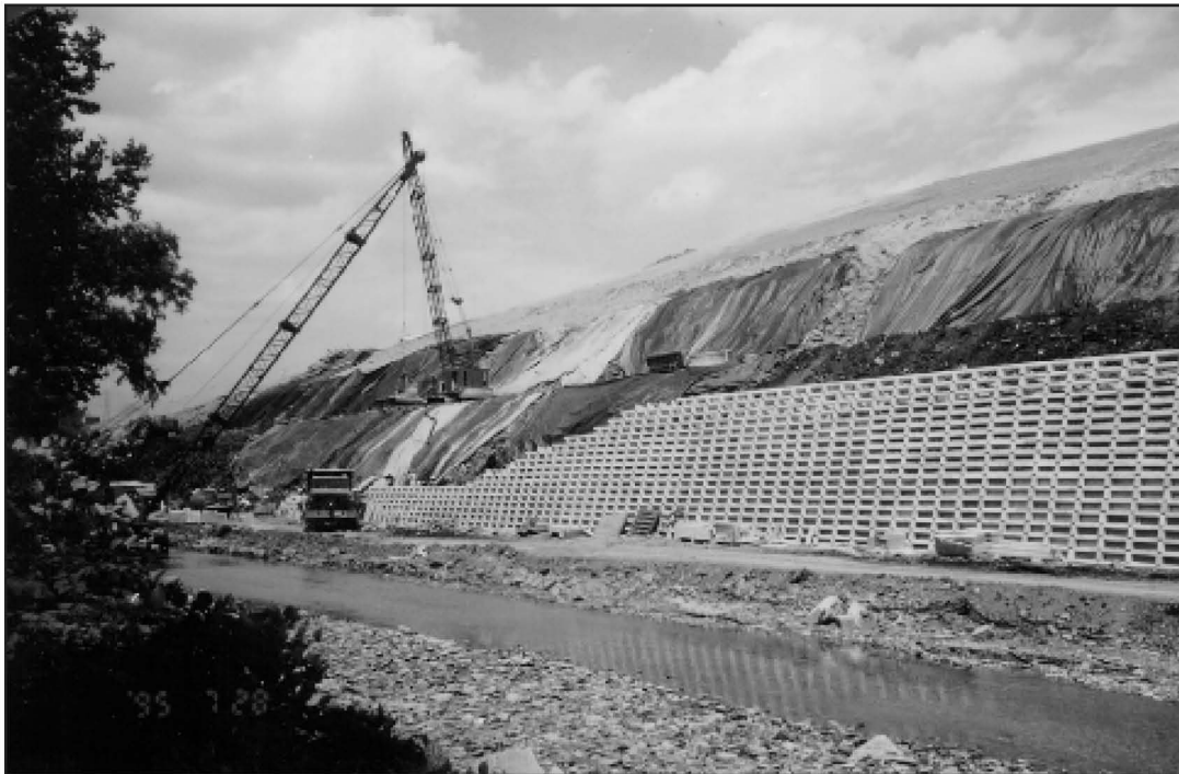
Figure 6-31. Construction of the Pre-cast Concrete Crib Wall Waste Buttress for a Sanitary Landfill.
