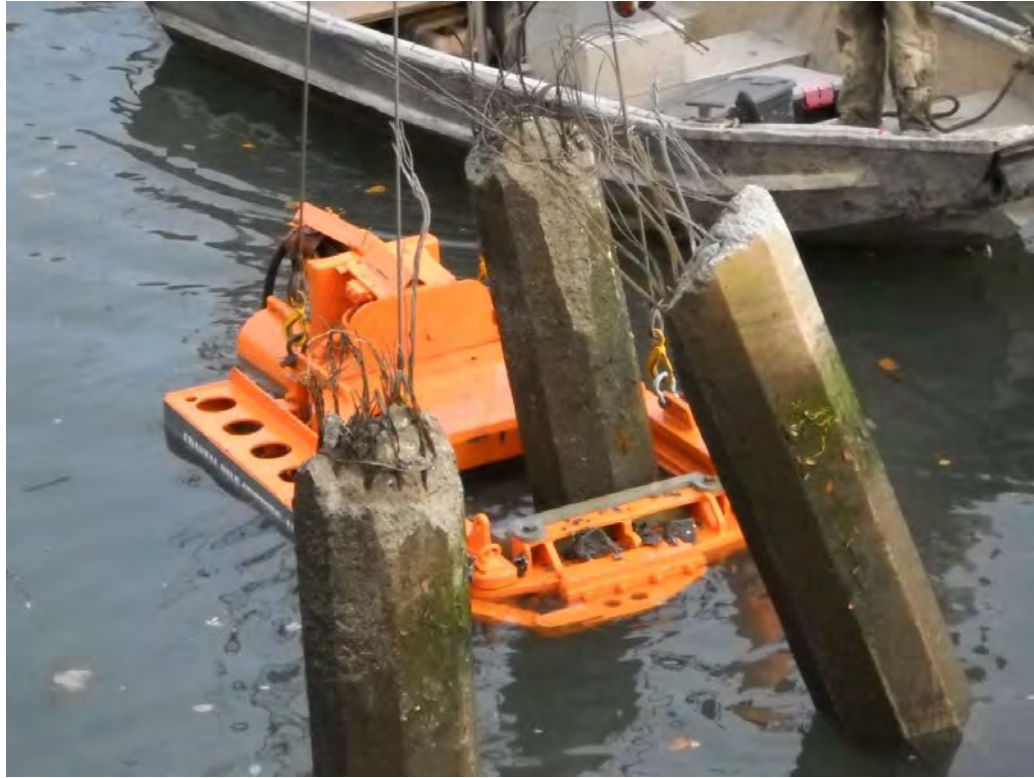
Photograph 3-13. Pier Demolition—Pile Cutting with Shear (December 16, 2011)
