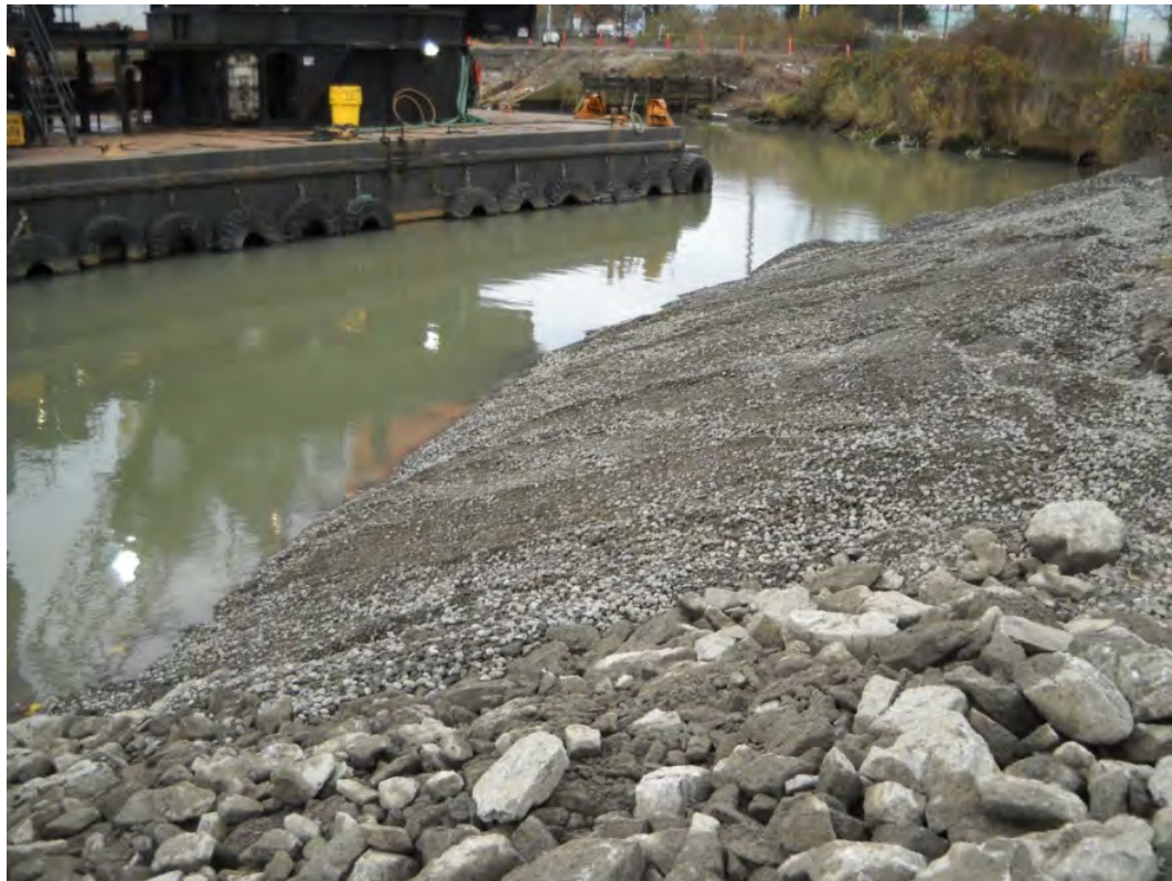
Photograph 3-8. Bank Capping—Filter Material ( top : December 6, 2011; bottom : December 8, 2011)
