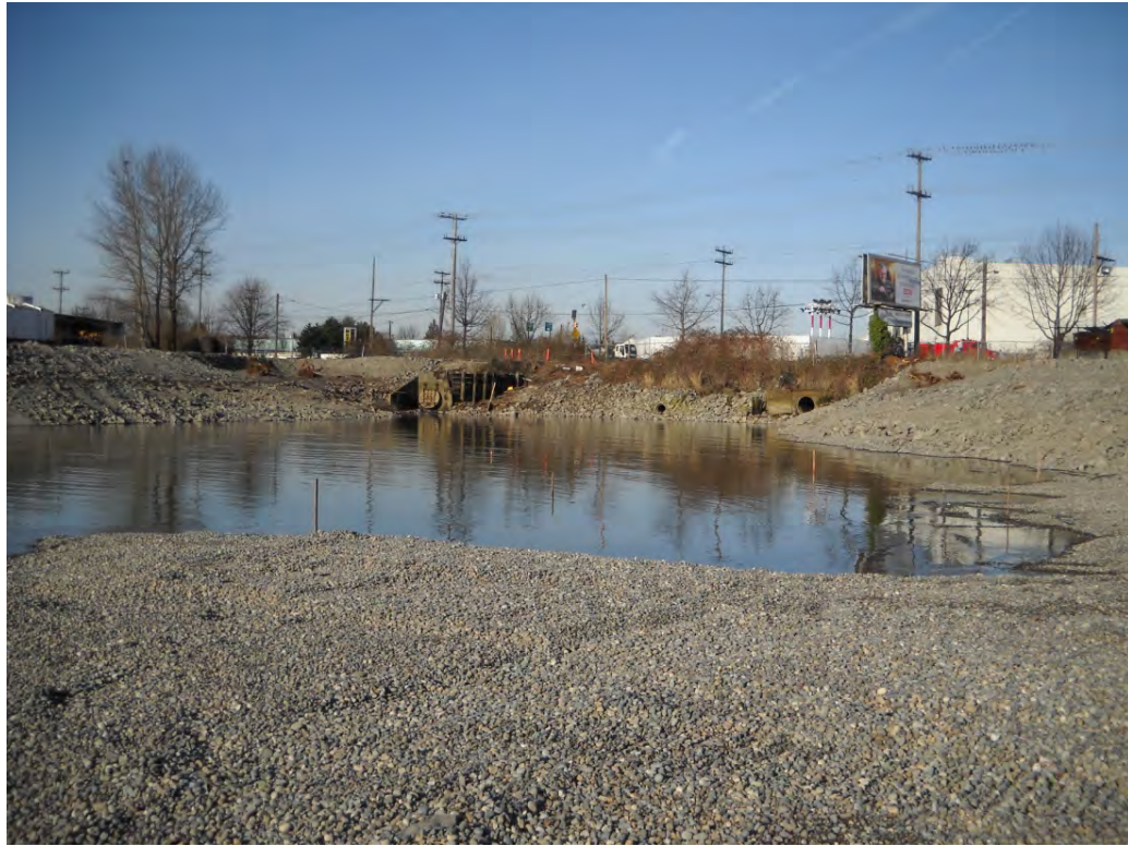
Photograph 3-15. Waterway Capping (January 27, 2012)
