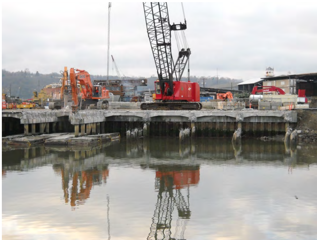
Photograph 3-12. Pier Demolition ( top : December 7, 2011; bottom : December 5, 2012)
