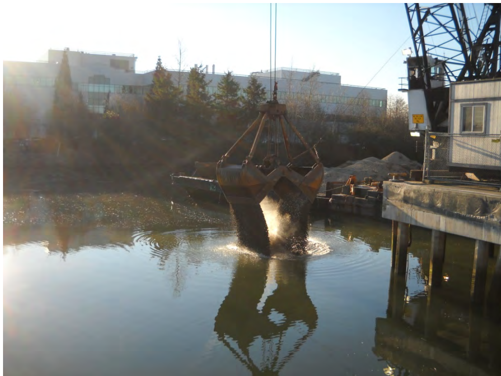
Photograph 3-16. Boundary Area Material Placement (February 7, 2012)
