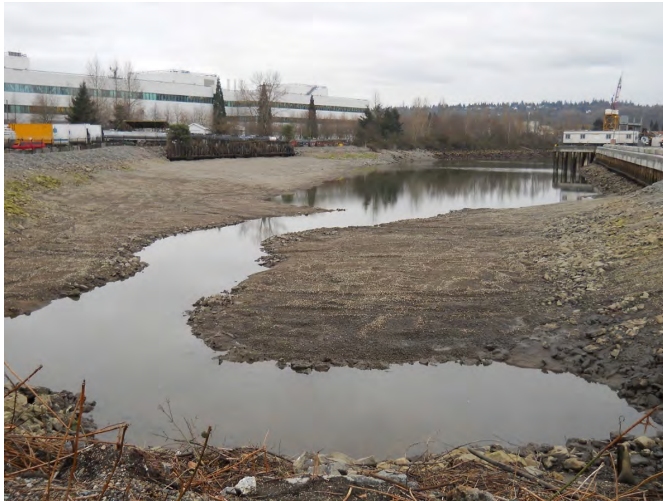
Photograph 3-14. Waterway Capping ( top : January 10, 2012; bottom : February 13, 2012)
