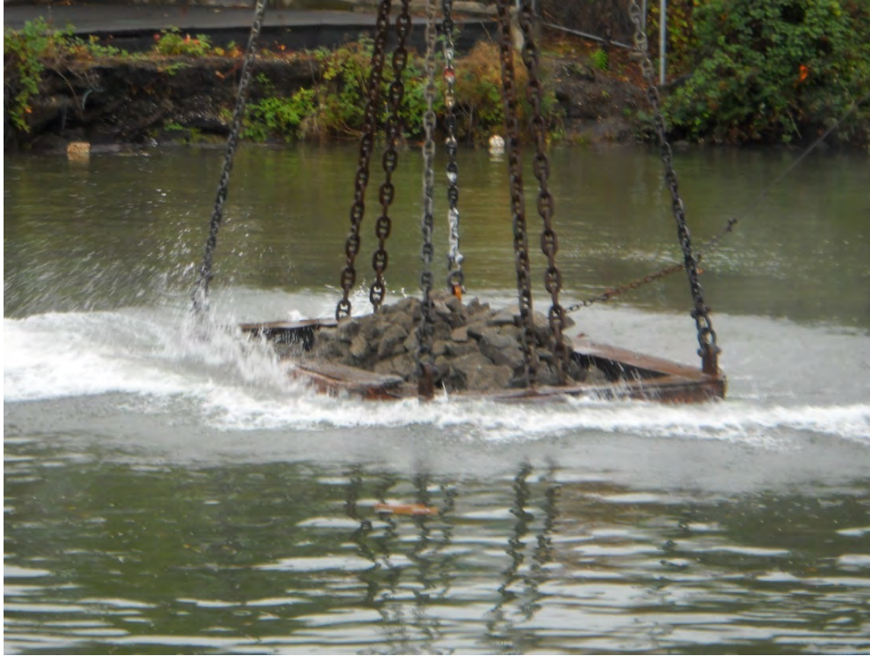
Photograph 3-1. Placement of Boundary Berm with "Bombay Box" (October 3, 2011)
