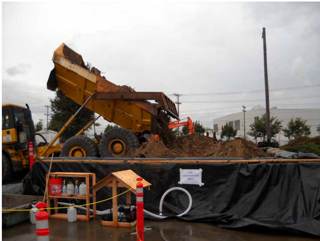
Photograph 3-5. Bank Excavation (October 5, 2011)
