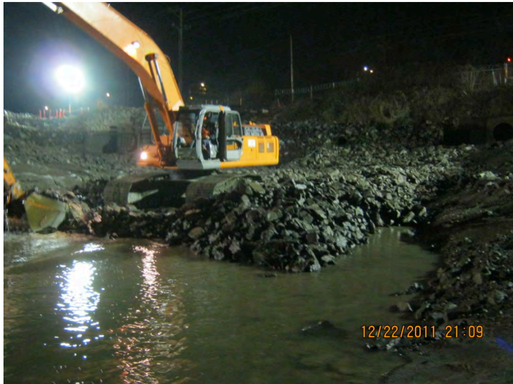
Photograph 3-11. Outfall Area Capping (December 22, 2011)
