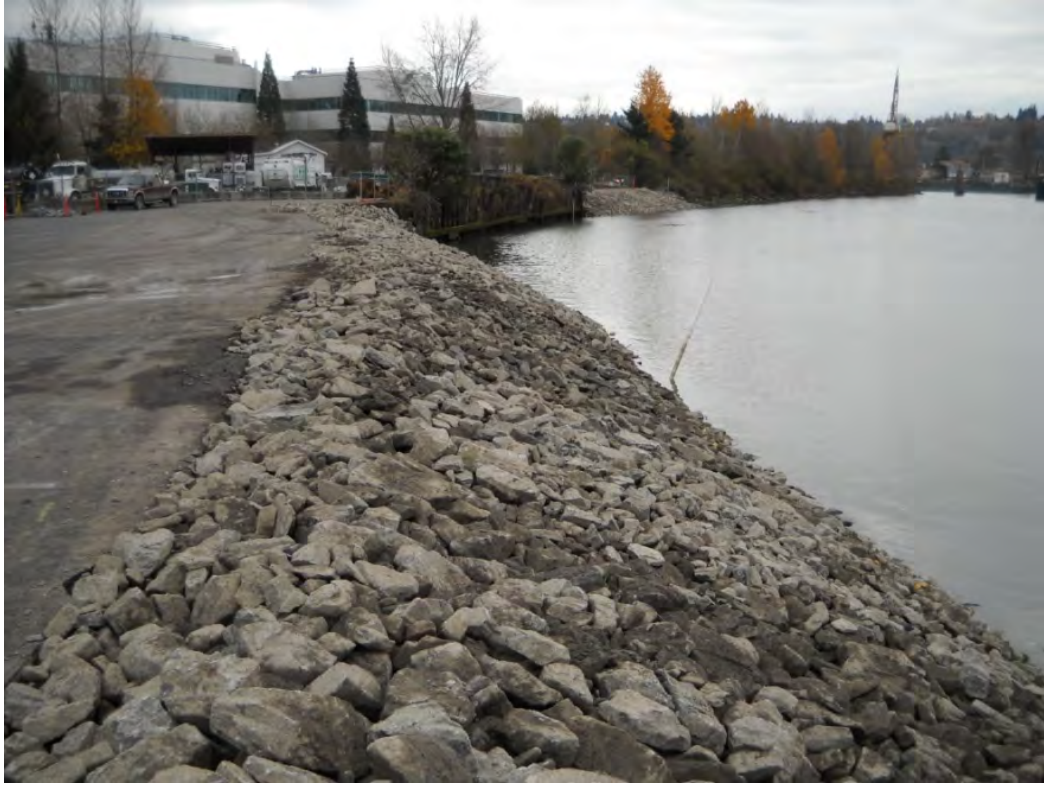
Photograph 3-9. Bank Capping—Cap Armor (December 8, 2011)
