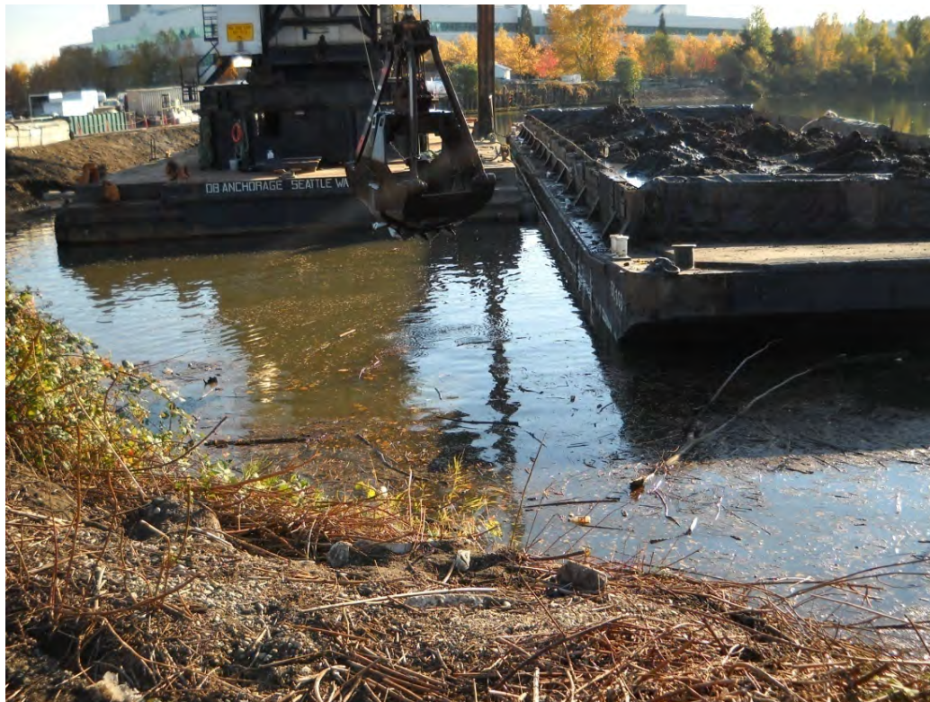
Photograph 3-3. Dredging of Sediment (November 10, 2011)
