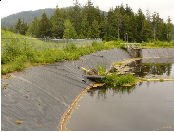
Photo 37. Geomembrane lined sediment lagoon at the KPC landfill. Note six foot chain link fence surrounding lagoon. Inlet pipe.
