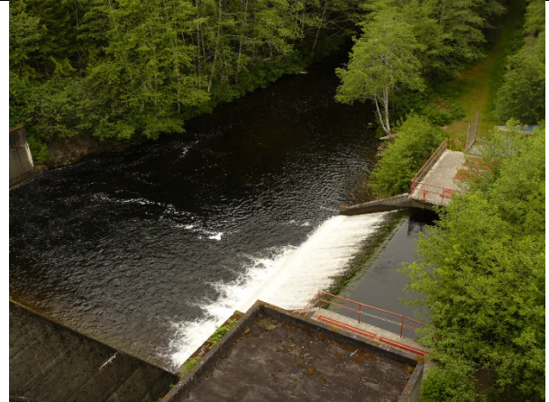
Photo 52. Outflow from dam and intake point for wood pipeline.
