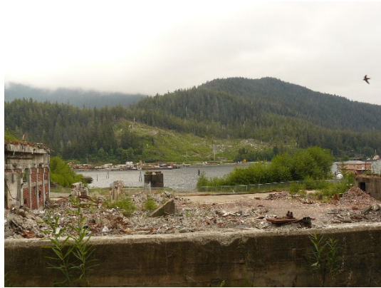
Photo 8. View to south of rubble from former woodroom building.
