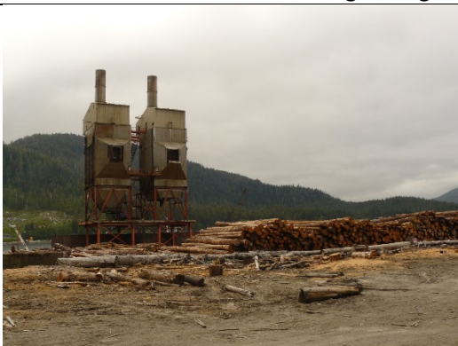
Photo 5. Electrostatic precipitators from KPC mill. Alcan log sorting yard on former boiler house site.
