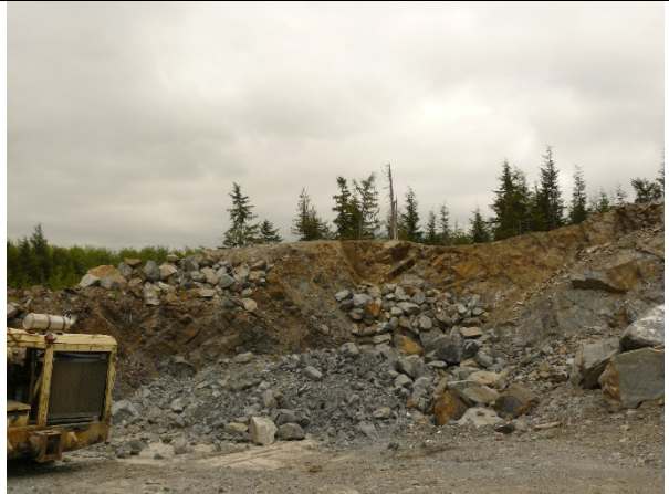
Photo 36. On-site quarry used for fill rock.
