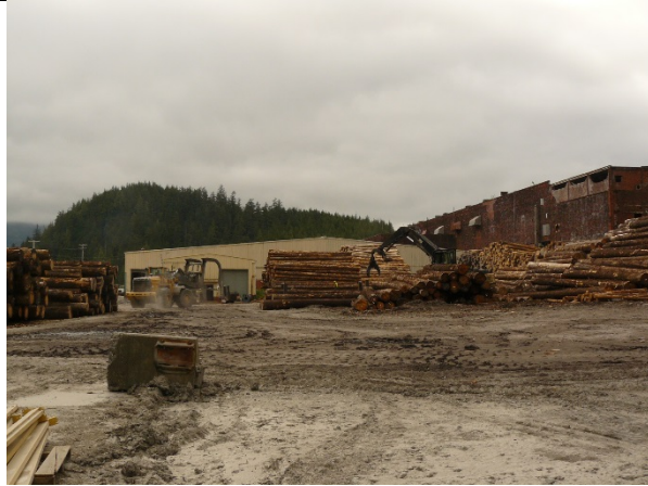
Photo 10. View west of former boiler house building, now used by Alcan as a log sorting yard. No. 2 Warehouse is the yellow building in the background
