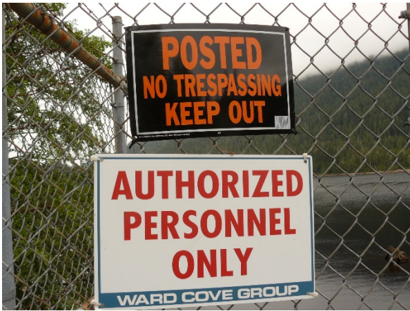
Photo 49. Locked gate at Connell Lake dam structure.
