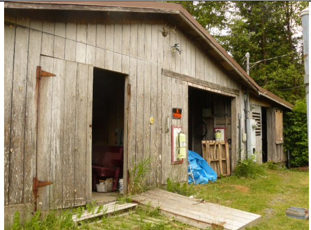
Photo 40. Landfill generator and storage building.
