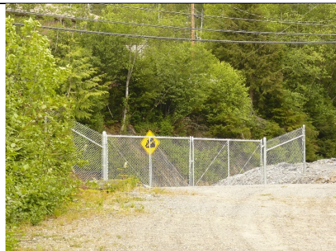
Photo 6. New fence installed by Ketchikan Gateway Borough at N. Tongass Hwy. Site perimeter fence was removed by KGB.
