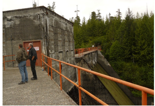
Photo 50. Connell Lake Dam structure
