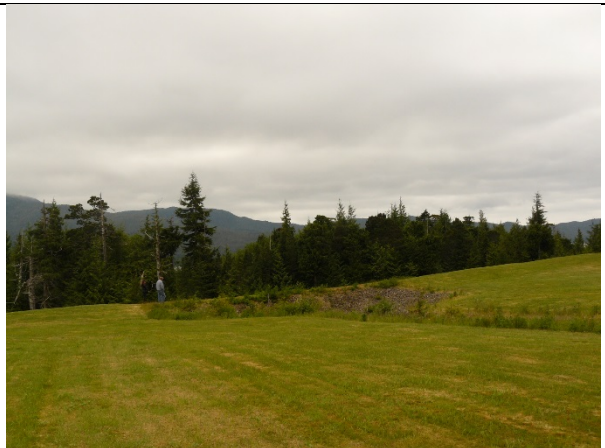
Photo 48. Surface overland flow drainage swale on top of landfill.
