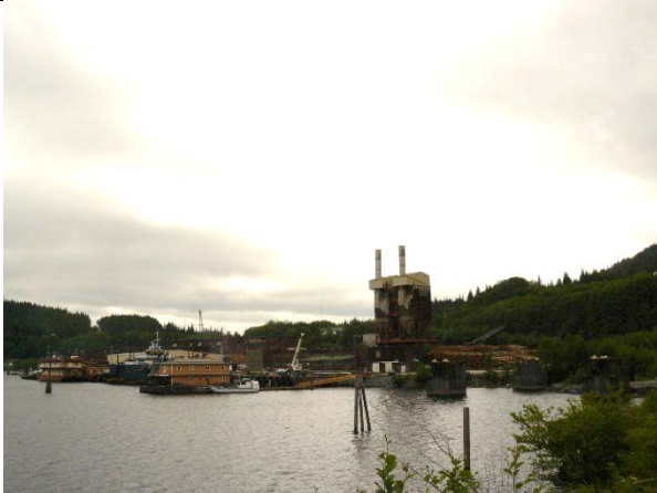
Photo 15. View Northwest from AMHS parking lot towards former mill site.
