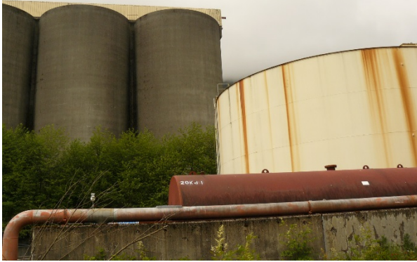
Photo 13. View north of silo's and 1 million gallon fuel tank. Tank interior has been restored for future marine fuel storage and distribution.
