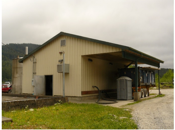
Photo 32. Former KPC effluent neutralization building. Used by Full Cycle LLC.
