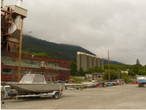
Photo 7. View east of silo's and former demolished woodroom and boiler house buildings.
