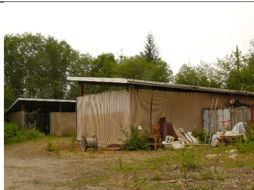
Photo 4. Former Hazardous Waste buildings. Floor drains to catchment basin.
