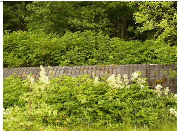
Photo 54. Wood stave pipeline
