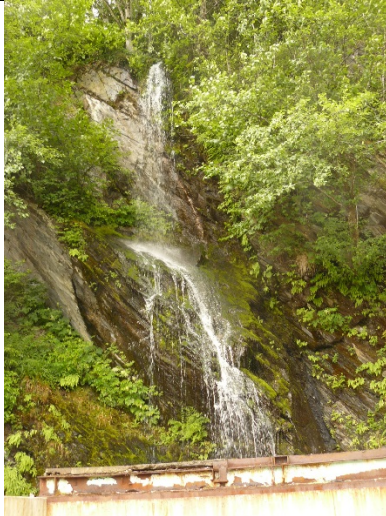
Photo 9. Leaking pipe 'waterfall' to north of demolished woodroom building
