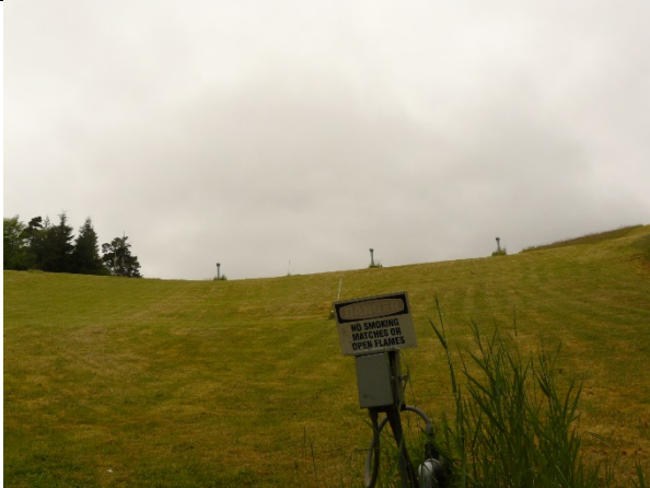
Photo 45. Looking upslope from landfill toe. Former manhole vent in foreground; passive landfill vents seen on landfill horizon.
