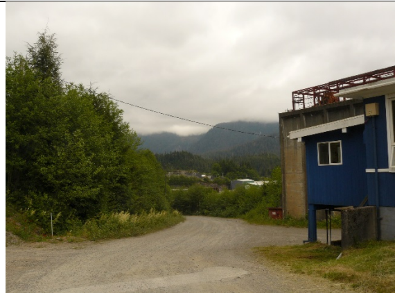
Photo 2. View to southeast downslope from administration building
