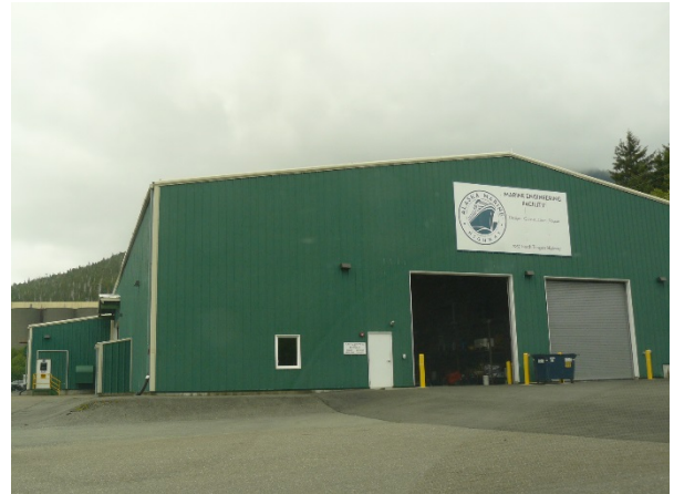
Photo 14. View of Alaska Marine Highway System Engineering building on east end of mill site.
