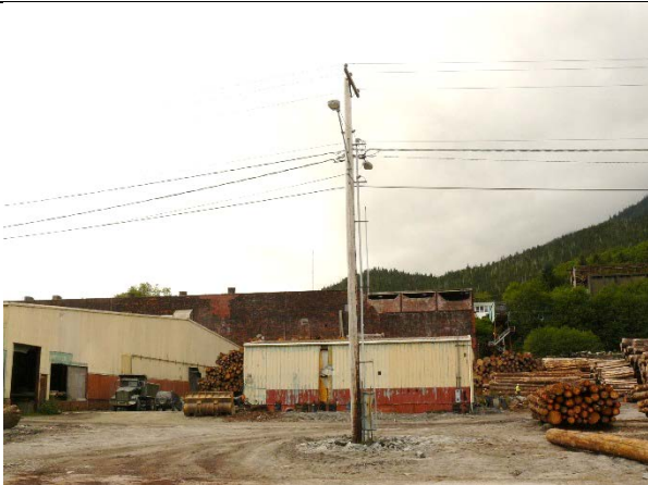
Photo 29. View north of No. 2 Warehouse (on left). Former paint shop removed from behind building in center. Note overhead powerlines installed by KGB.
