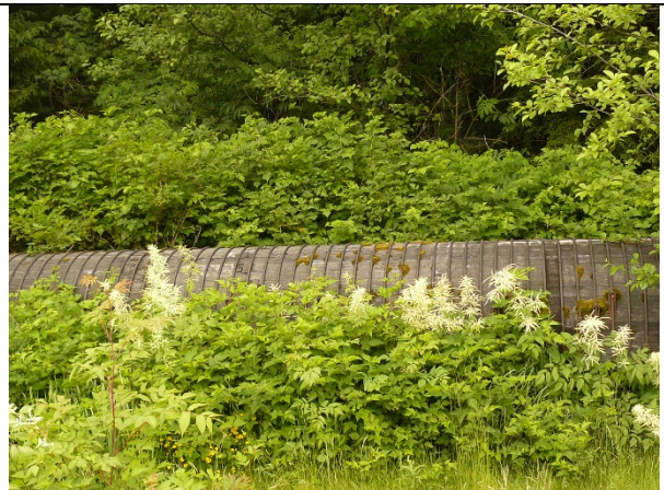
Photo 54. Wood stave pipeline
