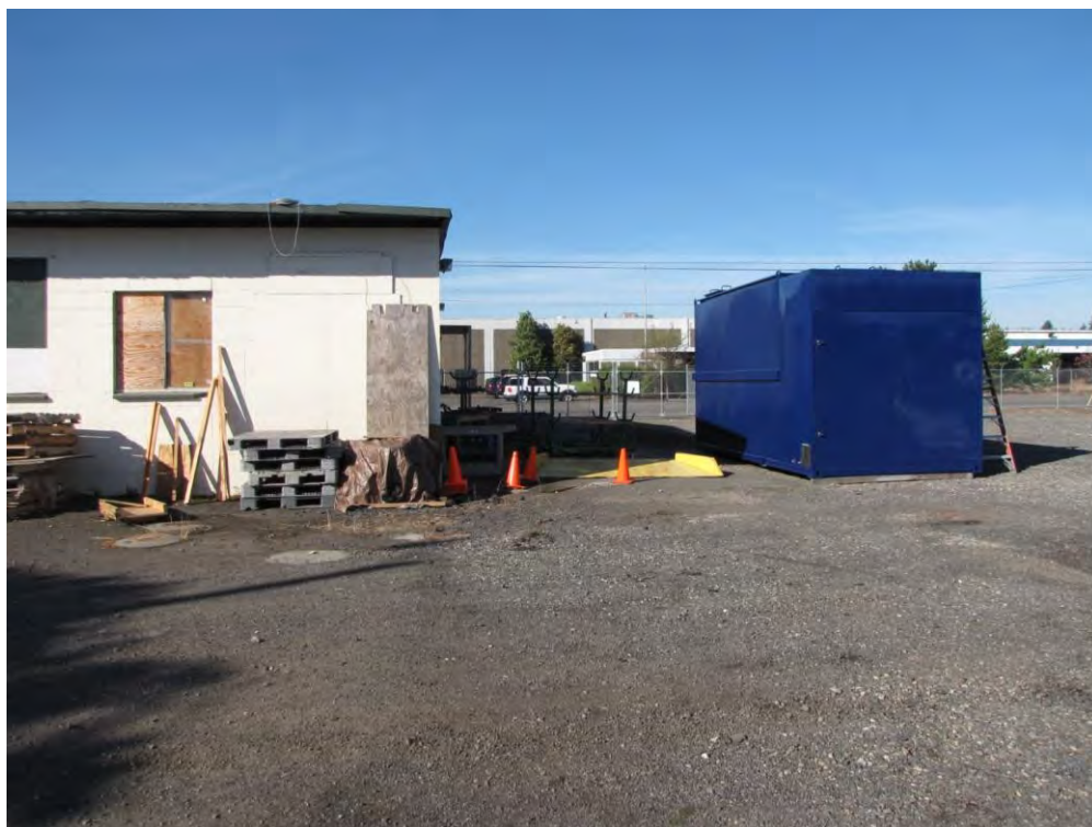
Photo 2. Location of reactive barrier. Monitoring wells RA-IW-4A/B in foreground.
