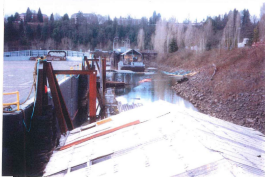
PHOTO 1: View to the west from the main dock platform. The roofed barge in the background is part of the adjacent facility.
