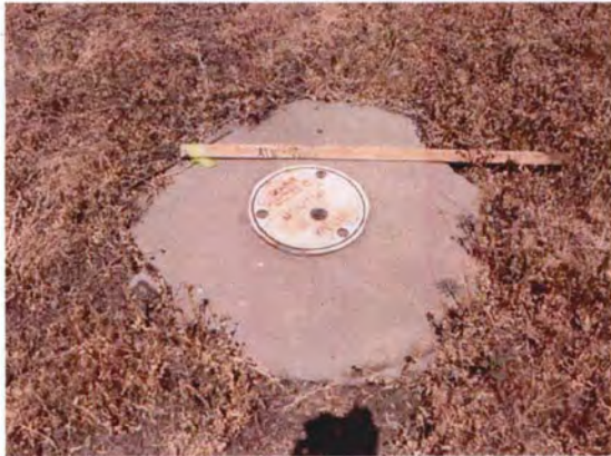
Monitoring well W-7
