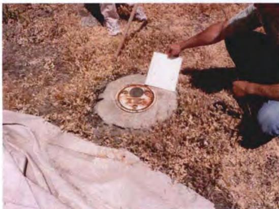
Monitoring well W-17
