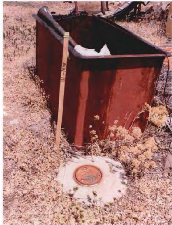
Monitoring well W-16
