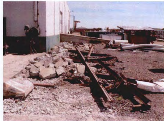
Demolition of old railroad spur looking east towards the southwest corner of Stephens Metal Products warehouse
