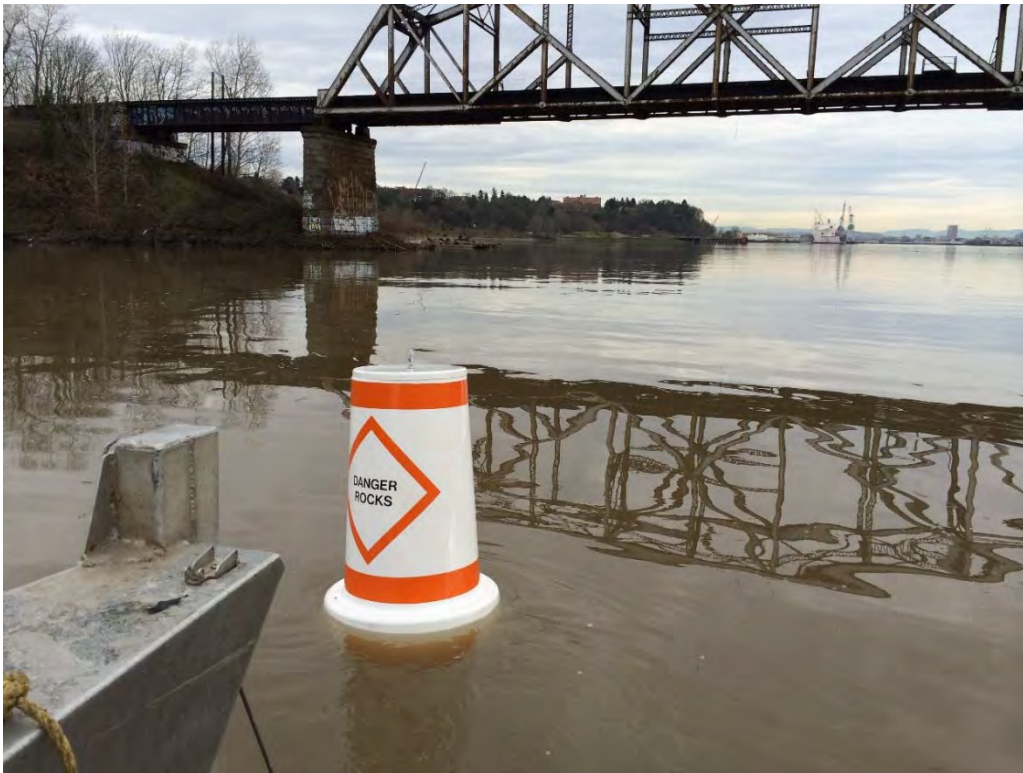
Photograph 3 – Buoy number 4 replacement.
