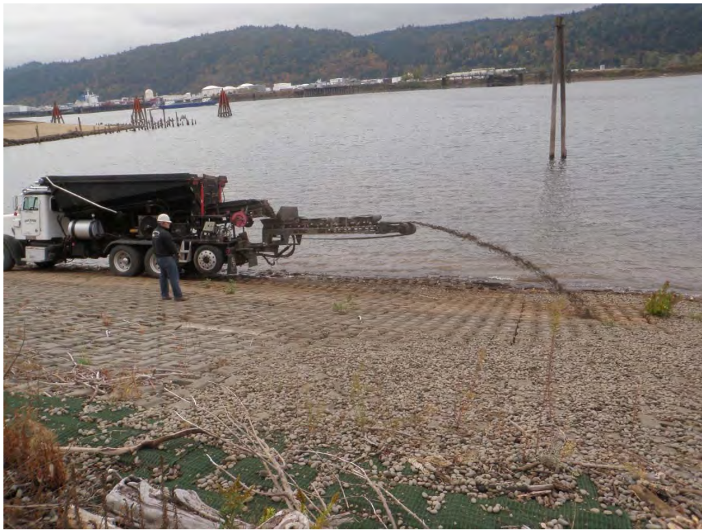
Photograph 10 – ACB gravel replacement in 2012.
