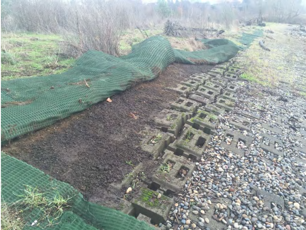
Photograph 4 – Mulch placed beneath TRM during December 2015 shoreline repairs.
