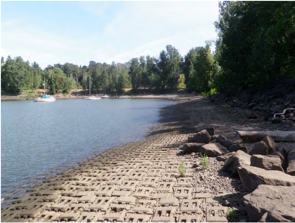
Photograph 2 – Typical habitat gravel within ACB armoring in Willamette Cover.
