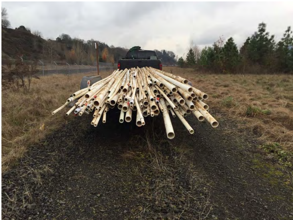
Photograph 11 – 2015 irrigation system decommissioning.
