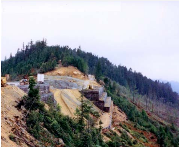
Exhibit 2-4. Crib wall structures on northwest side of Silver Butte ridge
