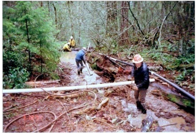
Exhibit 2-2. Hand excavation of tailing and alluvium to a pipe collection system that drains to MXR pond, March 1994
