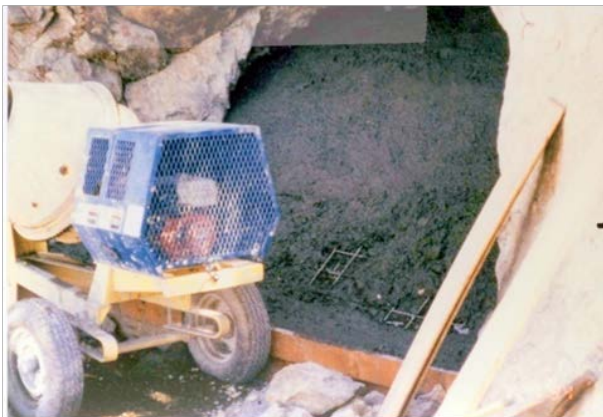
Exhibit 2-3. Closure of an Adit portal with rebar and concrete, July 1994
