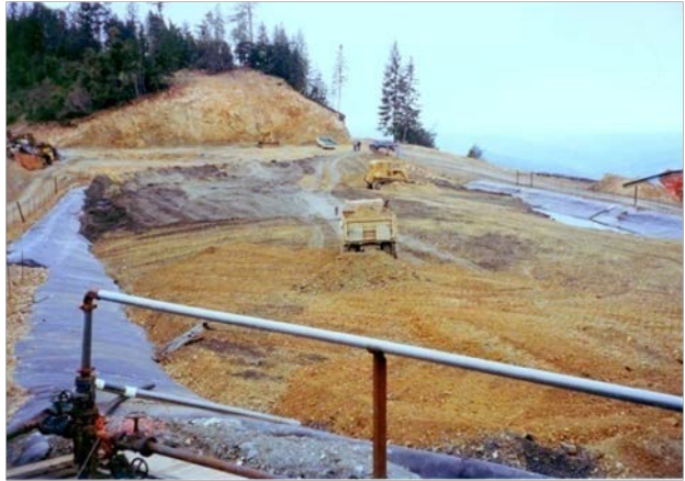
Exhibit 2-5. Backfill of low-grade ore over tailings during encapsulation mound construction, May 1994
