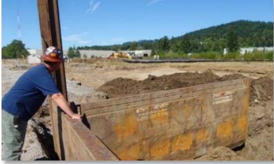
Figure 6. Soil excavation work during the site's final removal action in 2008.
