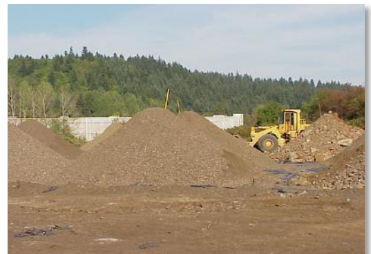
Figure 5. Excavated soil ready for off-site disposal.
