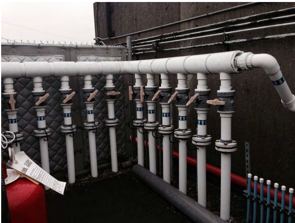
Photo 8. BP Terminal detail for the Soil Vapor Extraction Remediation System showing 11 individual well control valves and piping. Blue airlines to right were installed as a contingency in case additional remedial technologies, such as air sparging, would be needed to meet site cleanup objectives. This system is removing petroleum vapors from soil and groundwater for subsurface cleanup action.
