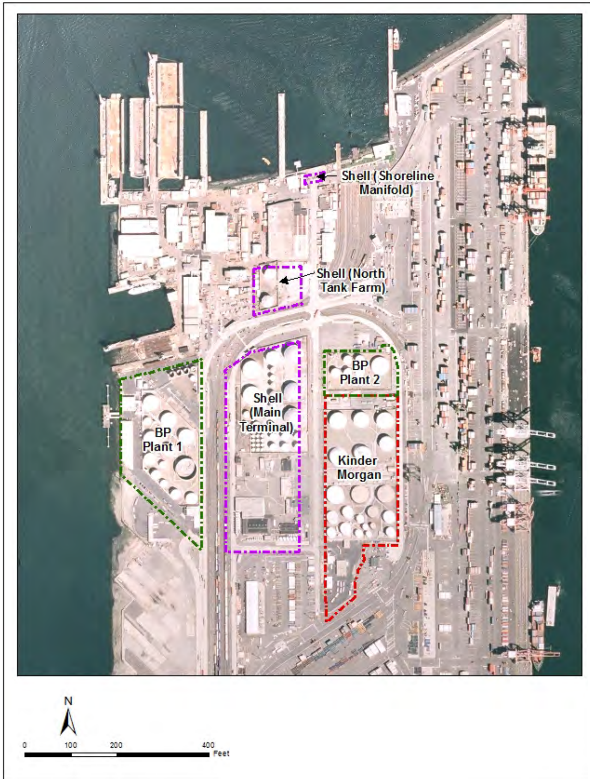
Figure 6. TF-OU2, Tank Farm Facilities
