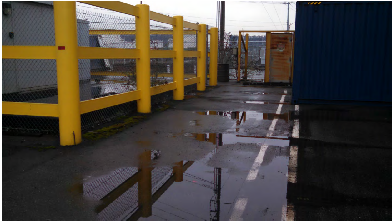
Photo 4. Vegetation growth in capped area
