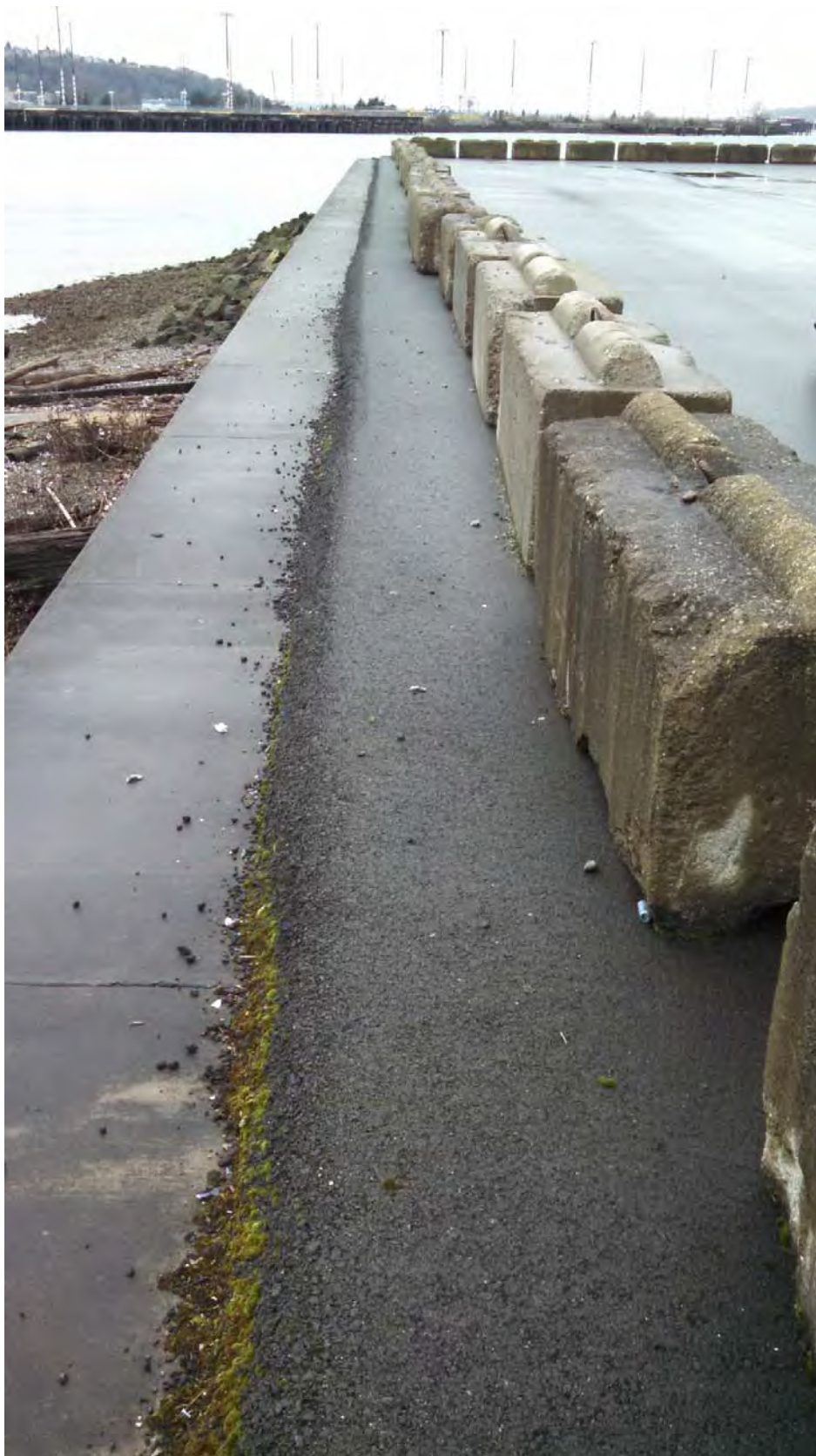
Photo 7. Edge of new asphalt cap
