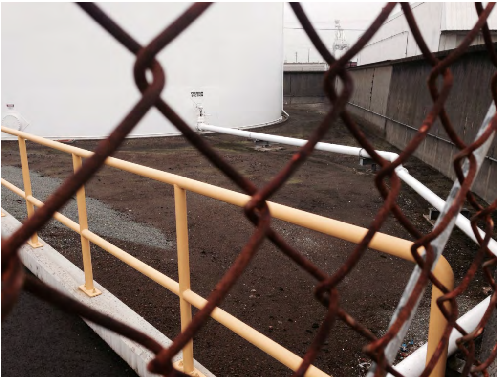
Photo 9. BP Terminal Plant 1 at south wall looking east where above ground storage tank (AST) No. 8 with monitoring well GM-16S is located in distance at the southeast corner of Plant 1.
