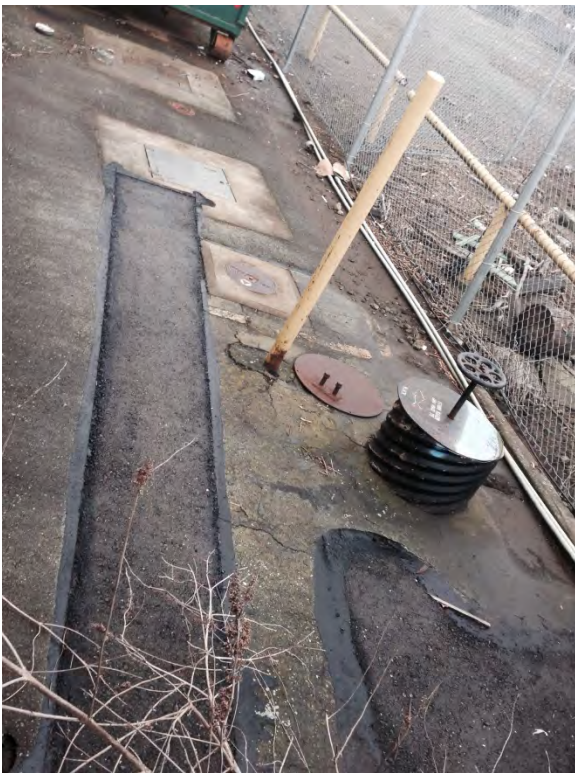
Photo 6. BP Terminal showing Compliance Monitoring Well AMW-01 to the left and behind the yellow bollard. Additionally, Recovery Well RW-10 is located directly behind AMW-01. Recovery Well RW-10 is an active pumping well utilized as part of the Groundwater/LNAPL Recovery System. Well heads are flush mounted to ground surface.
