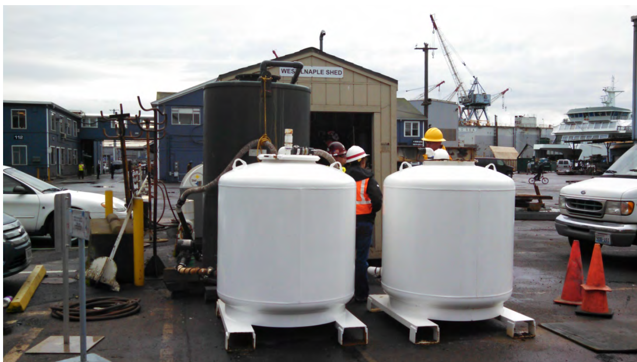
Photo 17. West LNAPL Shed carbon vessels
