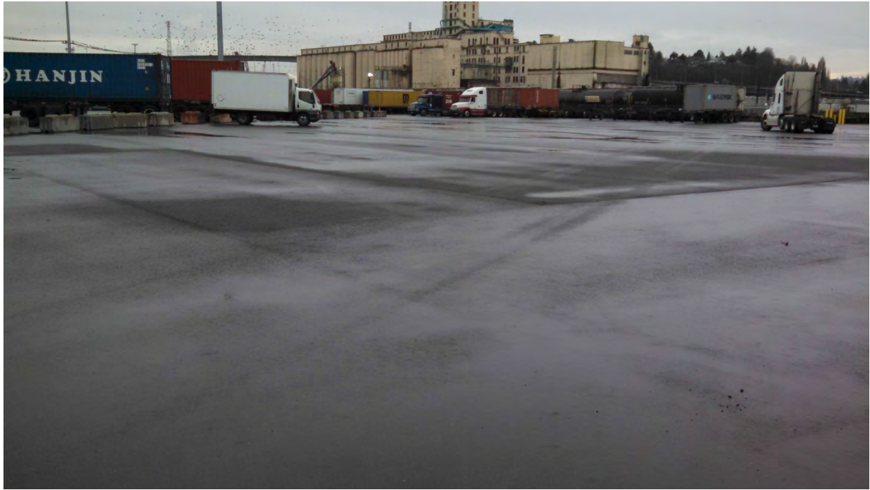
Photo 8. Minimal water ponding after regrading and capping
