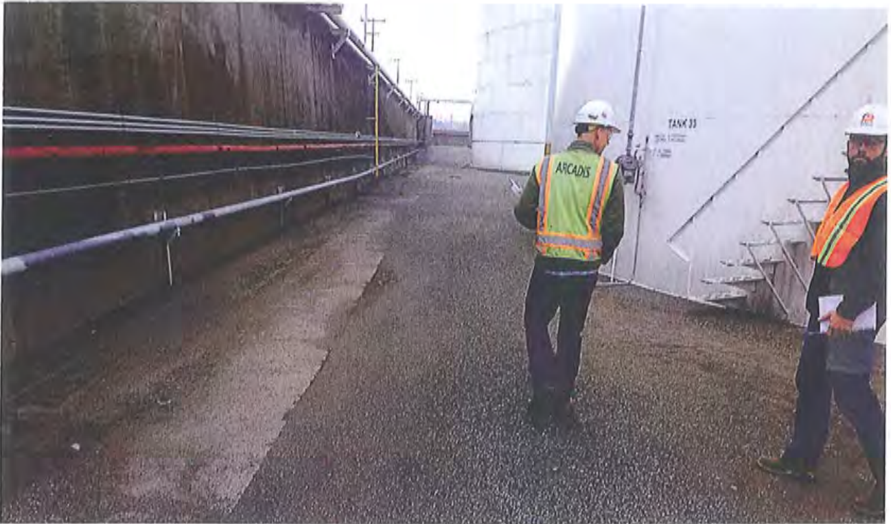
Photo 3. KMLT Above ground petroleum Storage Tank No. 33 at B Yard with containment wall and piping on left with two Arcadis consultants conducting the site inspection.
