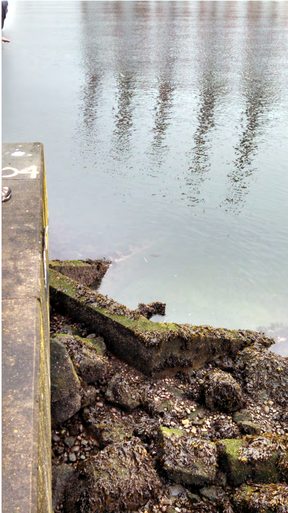
Photo 9. New stormwater outfall
