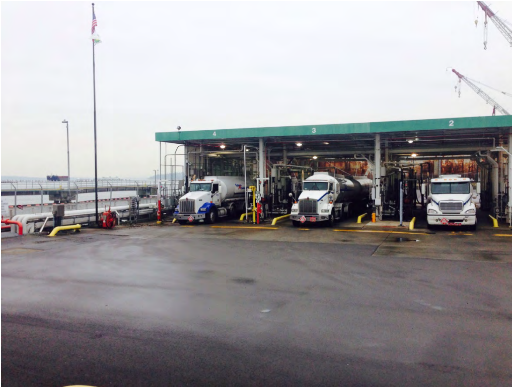
Photo 1. BP Terminal Harbor Island illustrating one petroleum fuels loading rack looking northwest.
