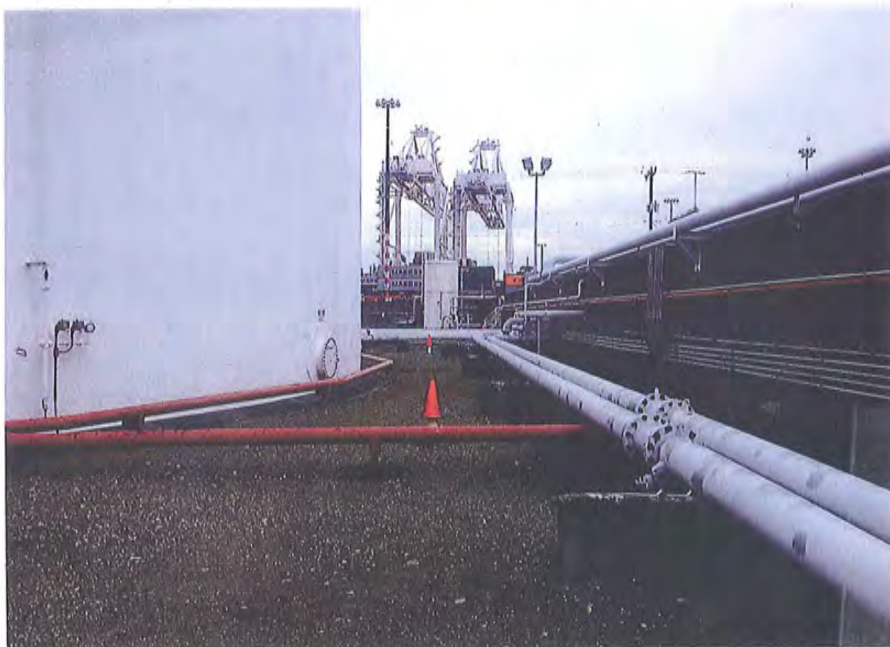
Photo 6. KMLT Above ground petroleum Storage Tank and supply piping with containment wall to right.
