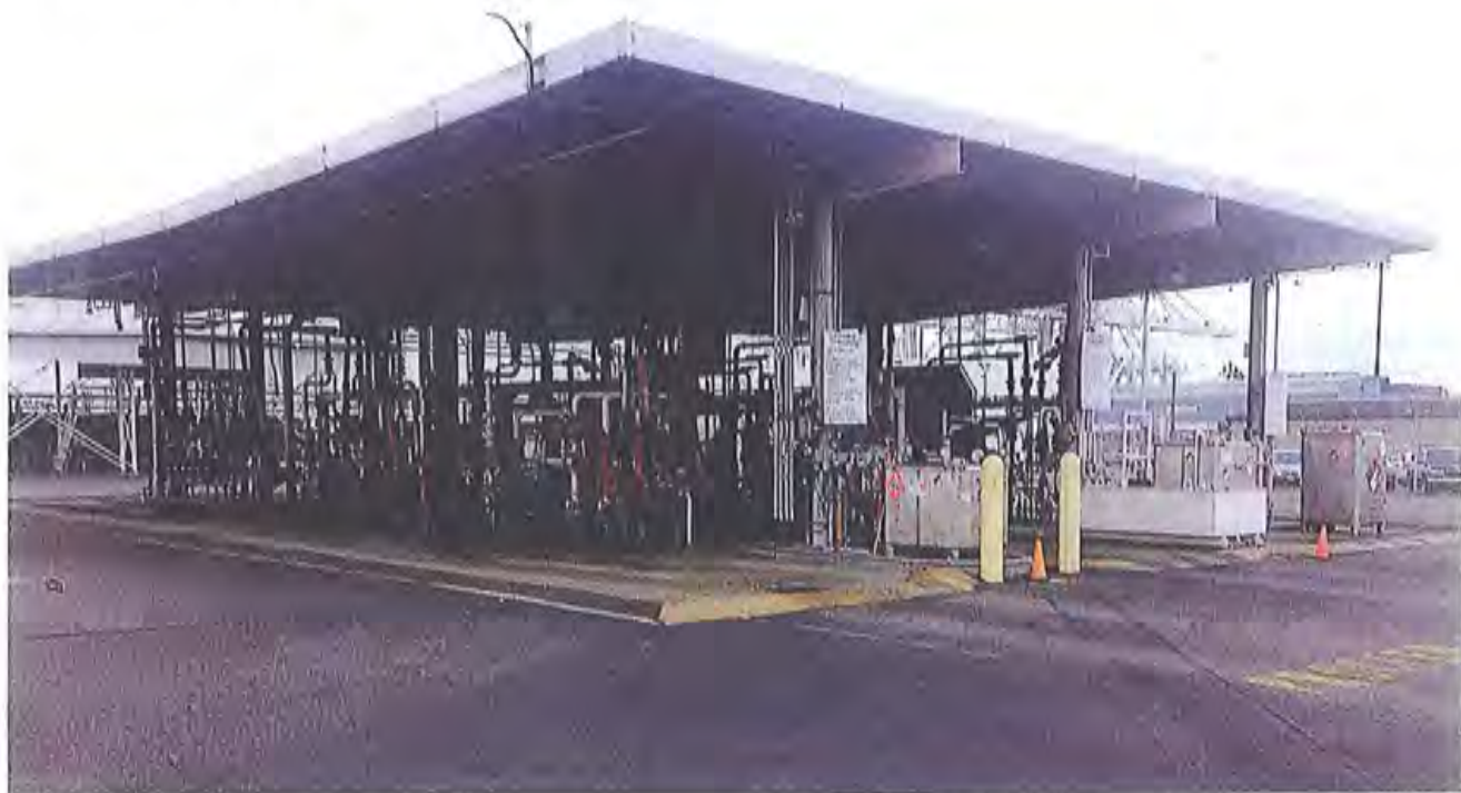
Photo 1. KMLT illustrating a petroleum fuels loading rack.
