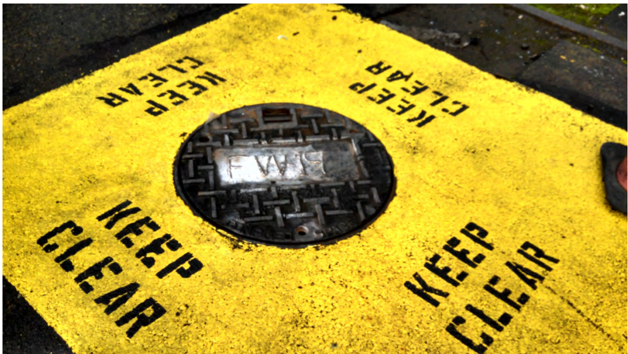
Photo 14. Extraction well FW-19
