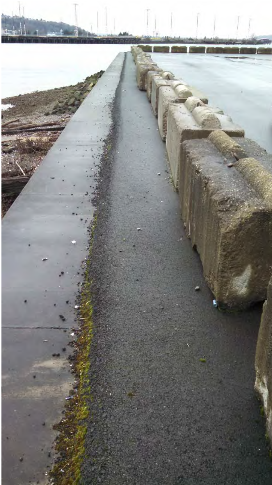
Photo 7. Edge of new asphalt cap
