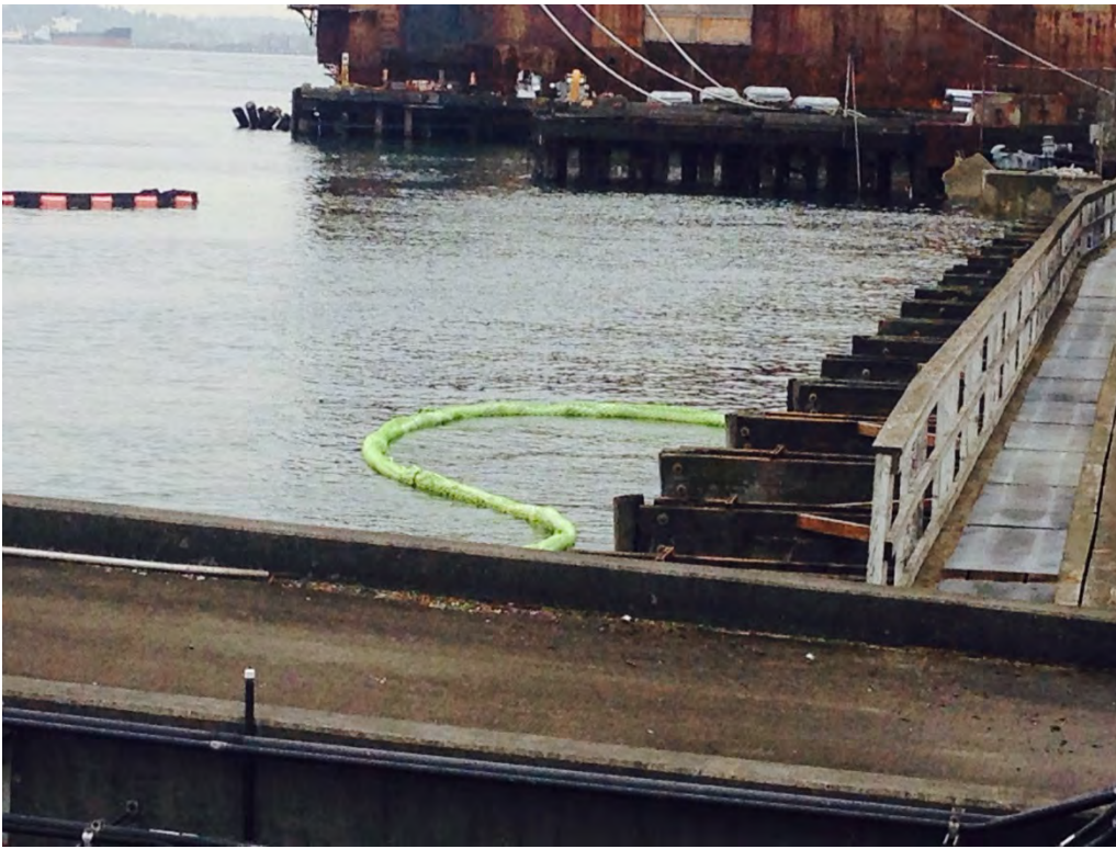
Photo 3. BP Terminal seawall and green boom to capture any sheen or floating product on West Waterway as a safety measure, and photo looking NNW at West Waterway and Elliott Bay in the background.
