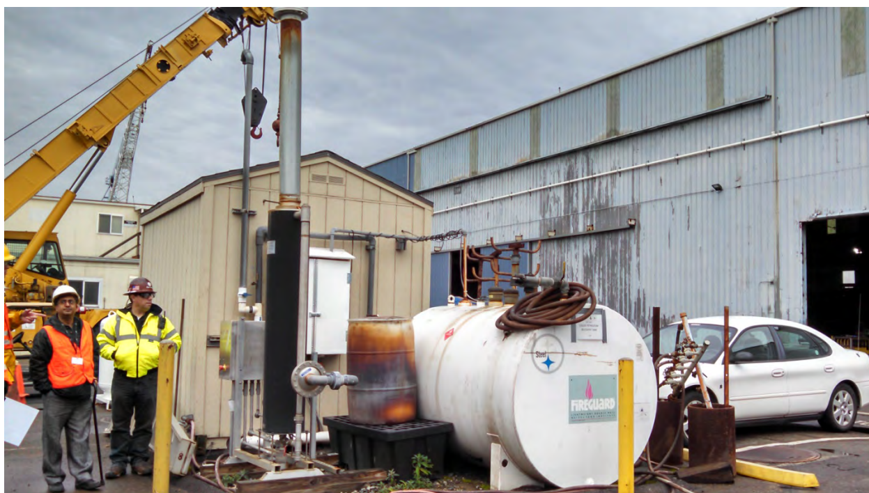
Photo 18. West LNAPL Shed LNAPL tank and catalytic oxidizer
