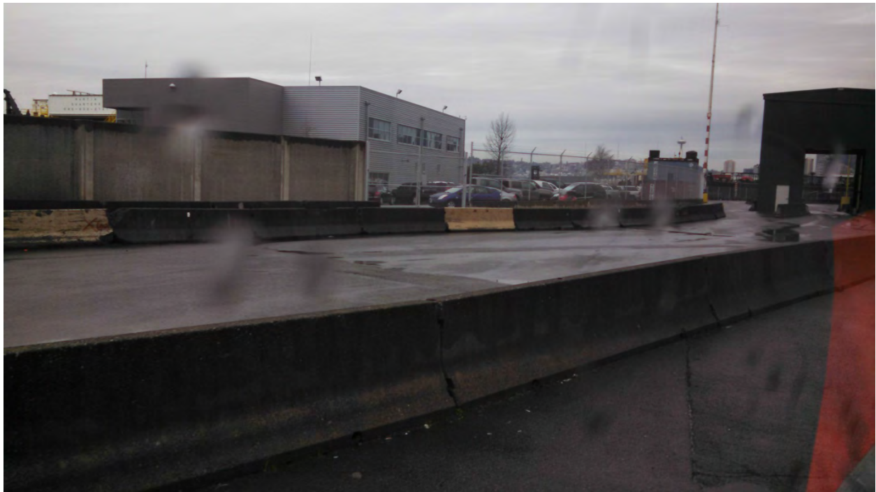
Photo 1. K-rail on the western S&G OU1 cap boundary
