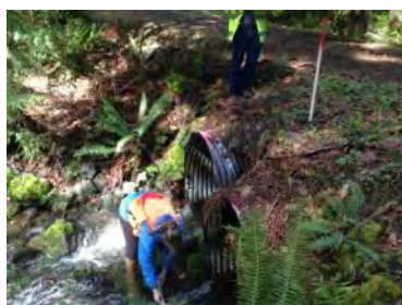
Photos 13 & 14 Culvert 7 outlets
