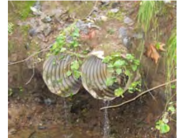
Photo 10 Culvert 3 outlets
