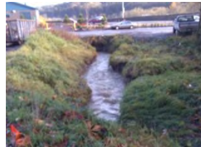
Photo 5 Looking southeast at ditch and 36-inch culvert crossing west of Hwy 3
