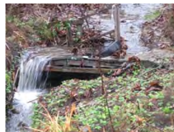
Photo 23 Private Wooden Bridge
