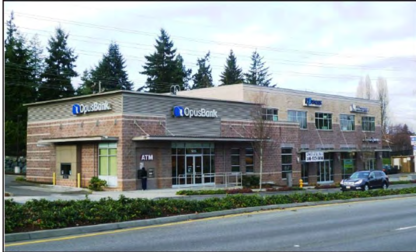
Example of a commercial building.
