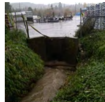
Photo 4 Looking south at 36-inch culvert (in shadow)
