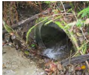
Photo 1 Culvert 1 outlet at south end
