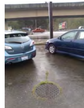
Photo 2 At south culvert end, looking south across SR 16 toward unnamed tributary
