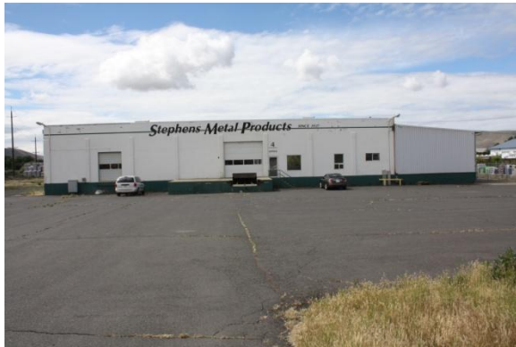
Front of Stephens Metal Products warehouse – parcel address is 4 W. Washington Avenue in Yakima, Washington (business has moved but is about to lease to another light industrial business).
