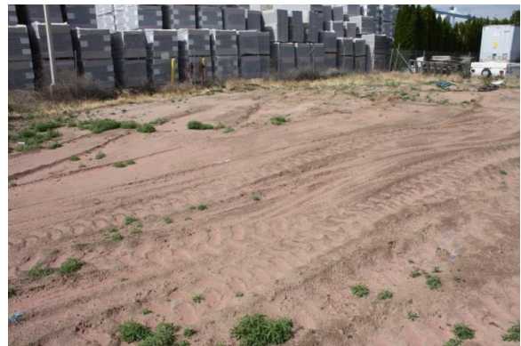
Soil brought in to help grade back part of Stephens Metal Products yard. One of the monitoring wells needed to be uncovered for the fall sampling campaign because it was buried under a couple feet of this material.
