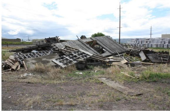
Pile of debris in the yard of the Stephens Metal Products property.
