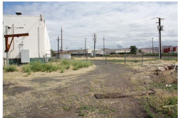
Looking north from the yard at the Stephens Metal Products property. Plume is underneath the location where the photograph was taken and the former pit area is between that position and the warehouse visible in the photograph.
