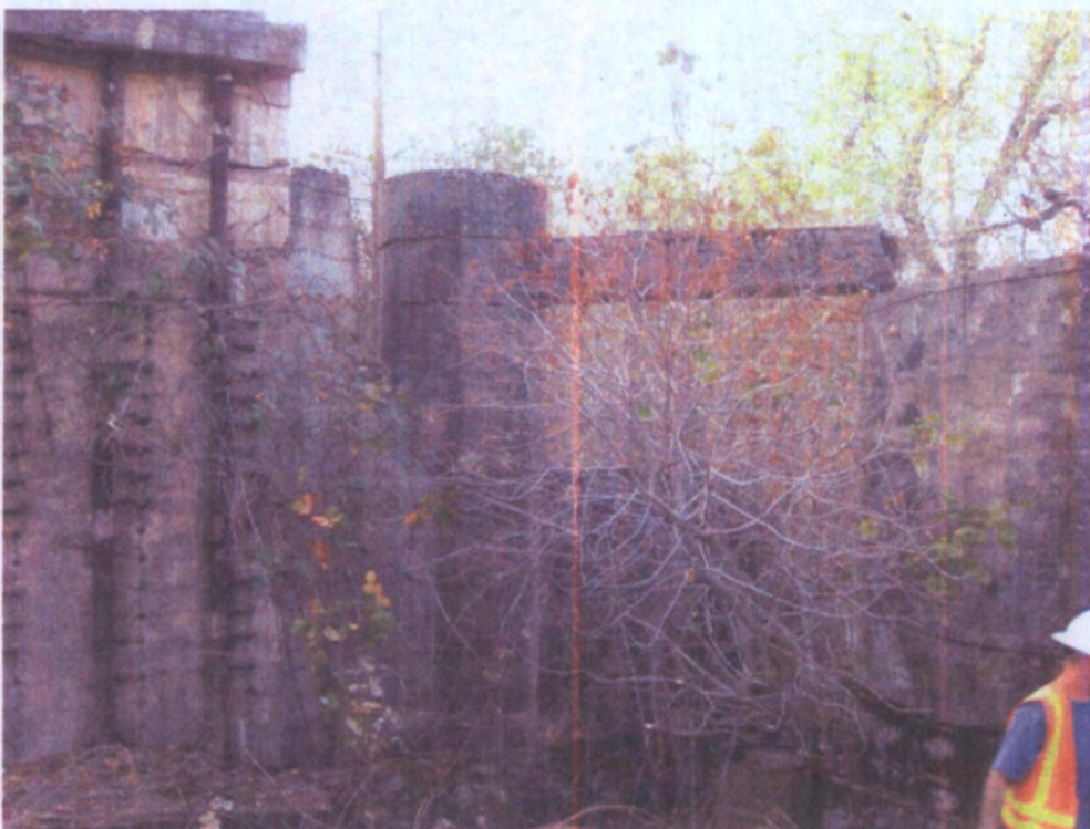
View of cyanide leaching, mixing and flotation tanks at the former cyanide plant
