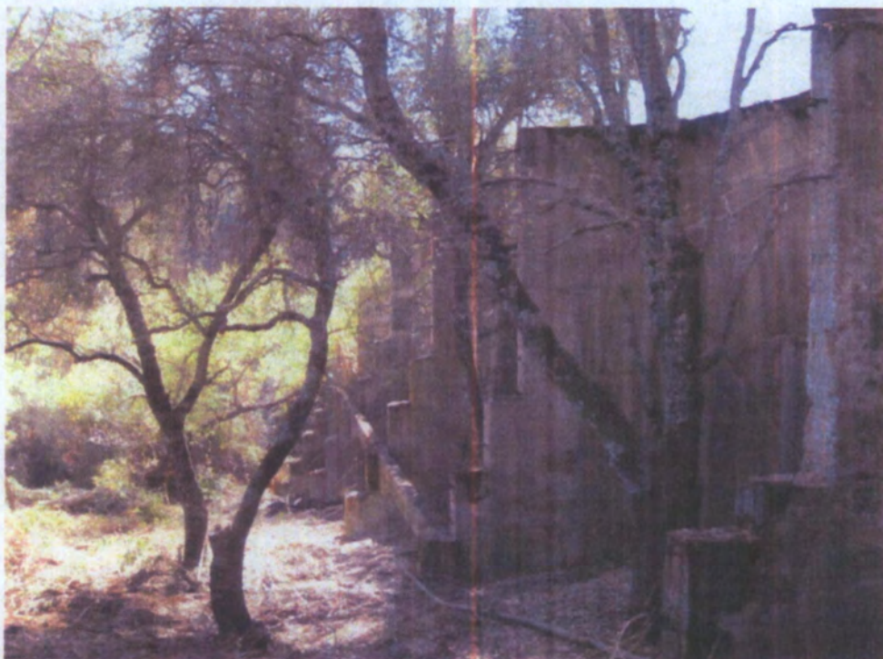
View of the Eastwood Multiple Arch Dam facing south. The dam was built in 1916 and is approximately 46 feet high and 420 feet long with 13 inverted arches.
