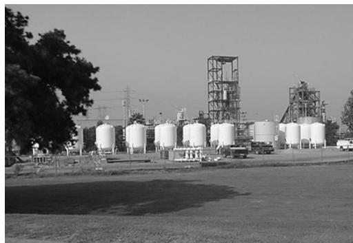
EPA has entered into an agreement with the City of Whittier (City) to operate and maintain the treatment facility. The system is designed to pump and treat 16 mgd of contaminated water. In 2005, the City began providing clean treated water from the intermediate zone potable water supply. The treated water from the shallow zone is discharged into Legg Lakes.
