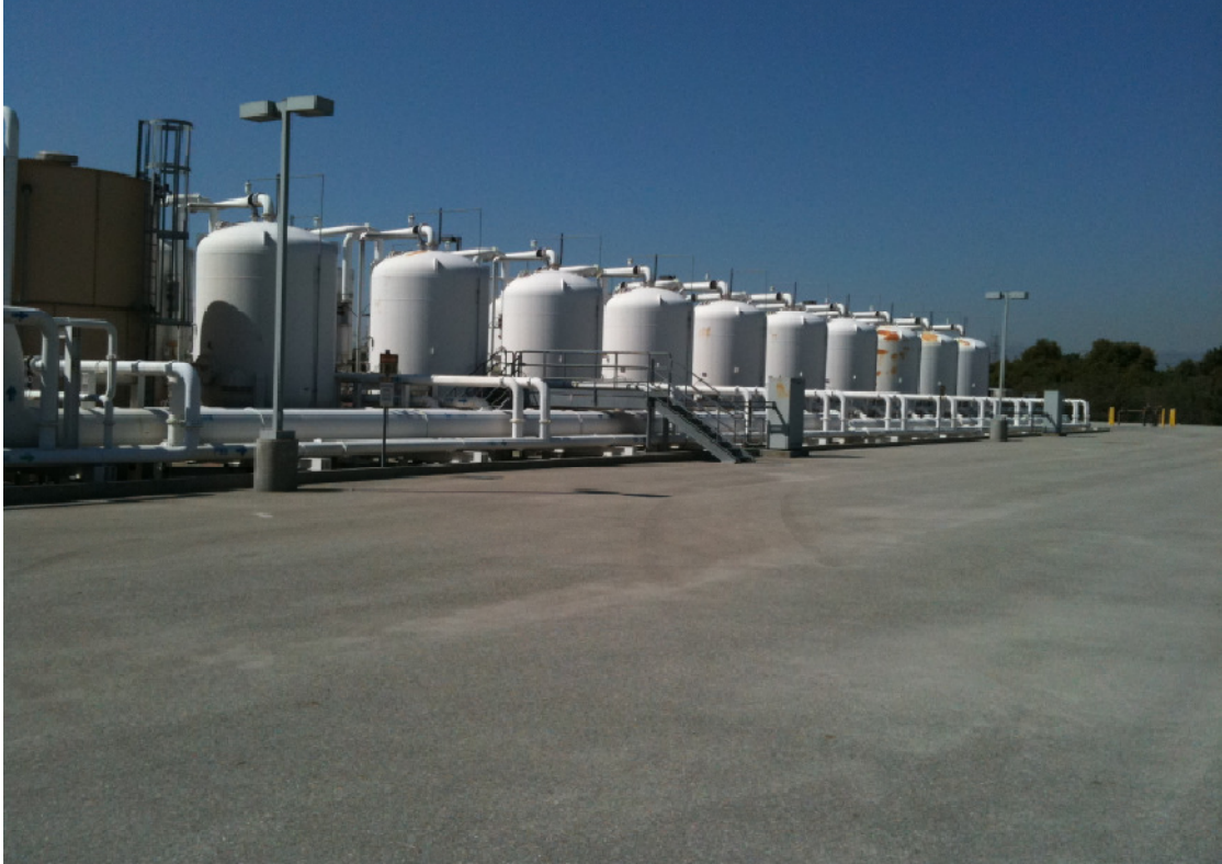
Photo 7: Treatment Plant Carbon Vessels – Back Half
