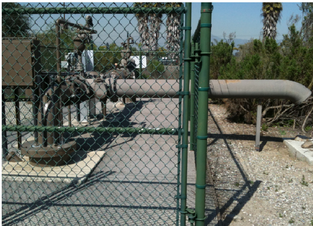
Photo 4: EW4-7 Wellhead (and flushline)
