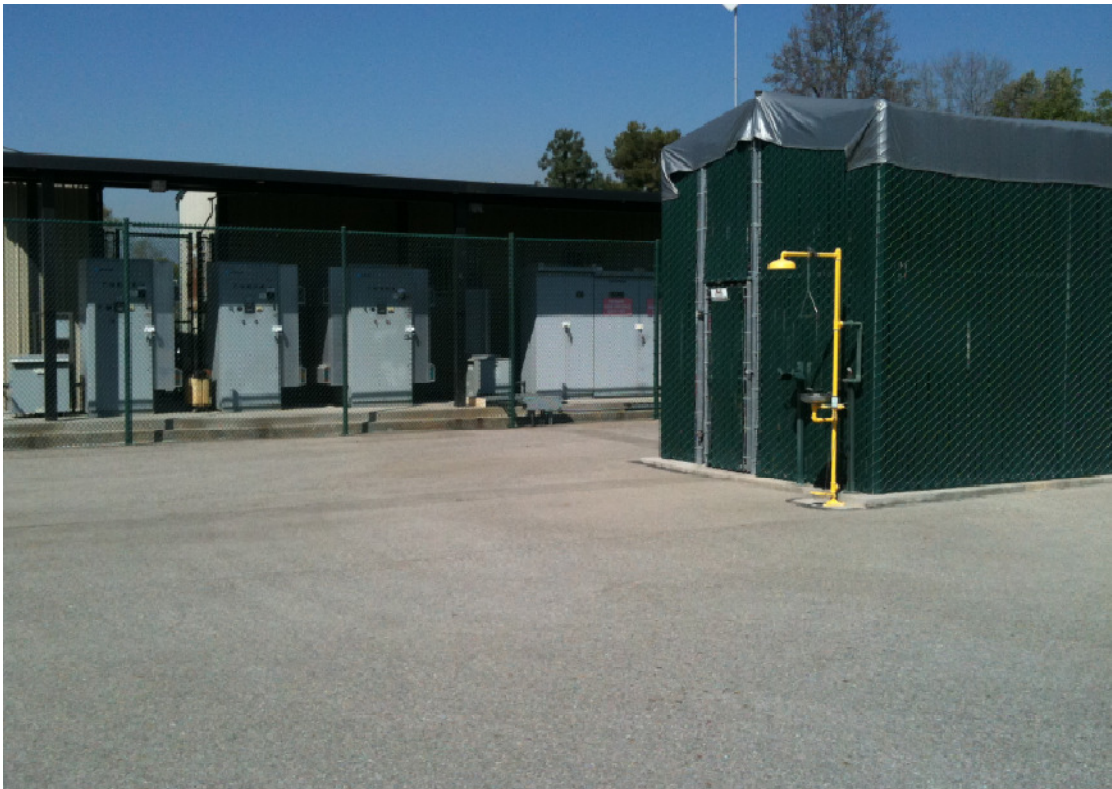
Photo 10: Disinfection System and Treatment Plant VFDs
