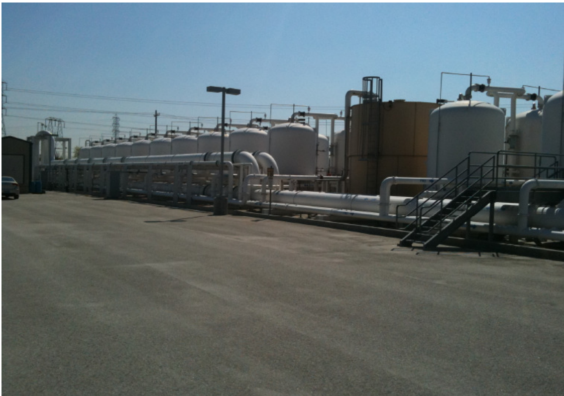
Photo 6: Treatment Plant Carbon Vessels – Front Half
