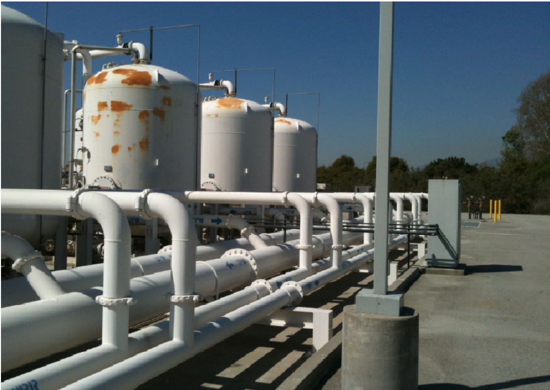
Photo 8: Close-up on Carbon Vessels Showing Need for Painting
