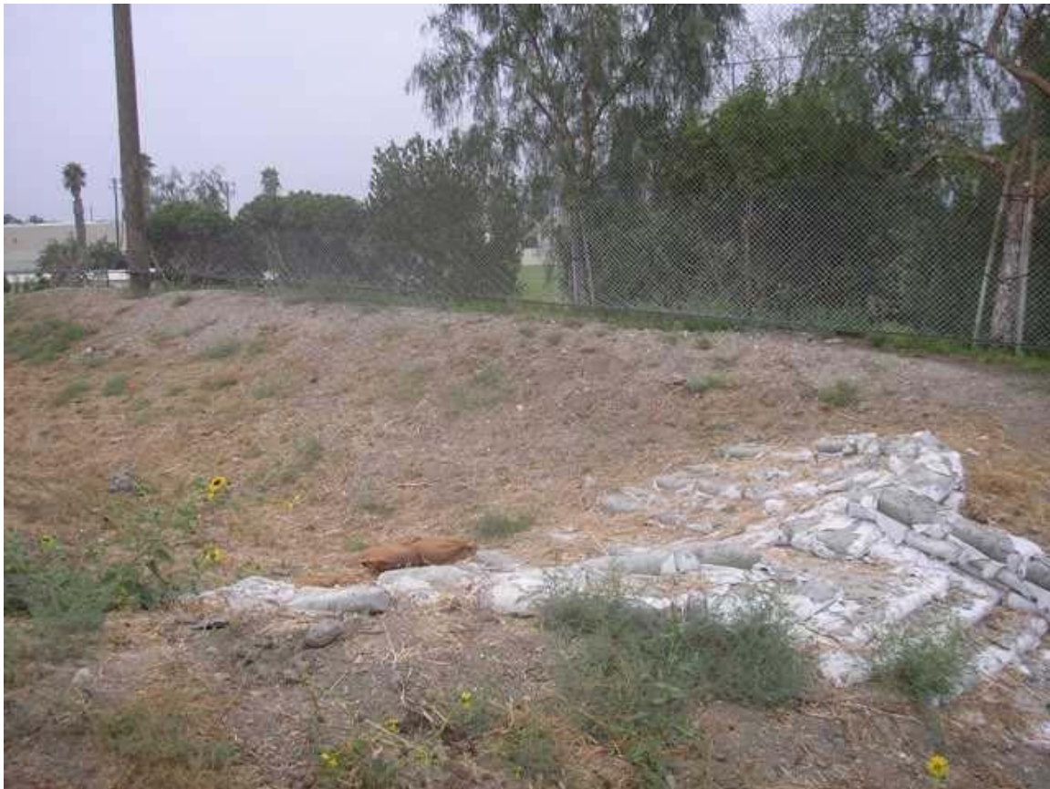
Photo 6: Storm Water Catch Basin, Northeast Area of Site
