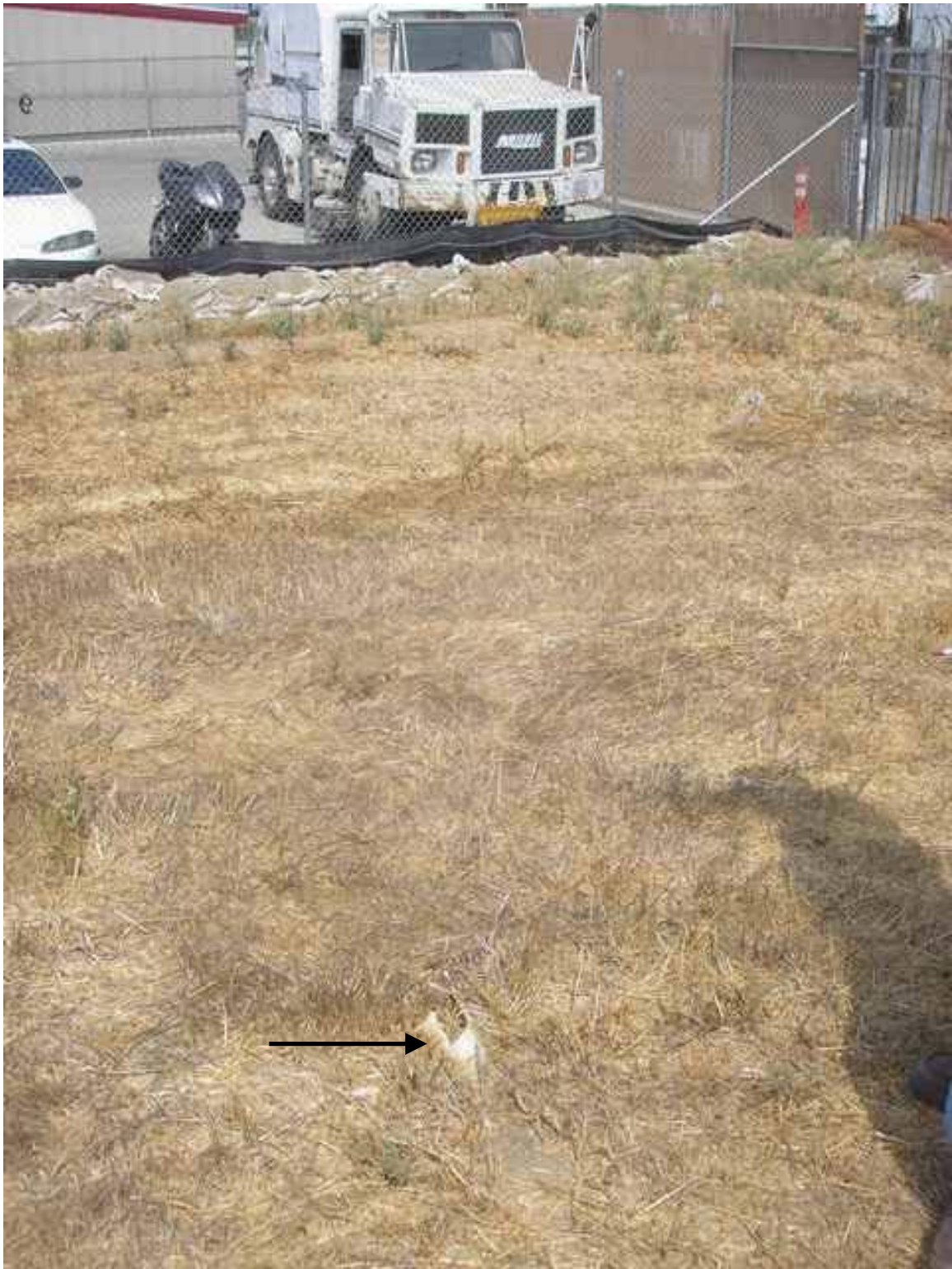
Photo 10: French Drain Outlet, West Side of Site
