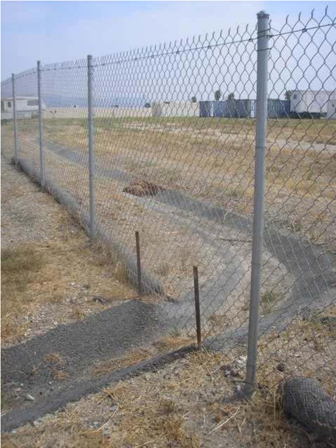
Photo 11: Storm Water Control – V-gutter, West Side of Site
