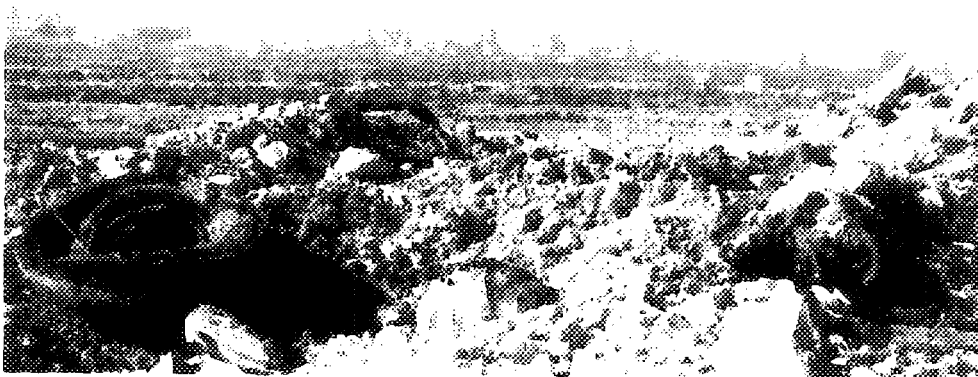
SW-6 WEST SIDE OF DRAINAGE CHANNEL AT TOP OF SIDE SLOPE, LOOKING WEST ACROSS SOUTHEAST CORNER OF UPPER LANDFILL - exposed trash in regraded area
