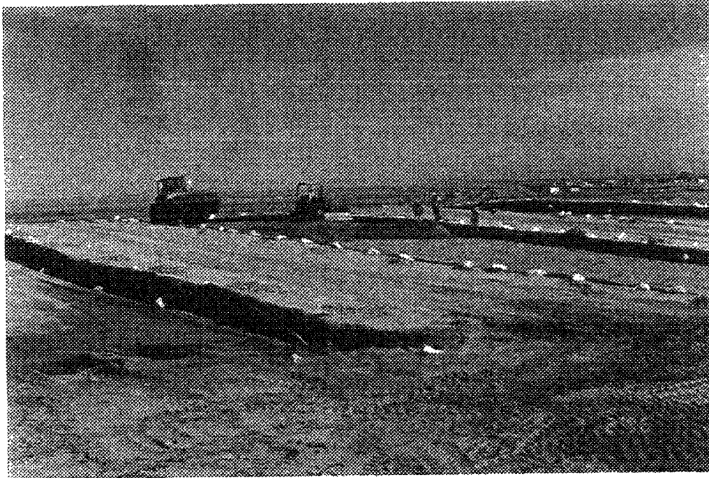
Figure 9. Capillary Barrier Installation
