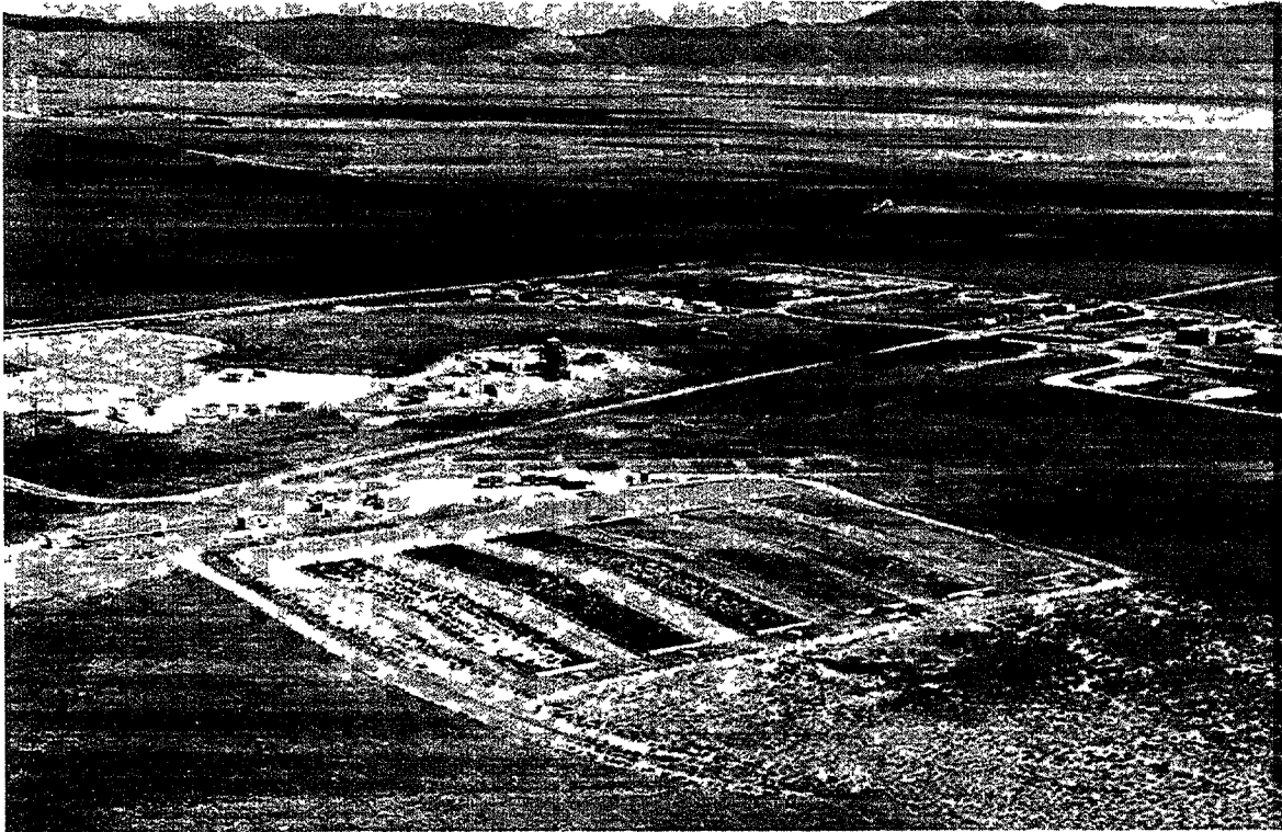
Figure 1. Aerial View of Alternative Landfill Cover Demonstration
