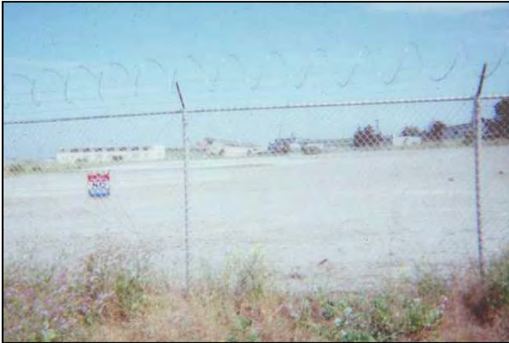
Photograph D-30. Permanent fence along west property line, with no trespassing sign and barbed wire.
