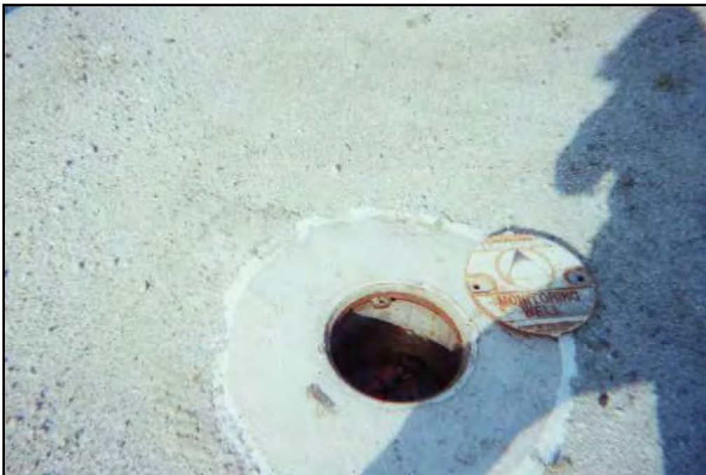
Photograph D-20. Well IR26MW46A; padlock on well and standing water in vault.
