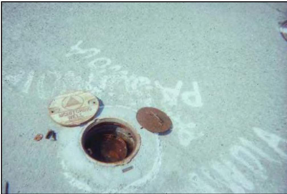
Photograph D-25. Well PA50MW01A; padlock on well and standing water in vault above wellhead.
