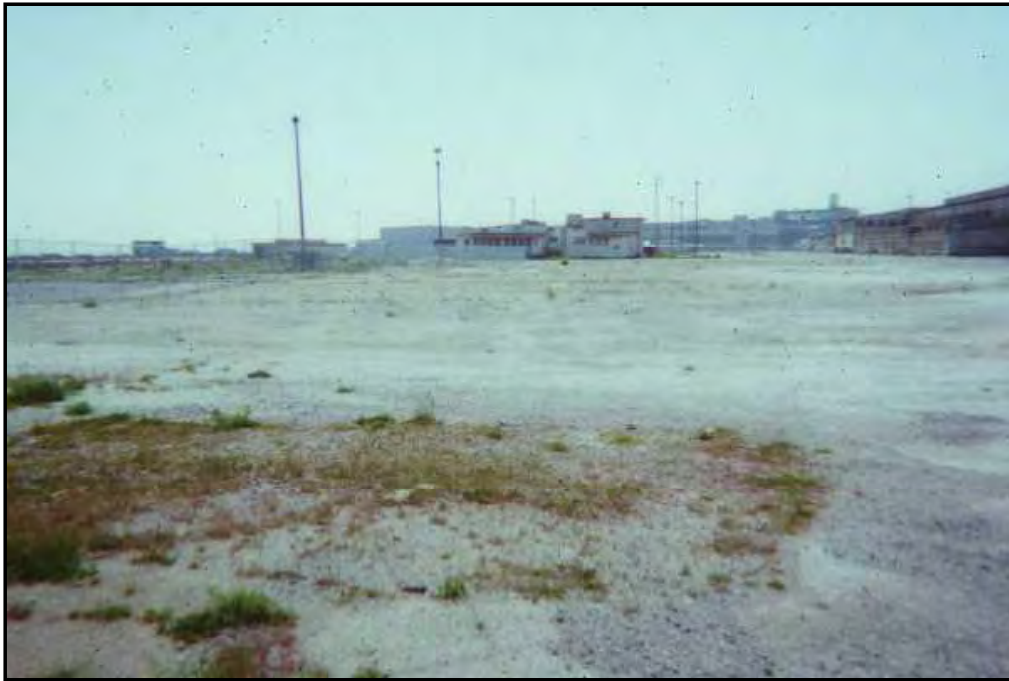
Photograph D-27. Newly installed permanent fence along shoreline new Dry Docks 5, 6, and 7. The fence runs perpendicular to the shoreline between Buildings 125 and 128.
