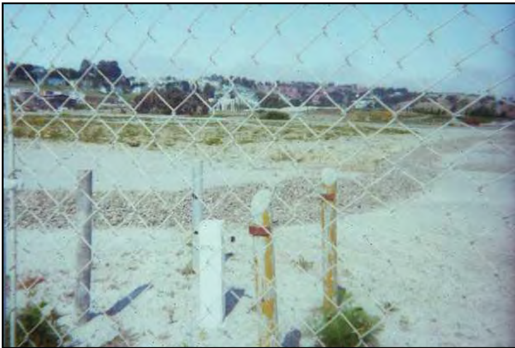
Photograph D-8. Well IR07MWS-2; wellhead is above ground and protected by well casing and concrete bollards.
