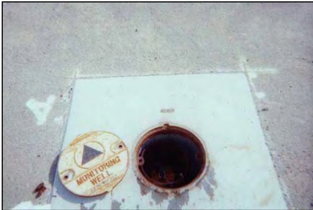
Photograph D-2. Well IR06MW45A; padlock on well and new concrete associated with vault.
