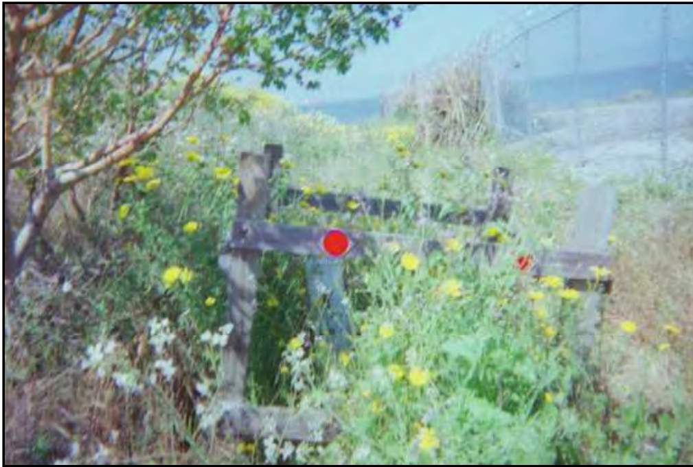
Photograph D-7. Well IR07MW28A; wellhead is above ground and protected by well casing and wooden fencing with reflectors.
