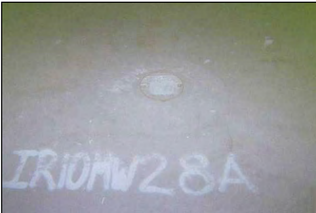
Photograph D-12. Well IR10MW28A; located inside Building 123. Orientation: South Date: May 13, 2003
