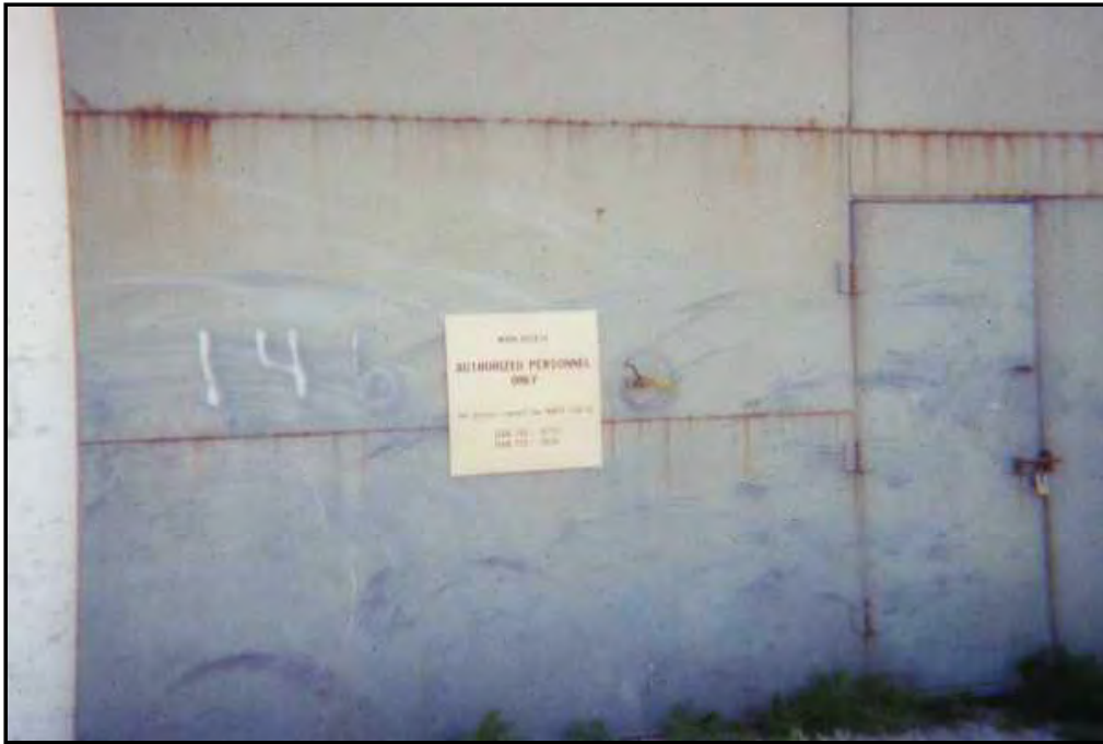
Photograph D-29. Access restriction sign posted on Building 146; representative of signs posted on abandoned buildings throughout Parcel B.
