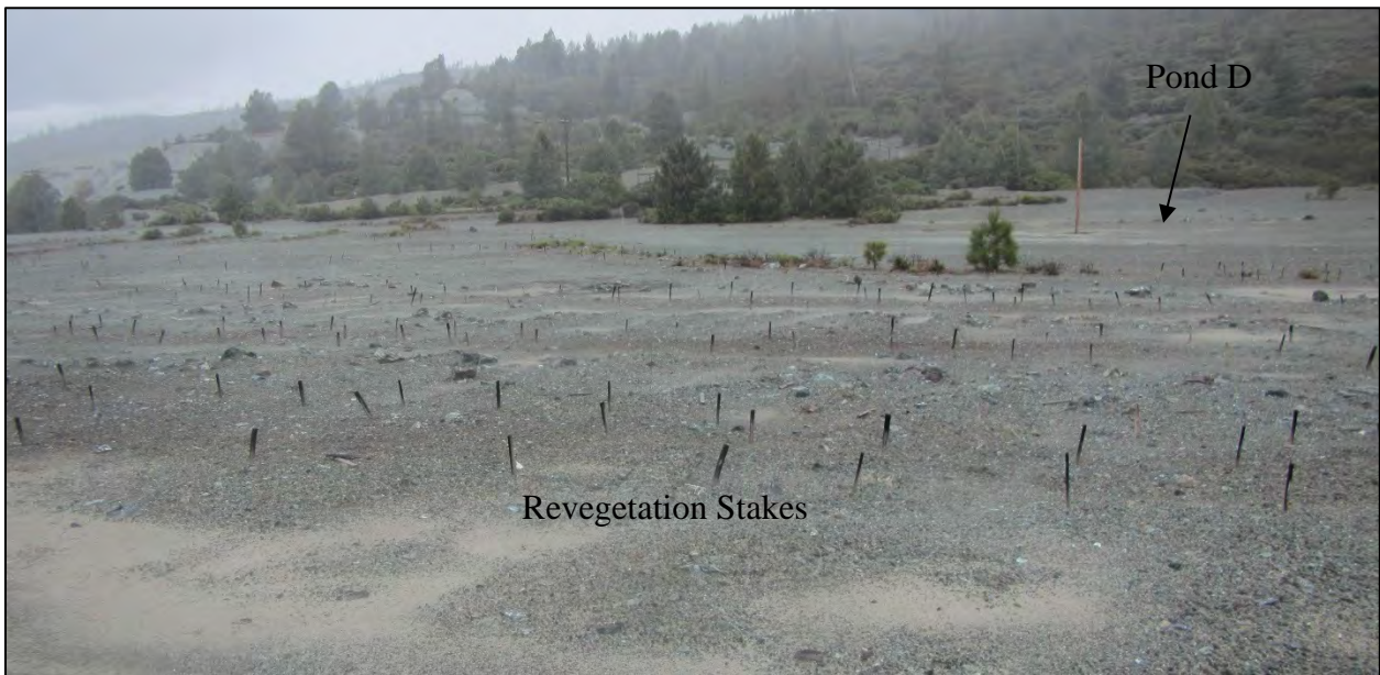
Photo 17. Atlas Pond D and Nearby Failed Revegetation.
