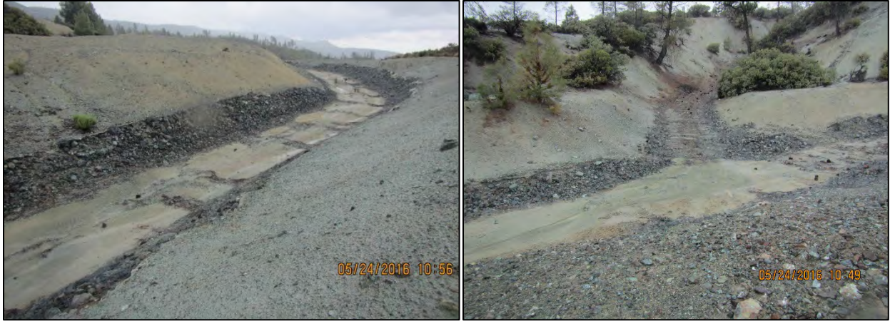
Photo 11. Sedimentation in Atlas Channel A.
