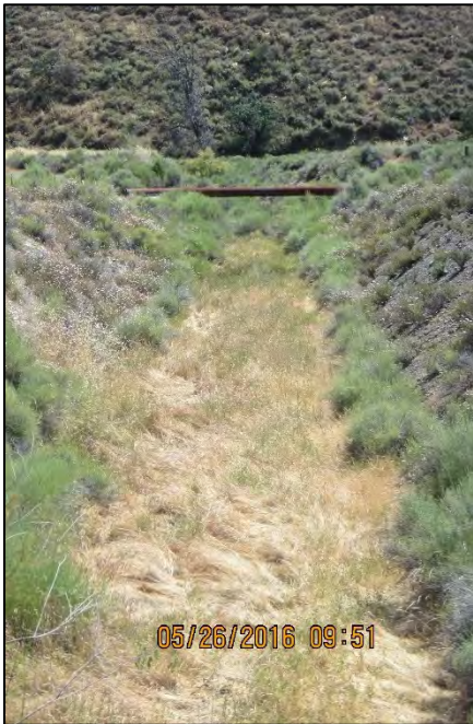
Photo 47. JMM Cross-Canyon Stream Diversion Channel.
