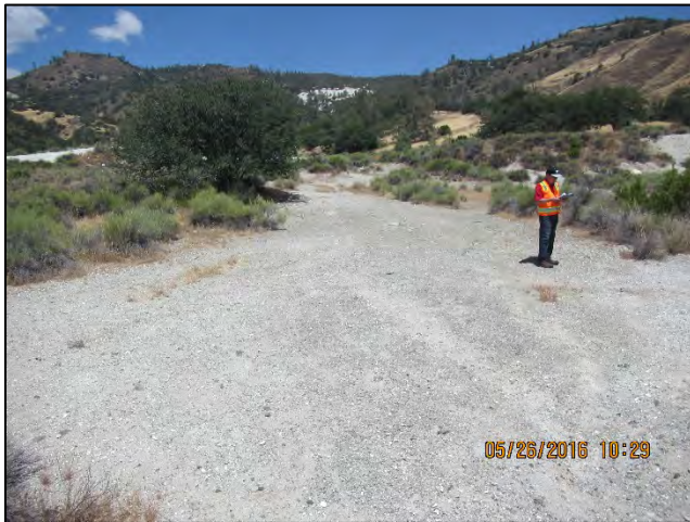
Photo 51. Former Road at JMM.
