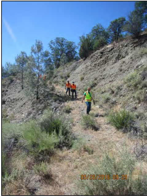
Photo 39. Trail to JMM Sediment Trapping Dam.
