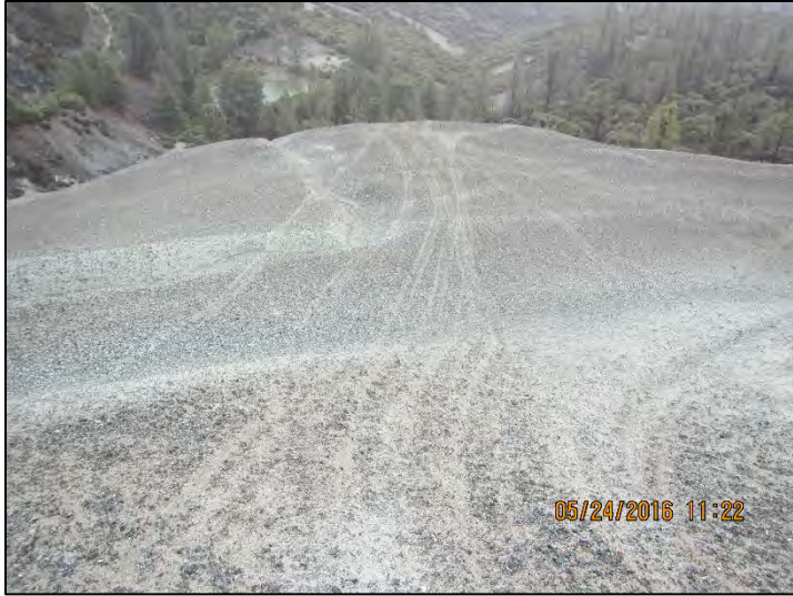
Photo 14. Tire Tracks at South Slope of Atlas Sediment Storage Area.
