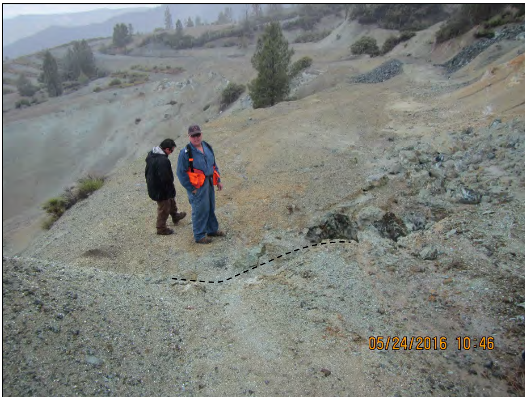
Photo 10. Active Landslide along Road to Atlas Rover Pit; ~4 foot drop.
