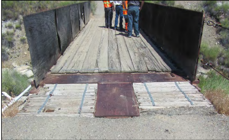
Photo 49. Bridge across Stream Diversion at JMM.
