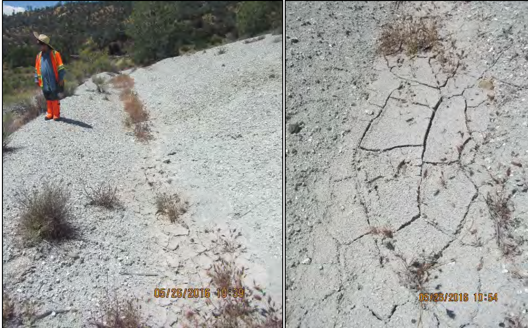
Photo 54. Sediment Collected in JMM Tailings Pile Slope Benches.
