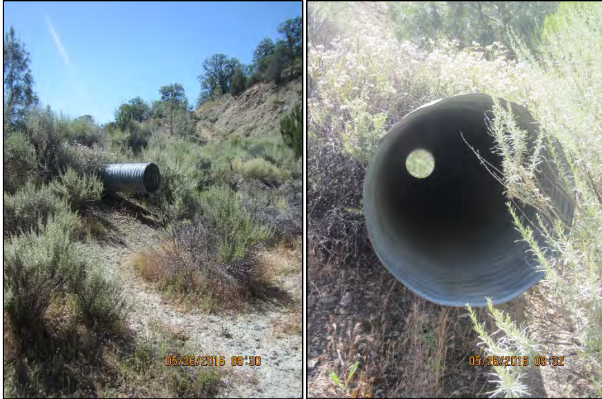
Photo 41. JMM Sediment Trapping Dam Outlet.
