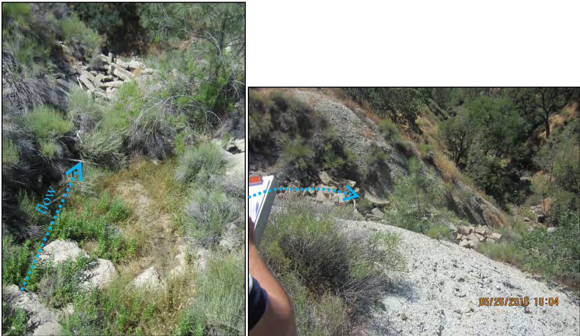
Photo 48. JMM Cross-Canyon Stream Diversion Outlet.
