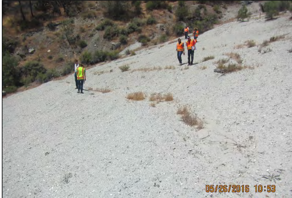
Photo 53. JMM Tailings Pile Slope.
