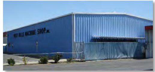
Figure 10. West Hill Machine Shop.
