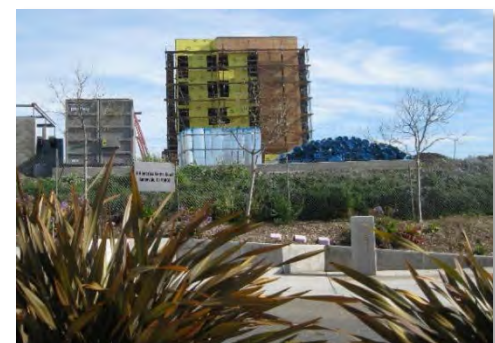
Figure 11. Hotel construction underway at America Center.
