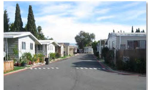
Figure 4. Summerset Mobile Estates is located on part of the former Santos Landfill.
