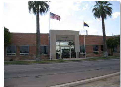
Figure 12. Commercial and light industrial businesses located at 1300 South Litchfield
