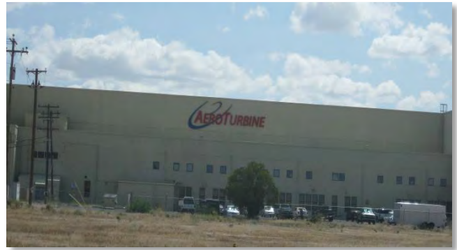
Figure 11. The Aeroturbine facility at PGA-South.
