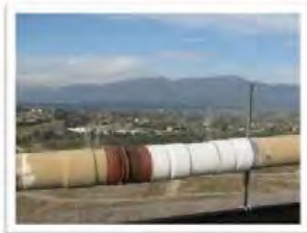
PVC Gas Conveyance line (typical joint repair)
