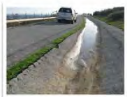
Stormwater ponding in 540N concrete gutter
