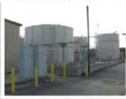
Secondary Containment for the LTP
