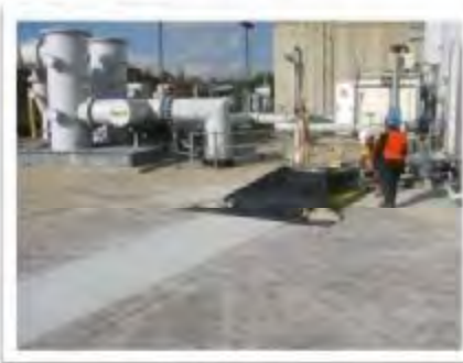
New concrete valve housing the HDPE connection
