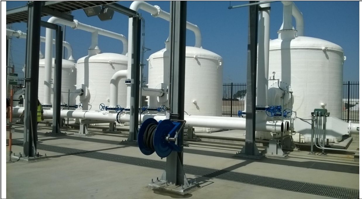
Photo 13. Vapor Granular Activated Carbon Vessels.
