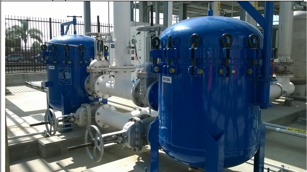
Photo 6. Bag filters prior to HiPOX reactor
