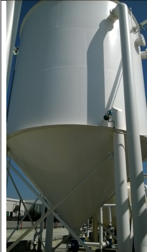
Photo 15. Cone bottom tank used to collect process water which is pumped to first equalization tank at the beginning of the process.
