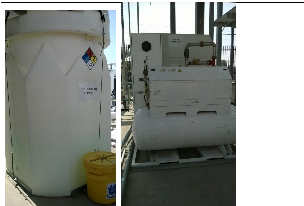
Photo 7. Hydrogen peroxide and the ozone generator for HiPOX Reactor
