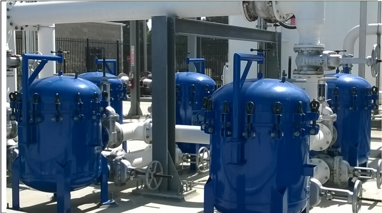
Photo 17. Bag filters before effluent tank
