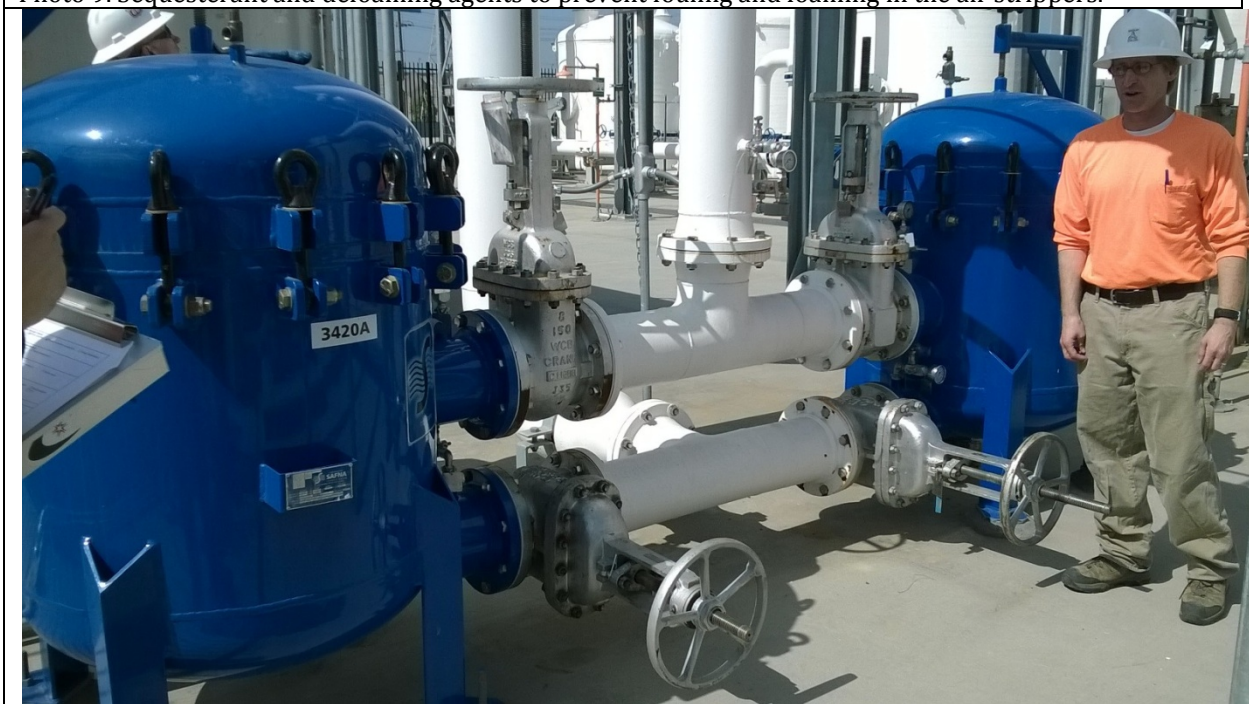
Photo 10. Bag filters before the air strippers.
