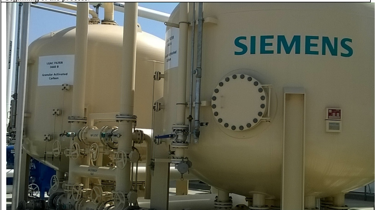
Photo 16. Liquid Granular Activated Carbon Vessels
