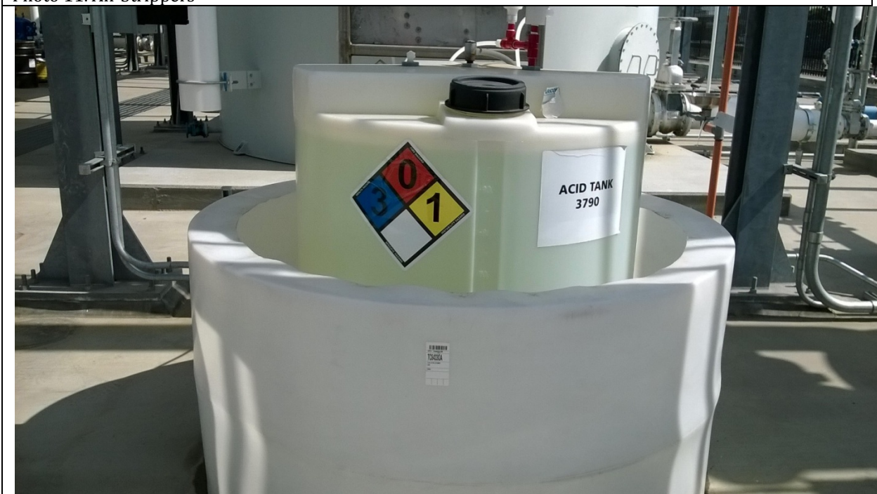
Photo 12. Acid to drop the pH of the treated water prior to the LGAC system
