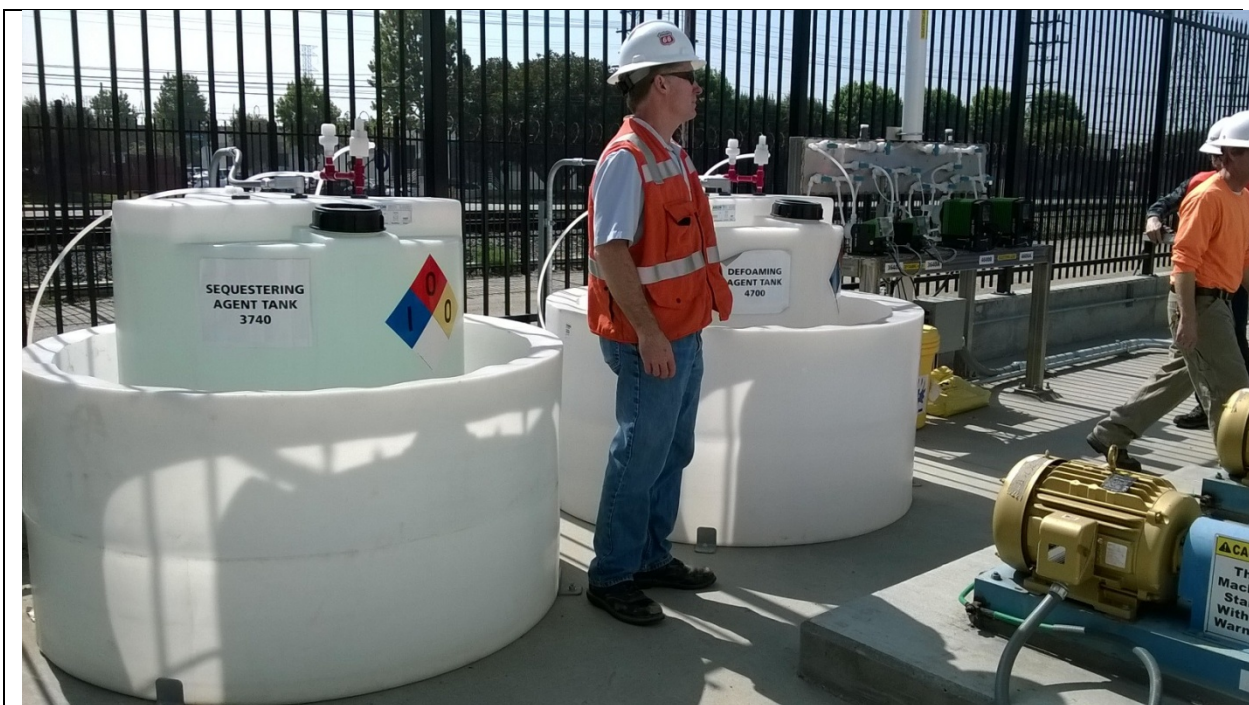
Photo 9. Sequesterant and defoaming agents to prevent fouling and foaming in the air strippers.
