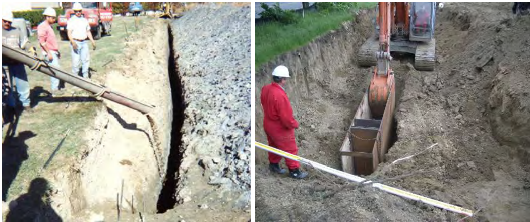
Figure 6-2. Unsupported excavation (left) and temporary trench box (right).
