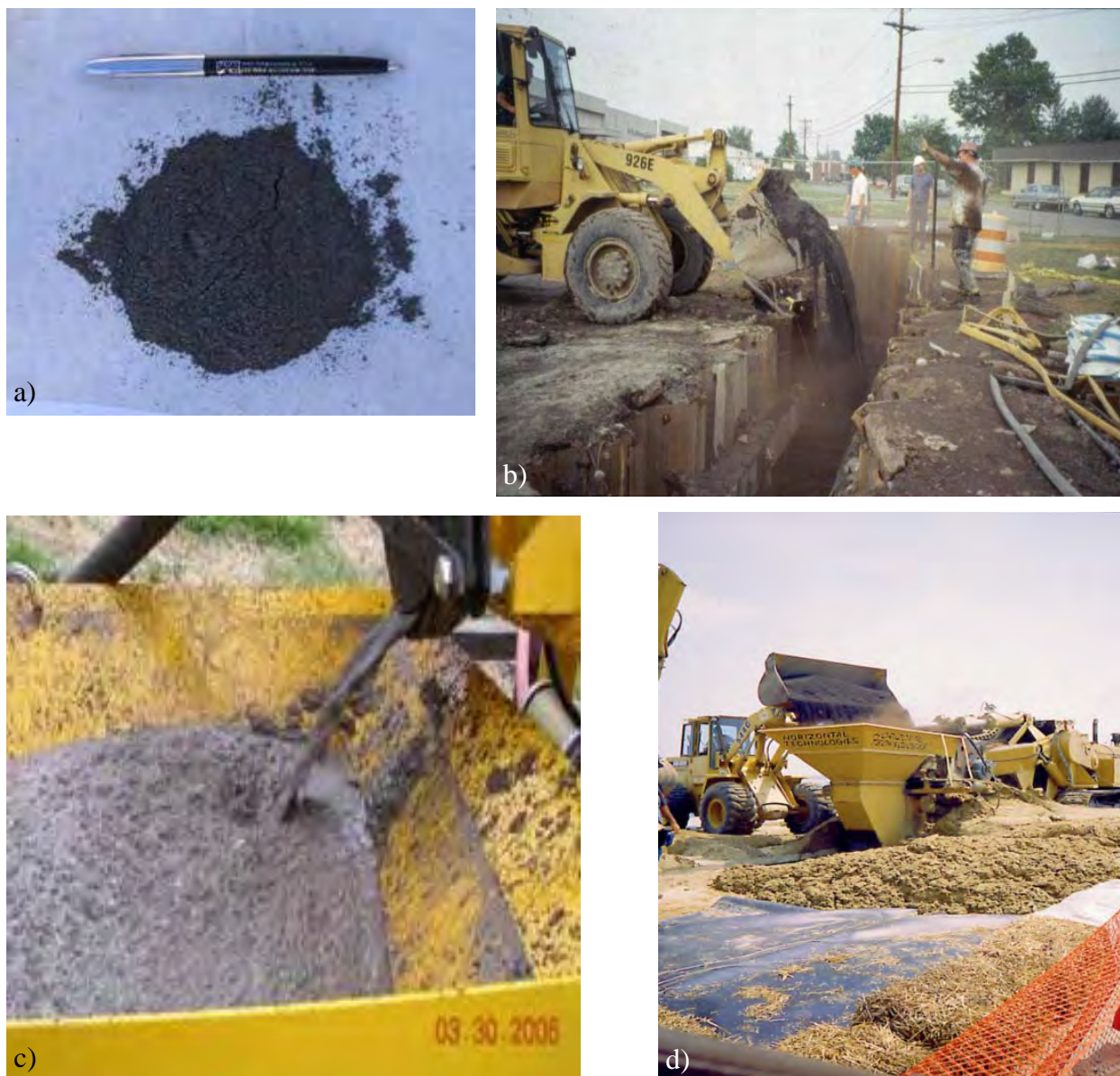
Figure 4-1. Examples of ZVI and ZVI emplacement: (a) fine-grained ZVI, (b) coarse-grained ZVI being placed in a trenched PRB, (c) microscale ZVI in an injectable EHC ® slurry, and (d) installation of ZVI PRB at a U.S. Coast Guard facility using a one-pass trencher.
