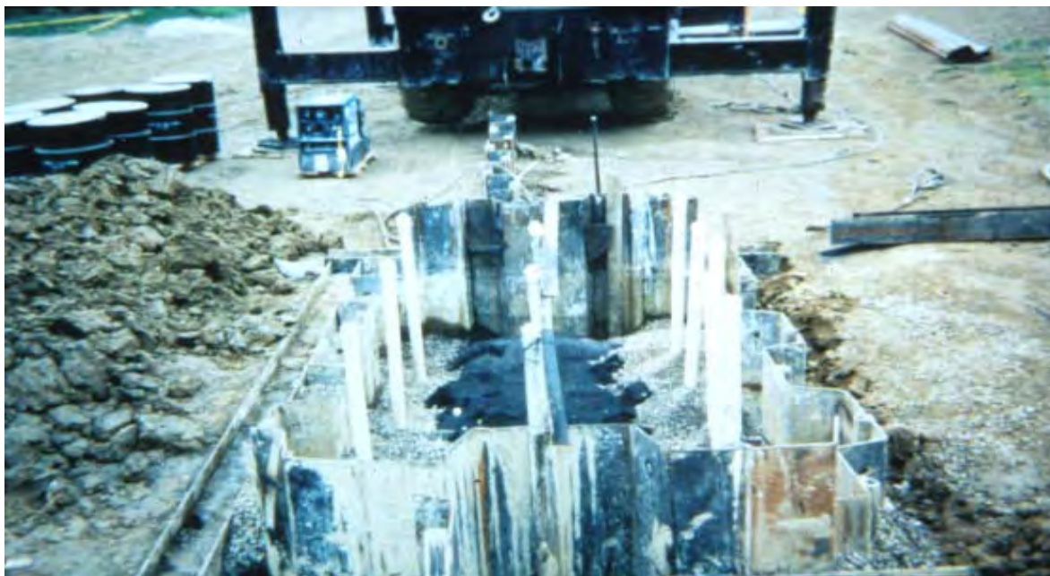
Figure 7-2. Photo of a pilot-scale monitoring system, New York (prior to sheet pile removal to create a flow-through gate section).
