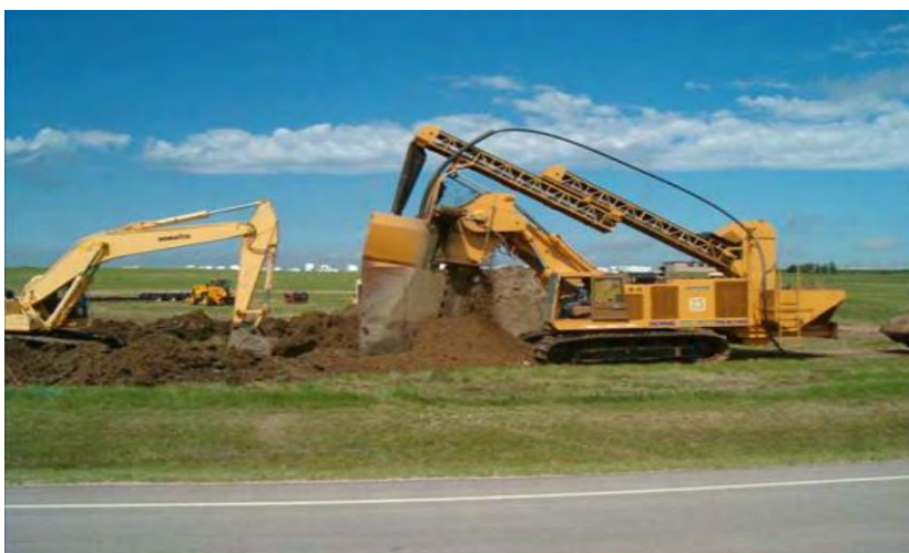
Figure 6-3. Continuous chain trencher at Ellsworth AFB, South Dakota. (Courtesy of the U.S. Air Force)
