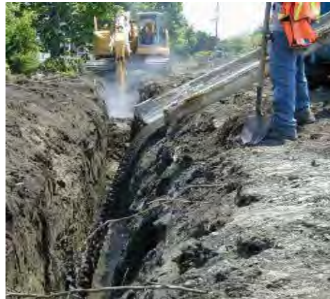
Figure 6-10. PRB installation in an unsupported excavation.
