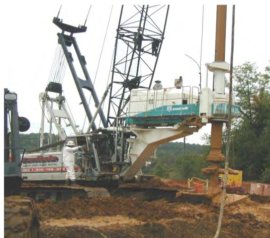
Figure 6-7. ZVI-clay application using soil mixing. (Courtesy of the U.S. Air Force)
