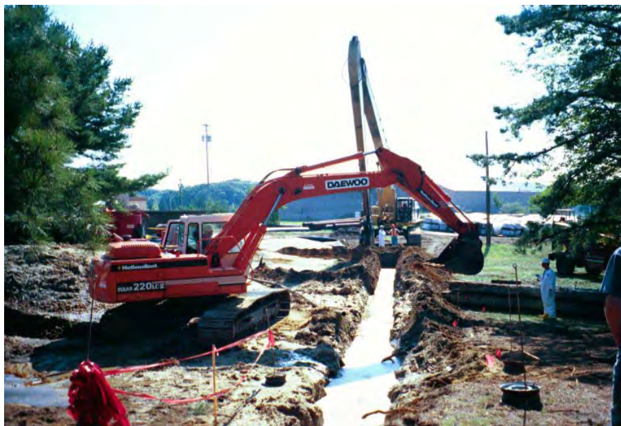
Figure 5-3. Guar slurry used during biopolymer PRB construction.
