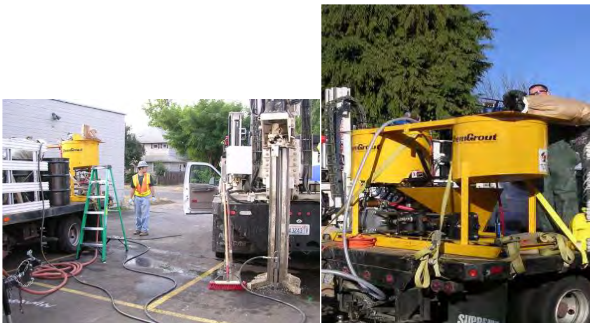
Figure 4-7. EHC mixing and injection equipment.
