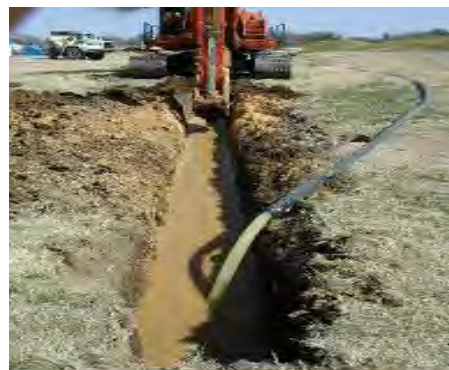
Figure 6-4. Biopolymer trench construction.
