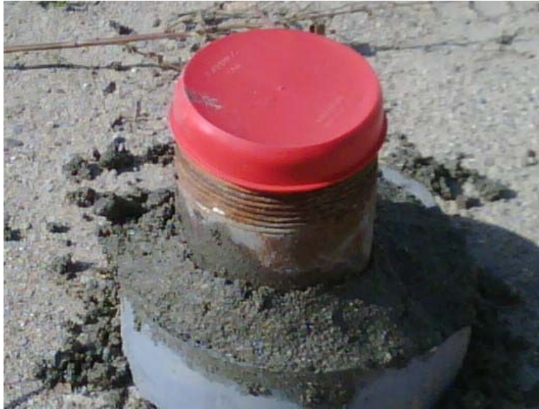
Caps and grout on electrode pipe taken March 10, 2010
