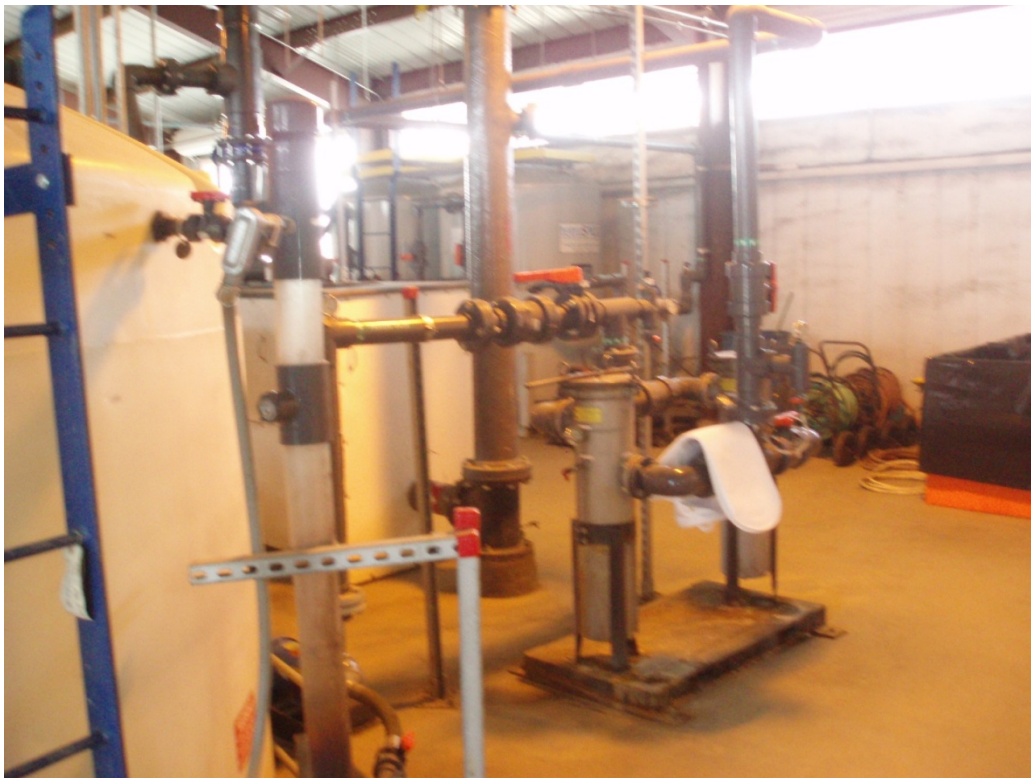
Photo 4: SP-204 and clean filter bag ready to be inserted into filter bag housing. May 27, 2010.
