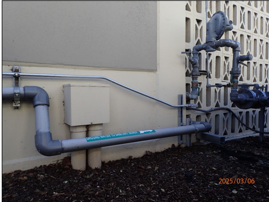
Photograph 1. March 6, 2025 at 2:35 PM Conveyance line to sanitary sewer. Facing south.
