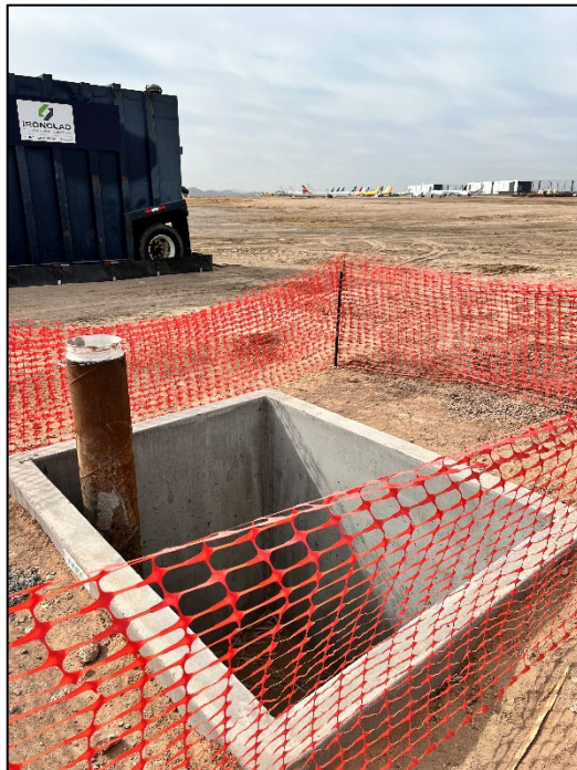
Photograph 8. February 13, 2025, 10:57 AM PGA South extraction well E-104 under construction. Facing south.
