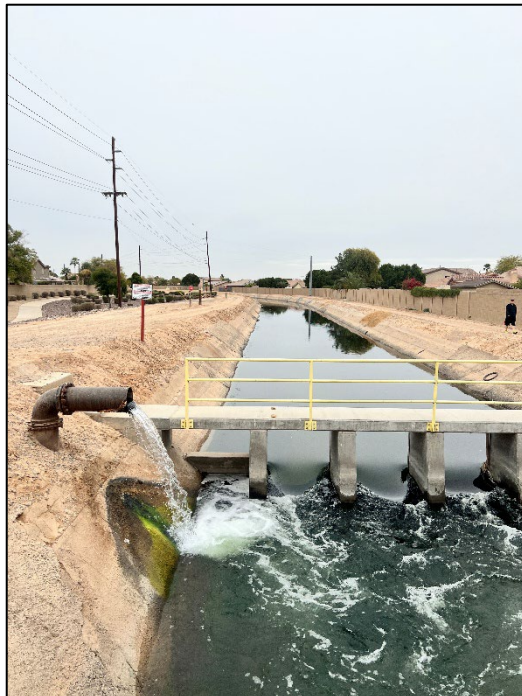
Photograph 22. February 13, 2025, 02:53 PGA North Treated groundwater discharge into the Roosevelt Canal. Facing east.
