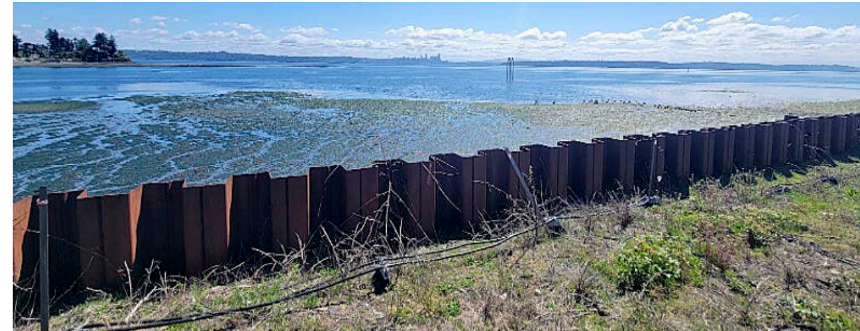
U.S. Army Corps of Engineers sheet pile wall at the Wyckoff/Eagle Harbor Superfund site
