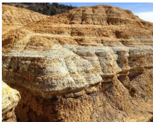
Photo 10: Heavily eroded tailings deposit in a depression at the smelter.
