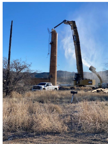
Photo 4: ADEQ dismantling the smelter smoke stack, 2022.
