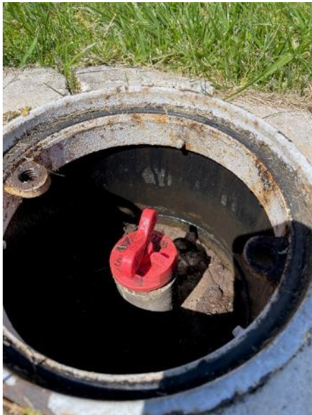
MW 165A with protective casing cover removed. The plug was not locked.
