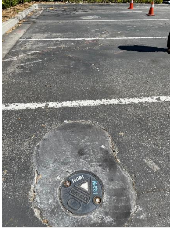
Monitoring Well (160B1) and grouted injection point in the background.
