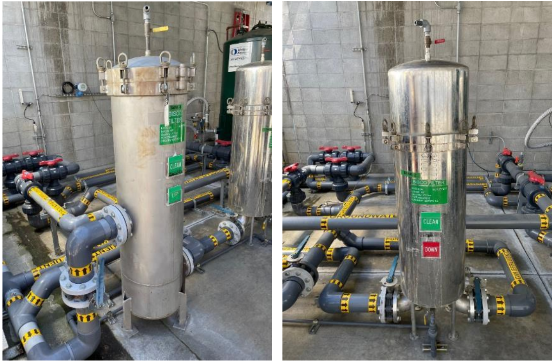
Cartridge filters. Capable of running series, or one at a time.
