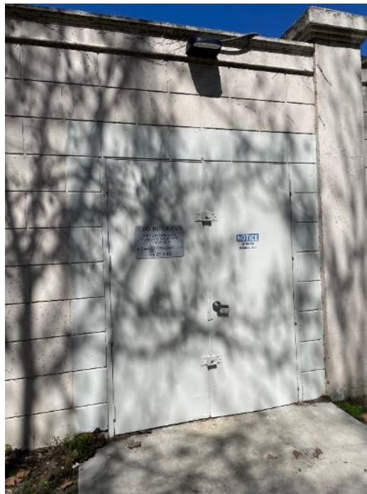
Locked door and outer wall of the Lakeside GWETS.
