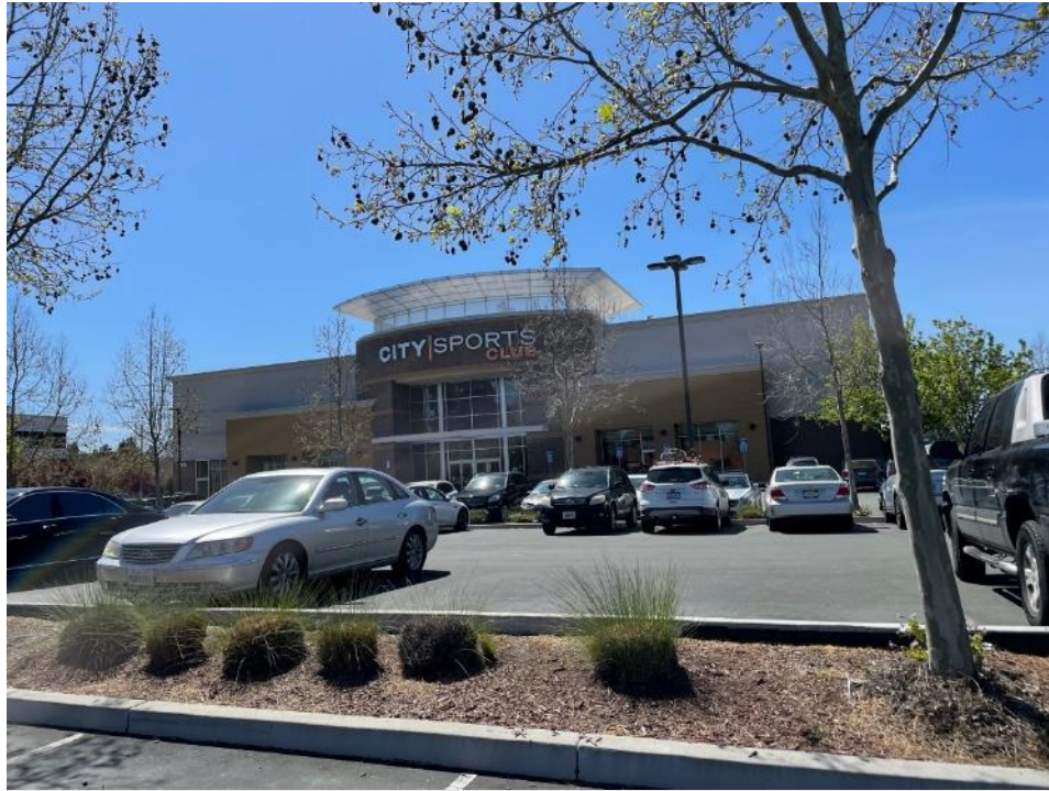
1165 East Arques Ave. Photo taken facing west.
