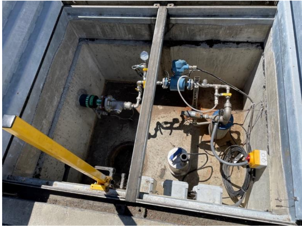
Extraction well EWA-1 located adjacent to the OU1 Subunit 1 GWETS.
