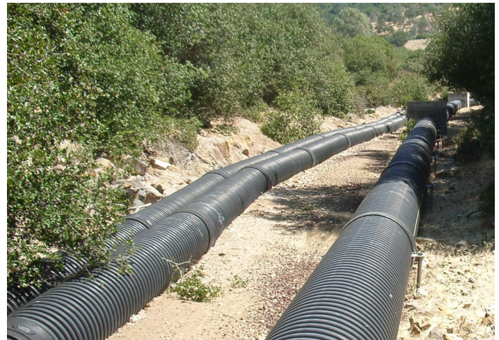
(Left) Face of Waste Rock Dam during installation of stormwater control features and (Right) Stormwater Diversion Pipeline.
