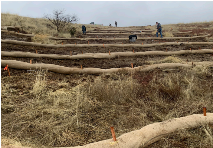
(Left) Face of Waste Rock Dam during installation of stormwater control features and (Right) Stormwater Diversion Pipeline.
