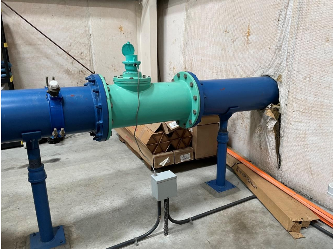
Figure 38 – Flow Totalizer leaving UV system
