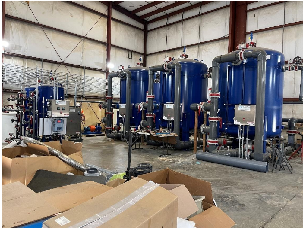
Figure 31 – New Nitrate treatment system by Evoqua (in the process of installation)
