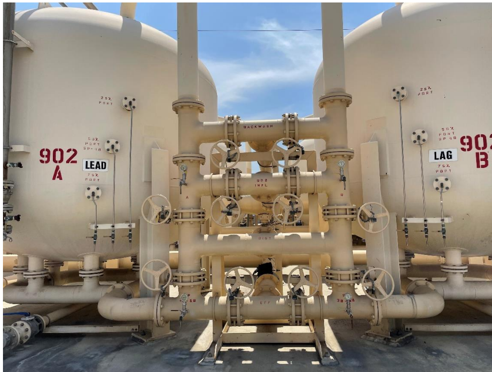
Figure 20 – Lead and Lag LGAC vessels
