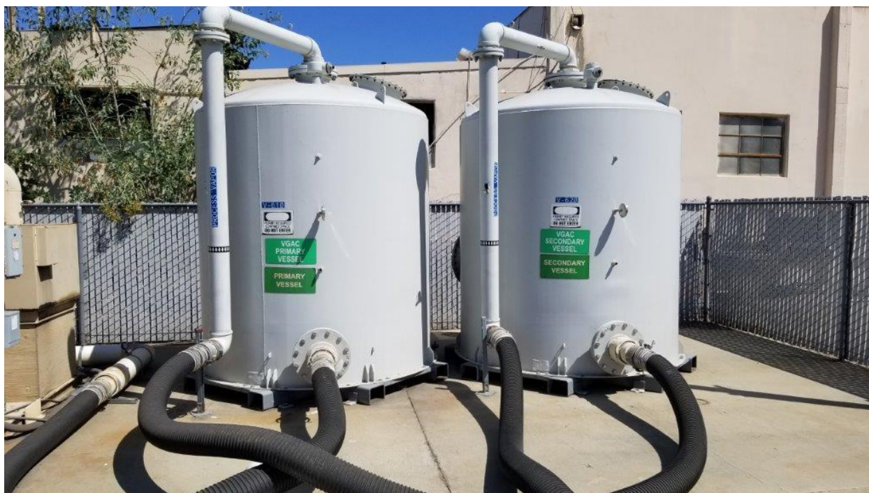
Figure 29. SVE system VGAC vessels facing NE.
