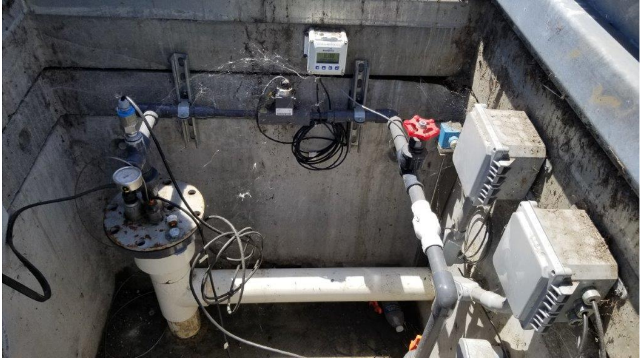
Figure 35. Dual Phase Extraction Well Vault DPE 10D.
