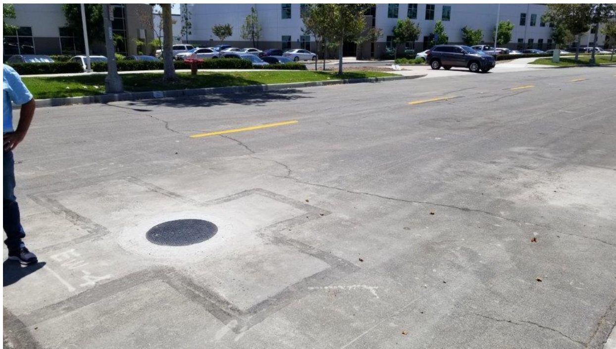
Figure 37. Extraction Well EW-4 located on Hawkins St. facing SW.
