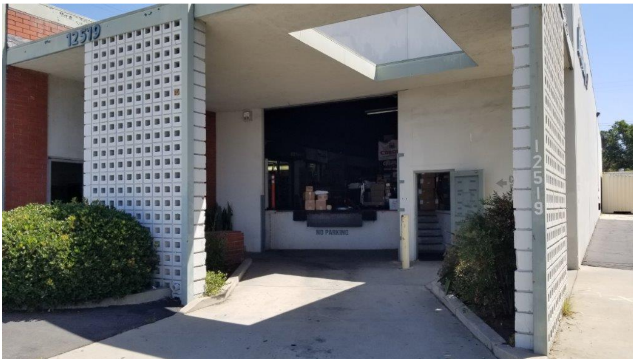
Figure 31. Bishop Company property facing SE.
