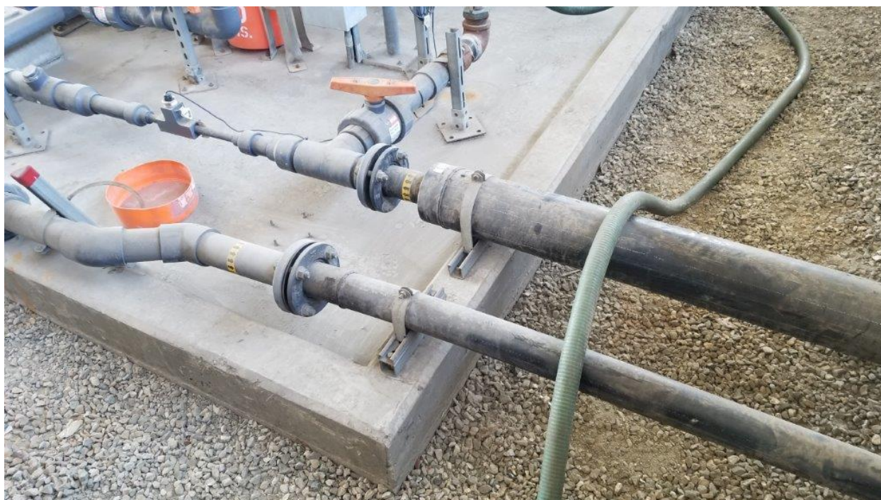
Figure 12. HDPE lines in.
