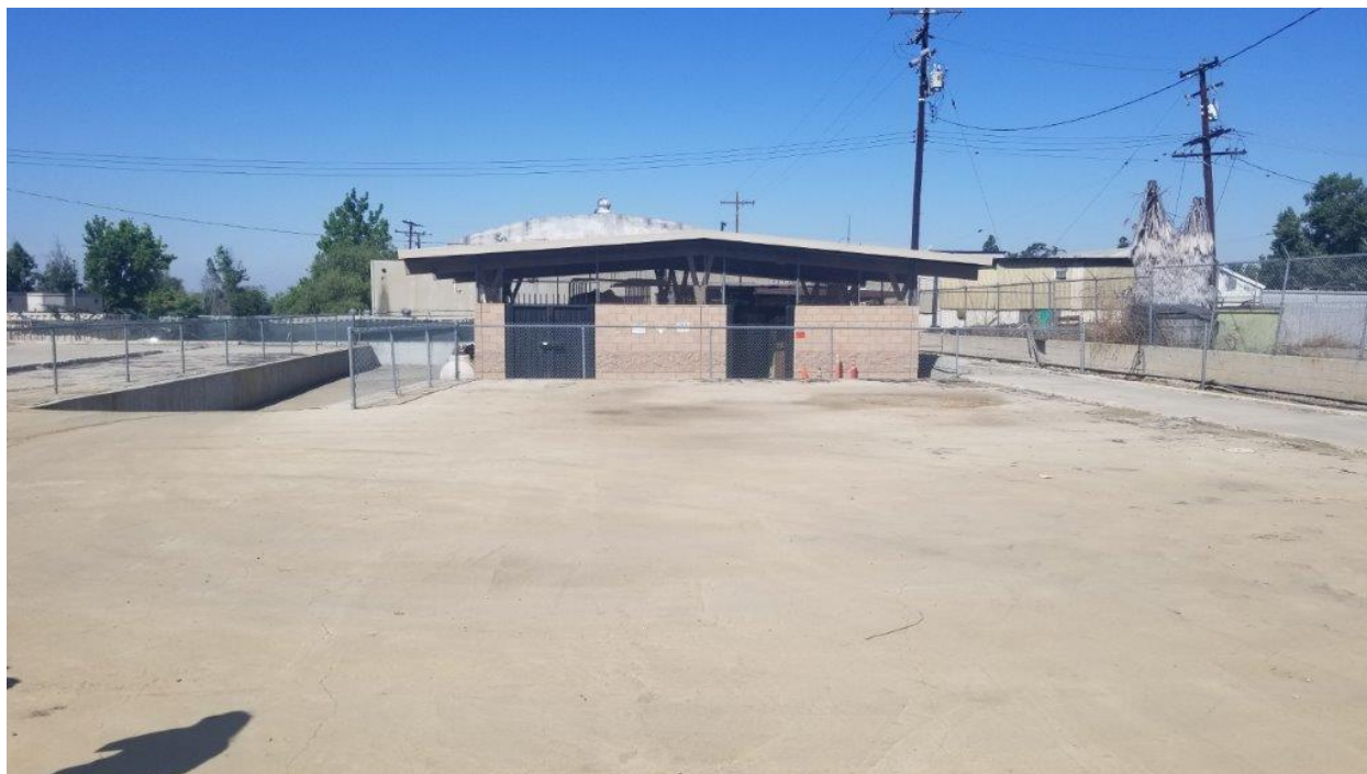
Figure 11. Overview of Groundwater Treatment Plant (GWTP) Compound facing NW.
