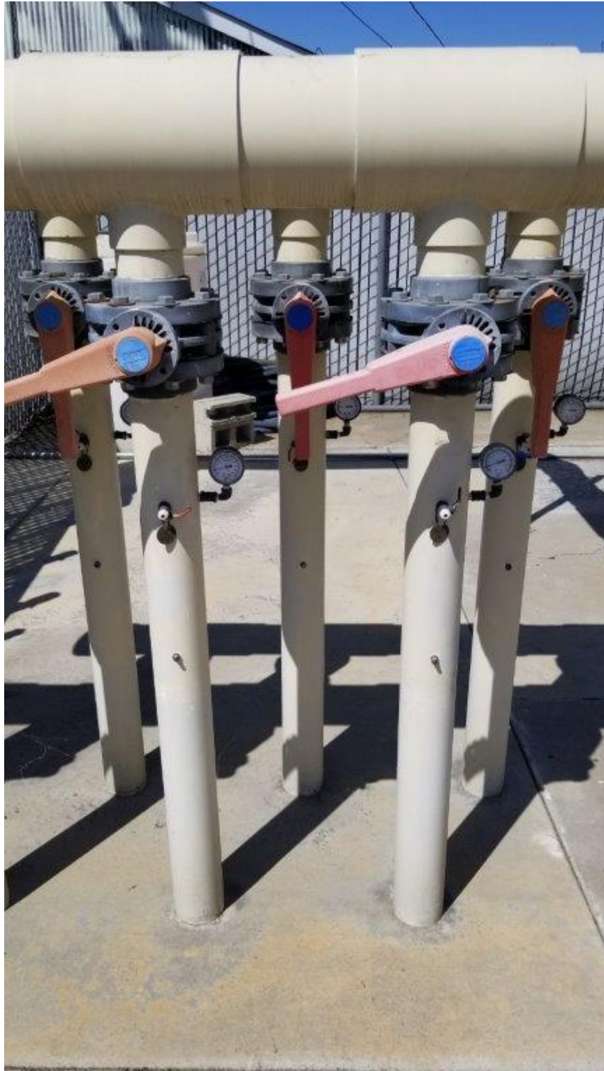
Figure 28. SVE sampling ports VE-14D and DPE-4.
