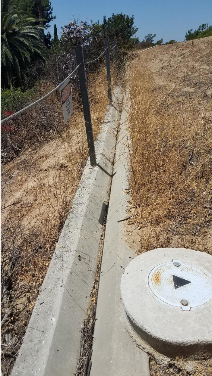
Drainage ditch on perimeter of Ramparts sumps
