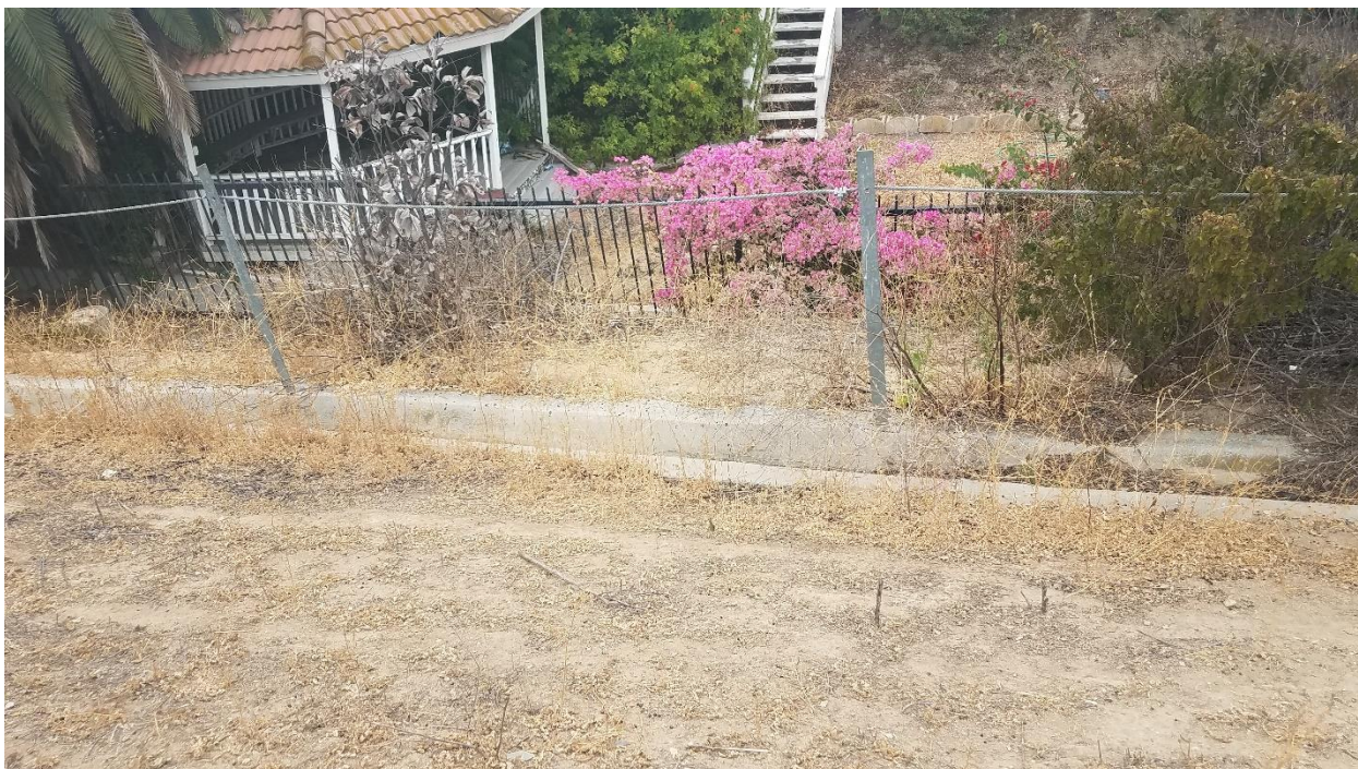
Drainage ditch on perimeter of Ramparts sumps
