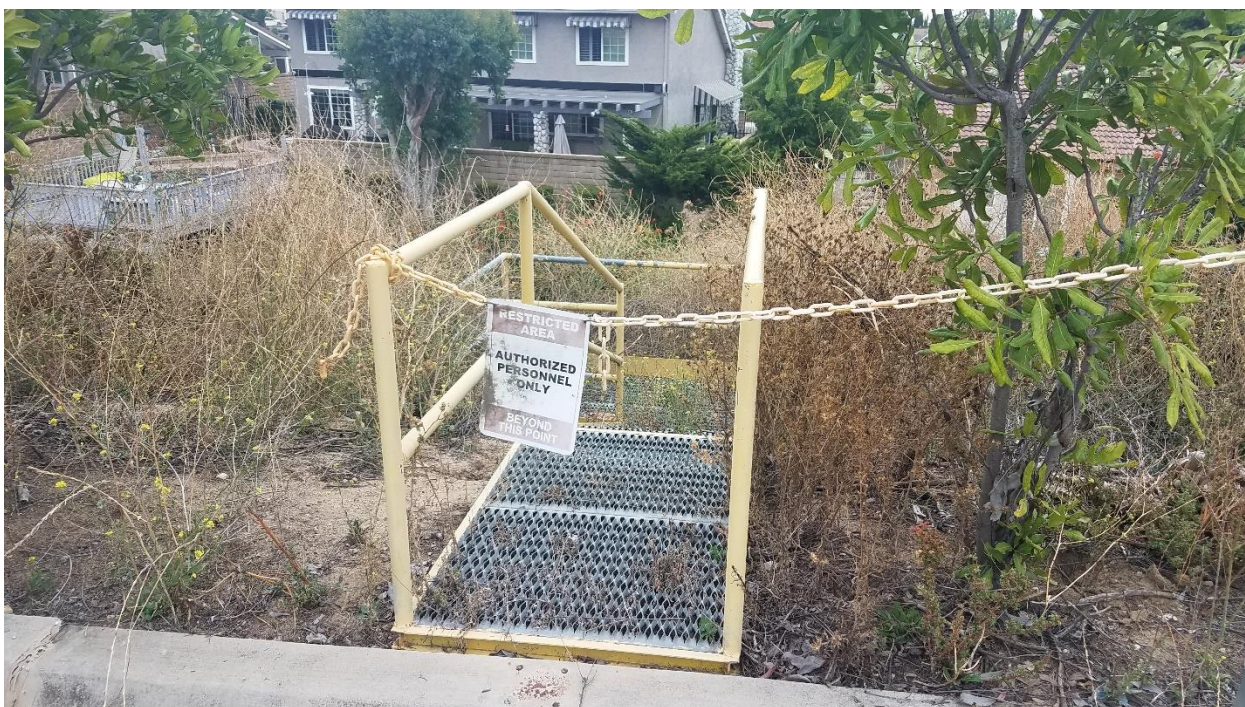
Sampling platform in Ramparts Sump area.
