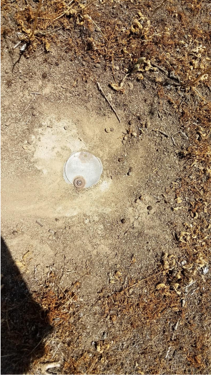
Settlement monument in Ramparts sump area
