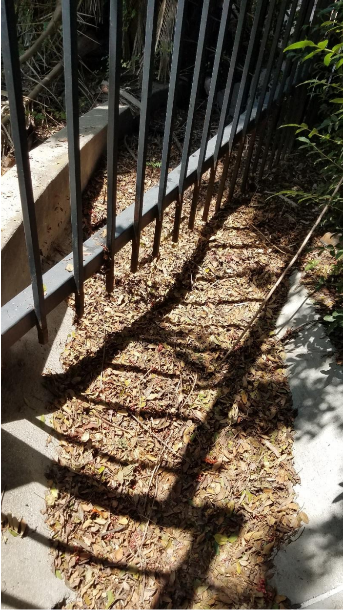
Drainage ditch on perimeter of Ramparts sumps
