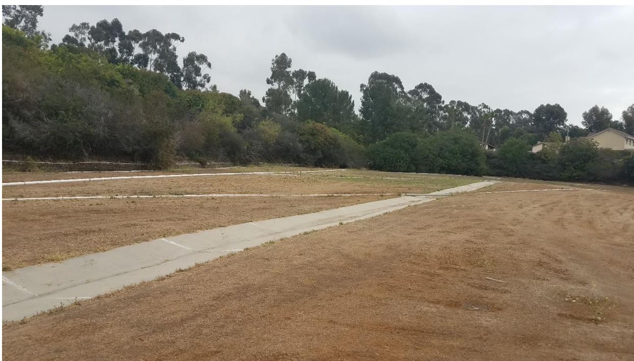
Surface drainage system for Ramparts sumps, with landscaping sprinkler system
