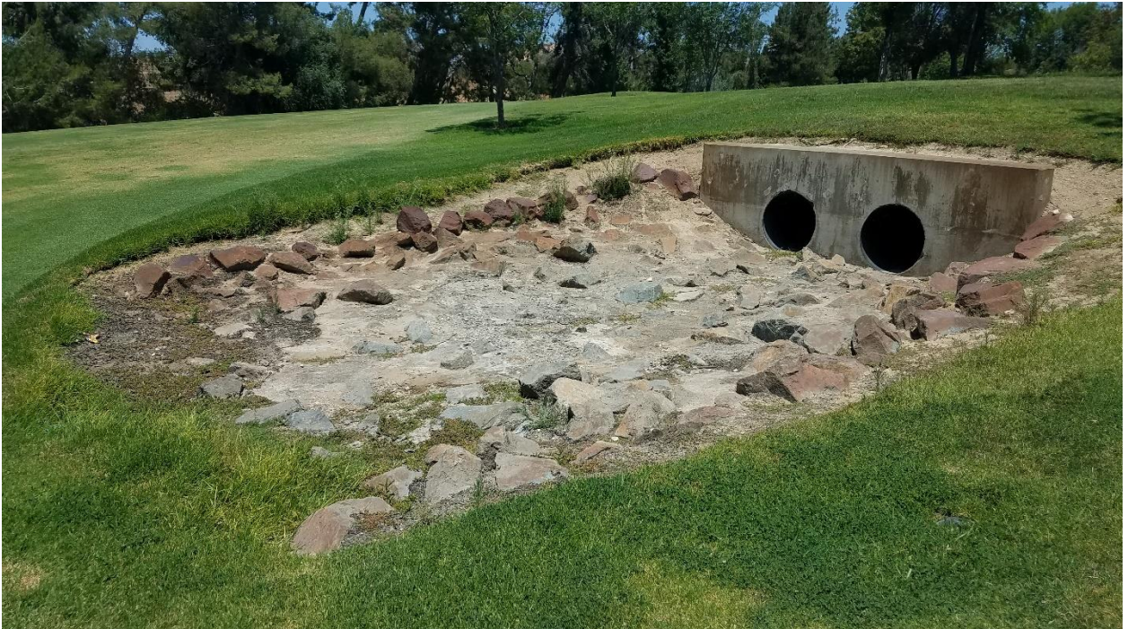
Riprap outlet also appeared to be functioning as designed
