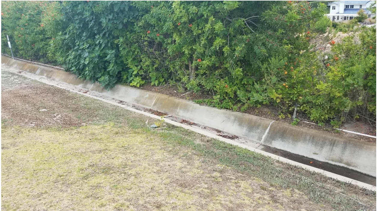
Drainage ditch surrounding perimeter of site
