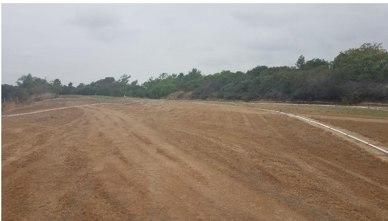
Another view of the Ramparts sumps and cap with dry vegetative cover
