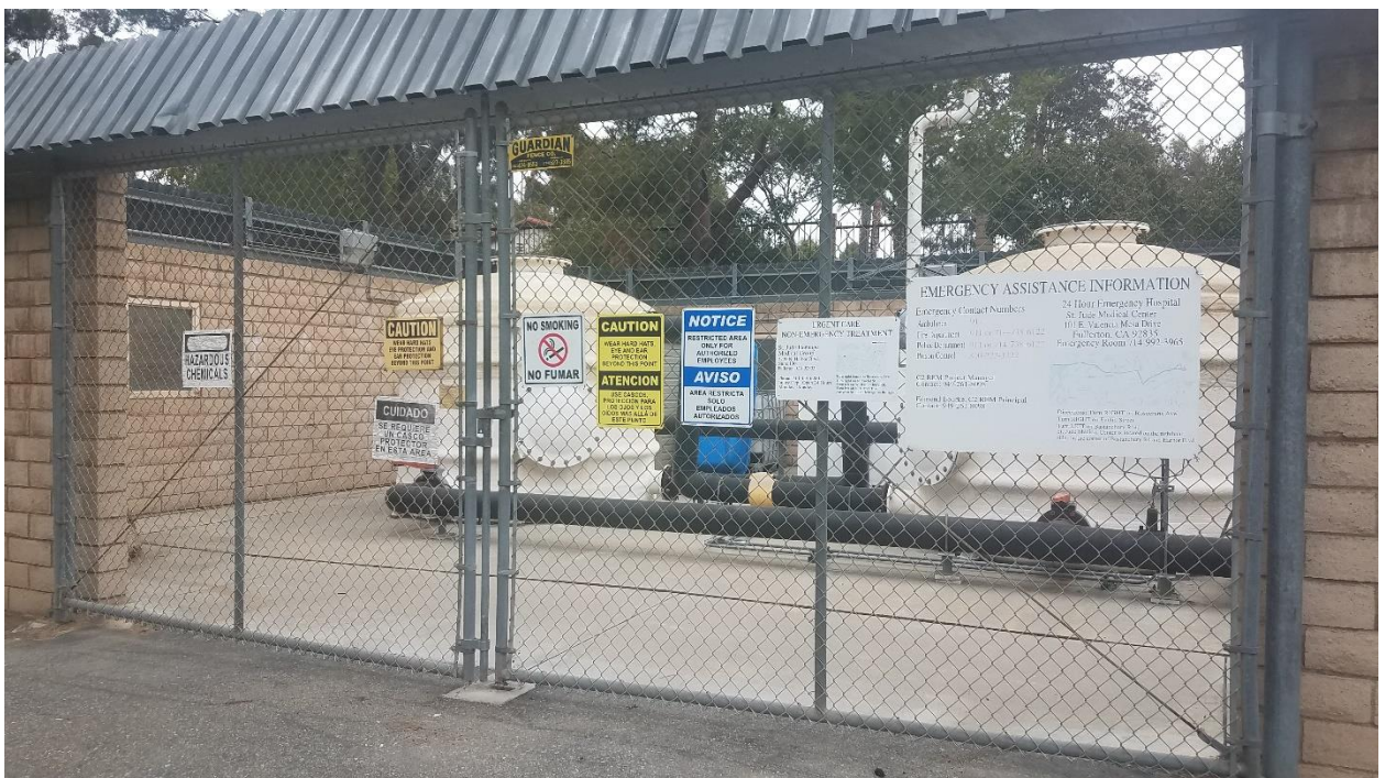
Remediation enclosure securely maintained with signage displayed on the outside fencing
