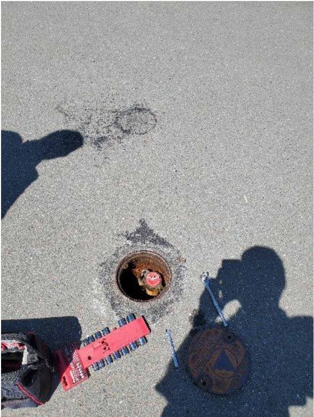
Photo 13 – MW-36A, watertight well cap locked, cover was bolted.
