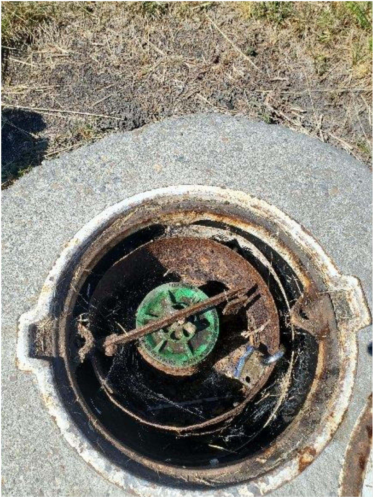
Photo 10 –MW-19A closeup with watertight cap.
