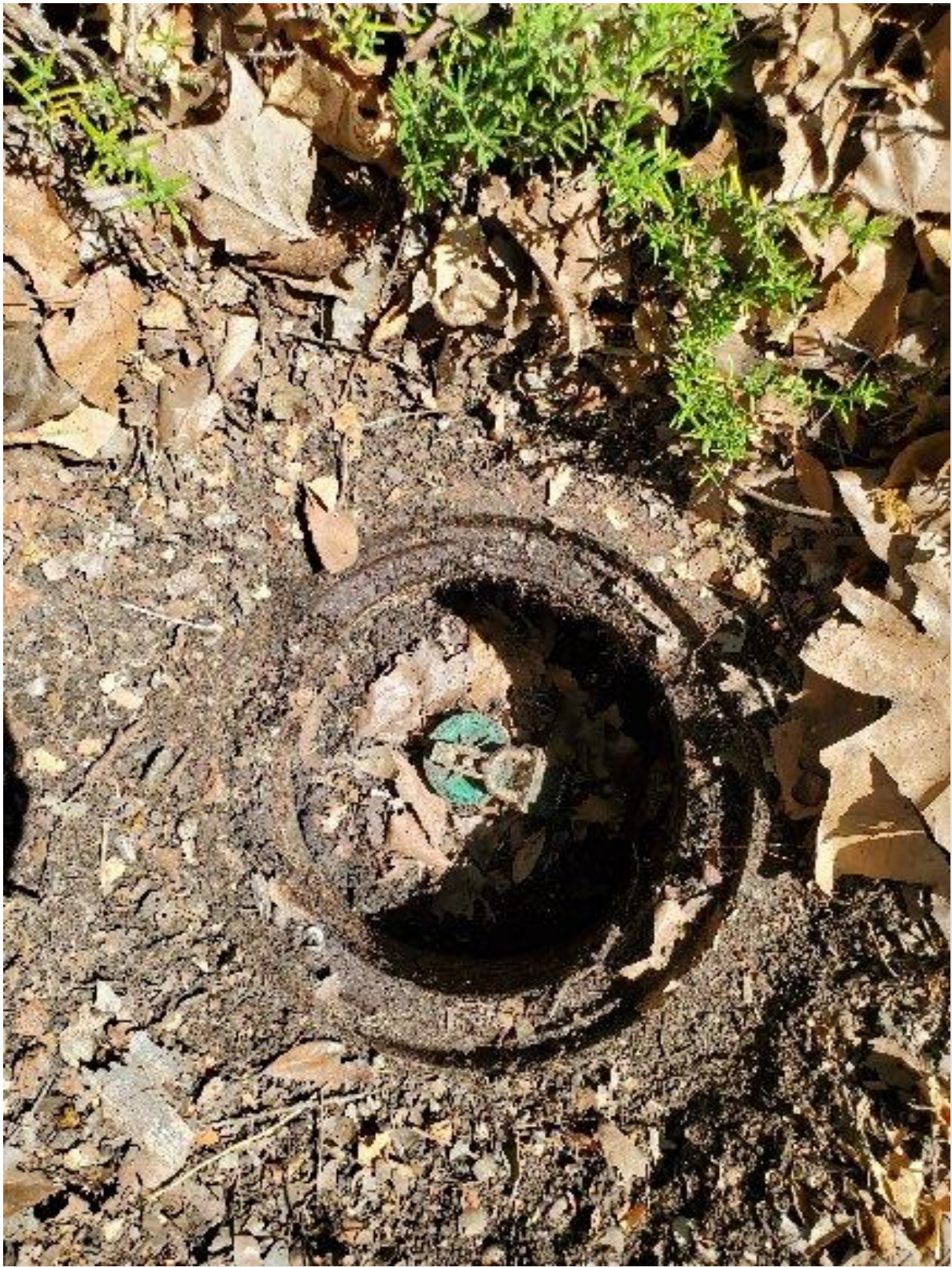
Photo 14 – MW-35A, watertight well cap locked, cover was unbolting.
