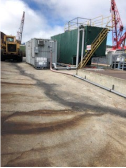
Photo 12. Treatment plant (looking south)
