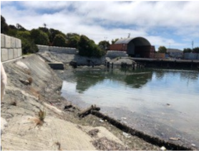
Photo 19. Outfall at SW-7 and shotcrete on shoreline (looking east)
