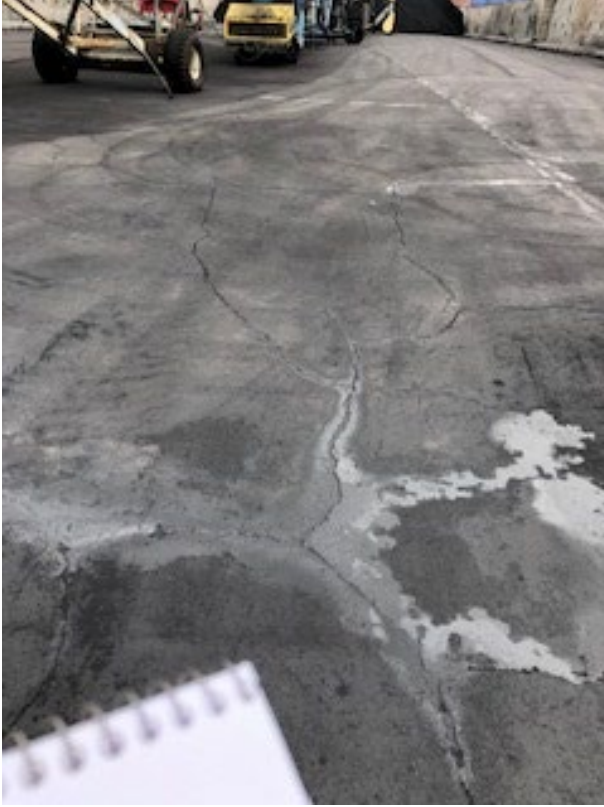
Photo 5. Cracking
