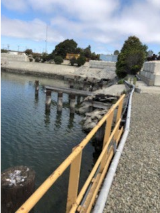
Photo 16. Shotcrete along shore near outfall
