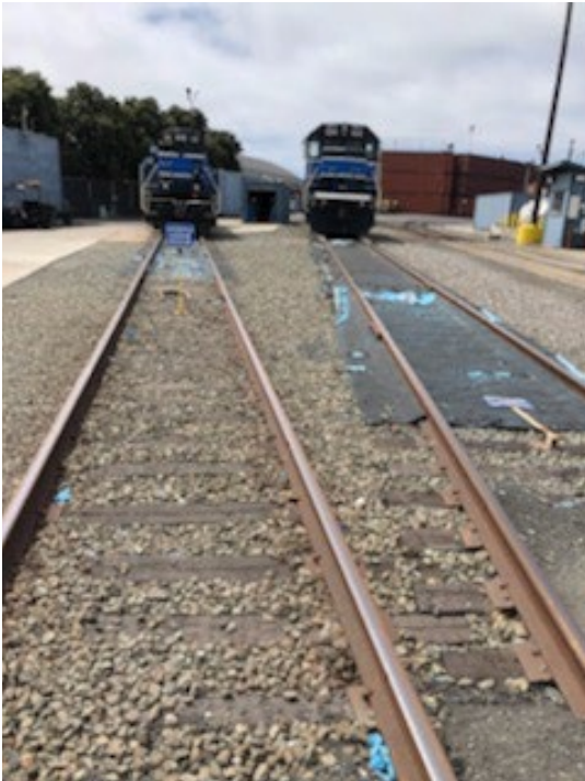
Photo 15. Railroad tracks (facing south)
