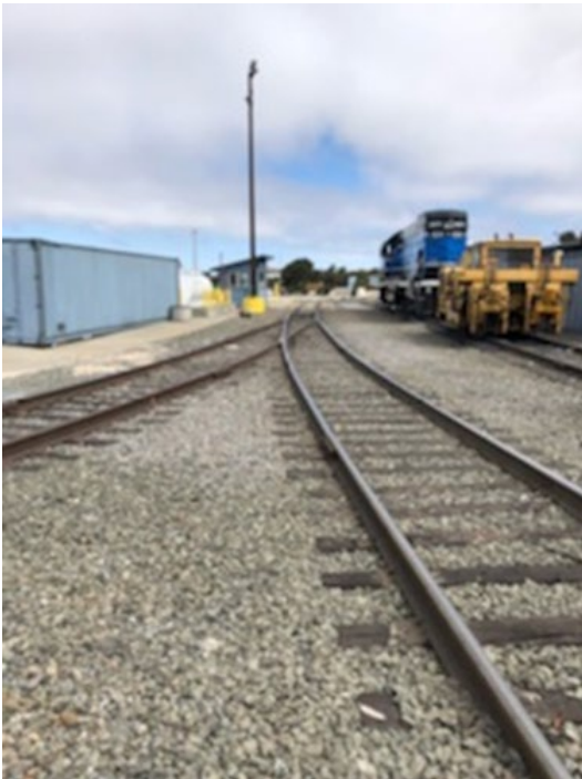
Photo 13. Gravel cover under railroad tracks
