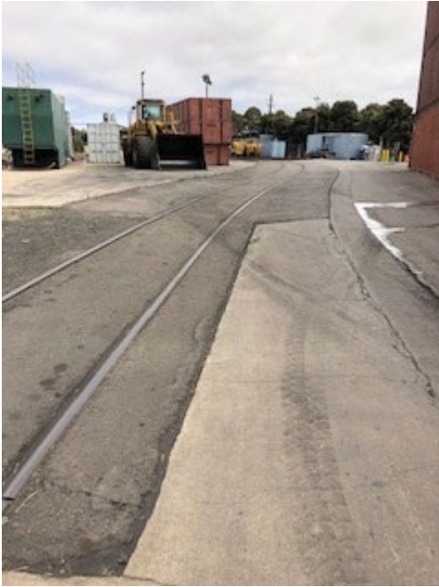
Photo 11. Connection between railroad pavement and asphalt (looking north past SW-4)
