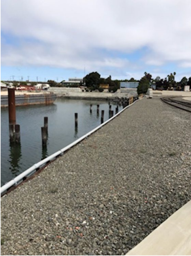
Photo 14. City Outfall and shotcrete along shore (looking north)
